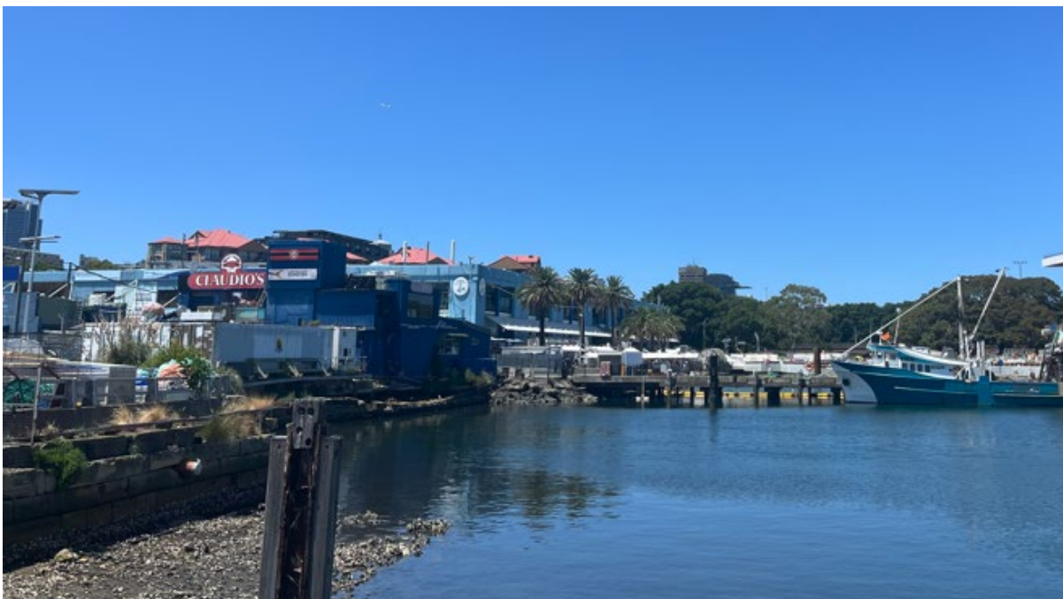
Figure 7 View of Blackwattle Bay and foreshore western edge of site (looking south)
