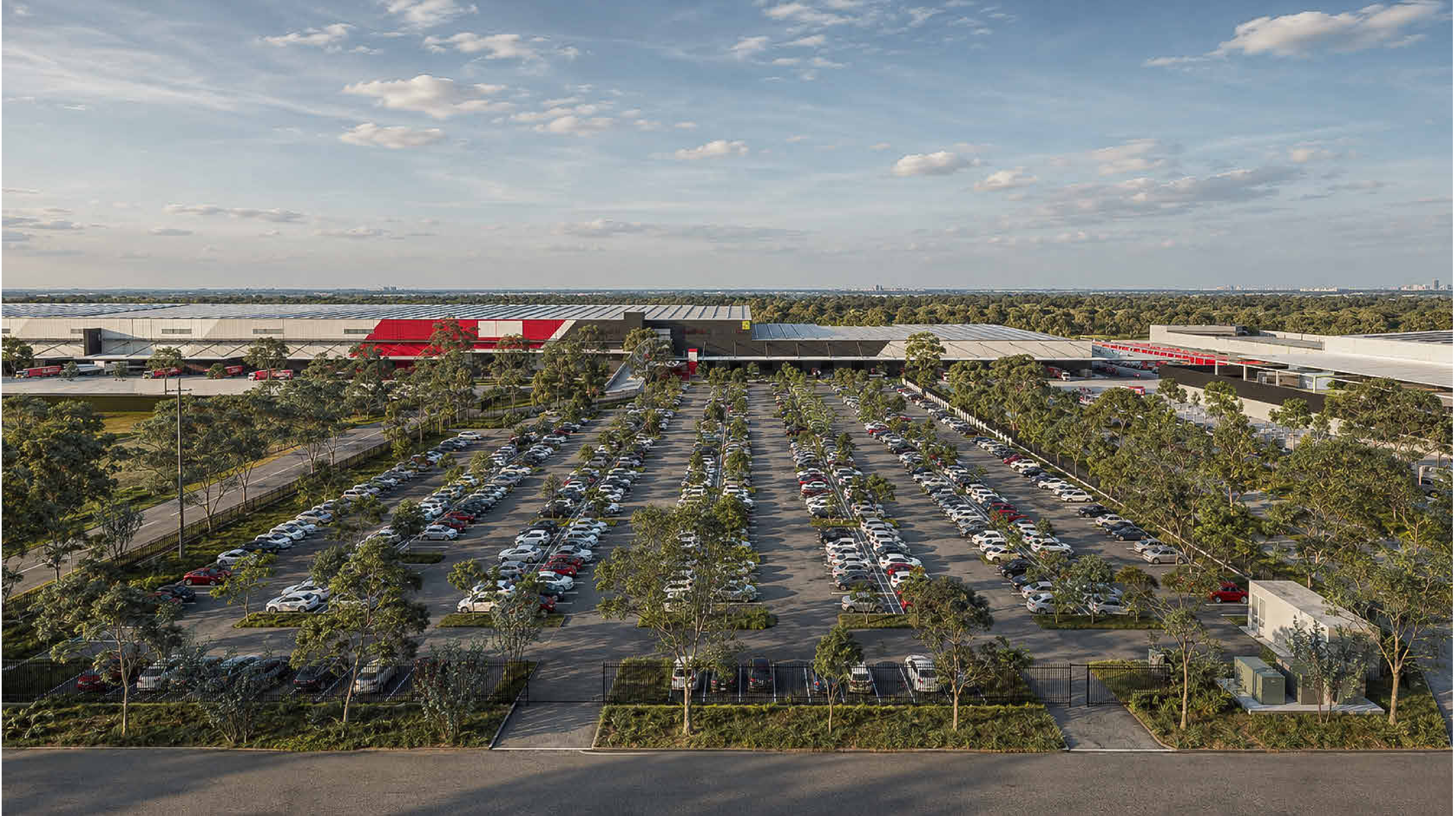
VIEW OF CARPARK FROM LATITUDE ROAD
