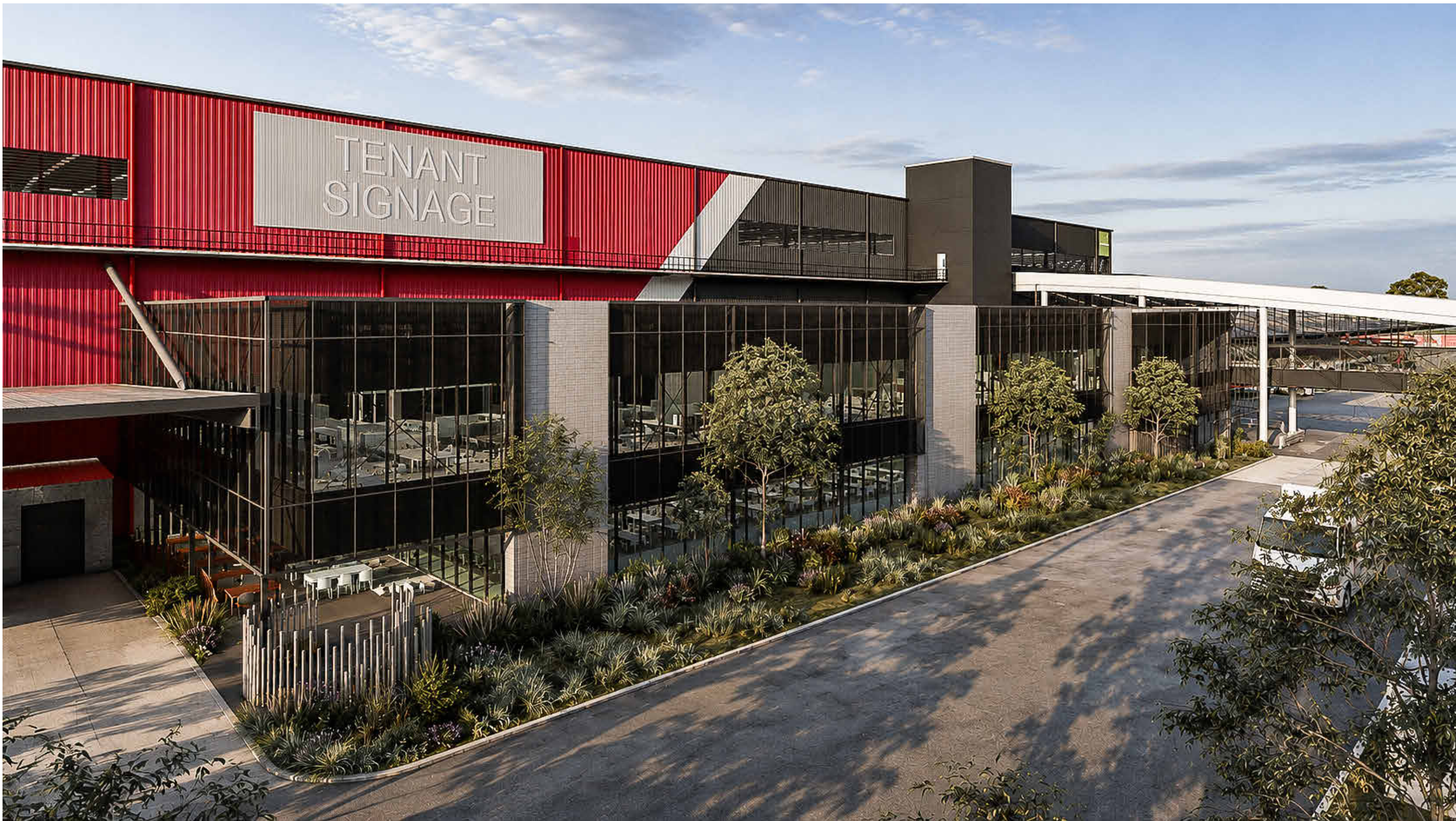
VIEW OF OFFICE FACADE FROM CARPARK
