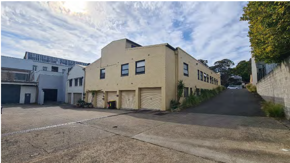
Figure 17 North-east facing view of the concrete paved carpark showing the gradual rise up to Francis Street.
