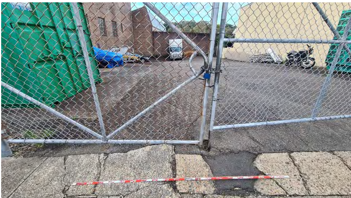
Figure 15 East facing view of the entrance to the asphalted carpark to the south of Cyclops warehouse building along North Street.
