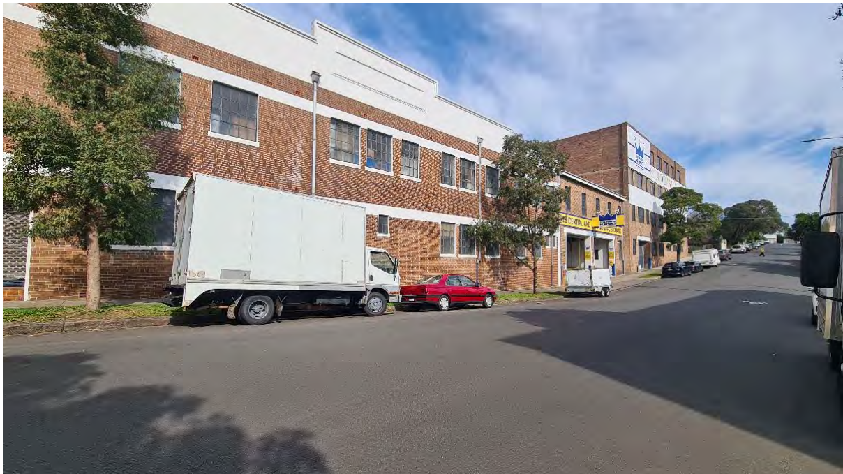
Figure 11 South-west facing view of the warehouse buildings along William Street.
