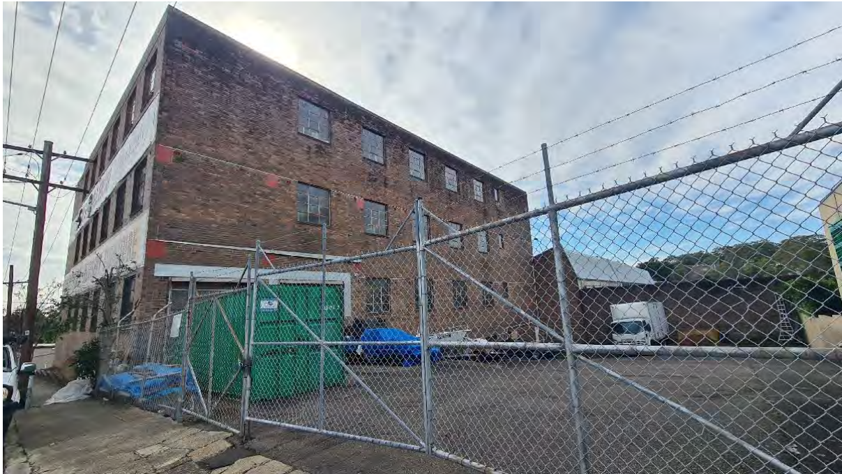
Figure 14 North-east facing view of the asphalted carpark area to the south of the building along North Street.
