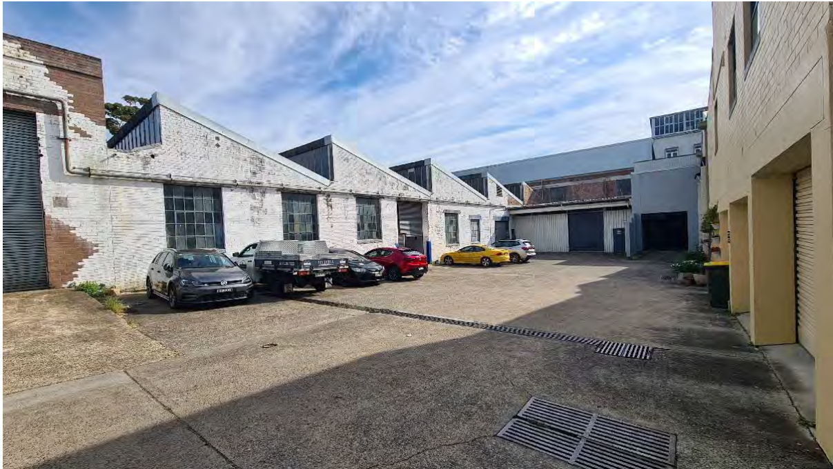
Figure 12 North-west facing view of the concrete paved carpark to the rear of the warehouses, showing the service pits and gutters.
