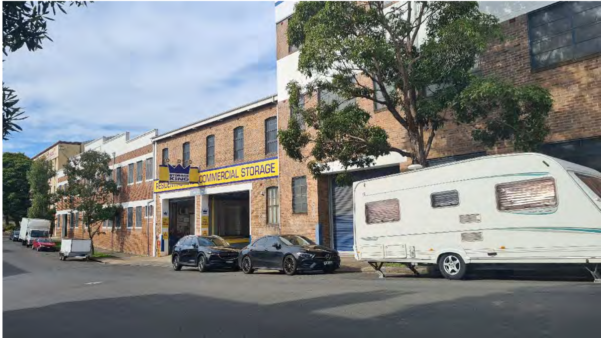
Figure 10 South-east facing view of the warehouse buildings along William Street.
