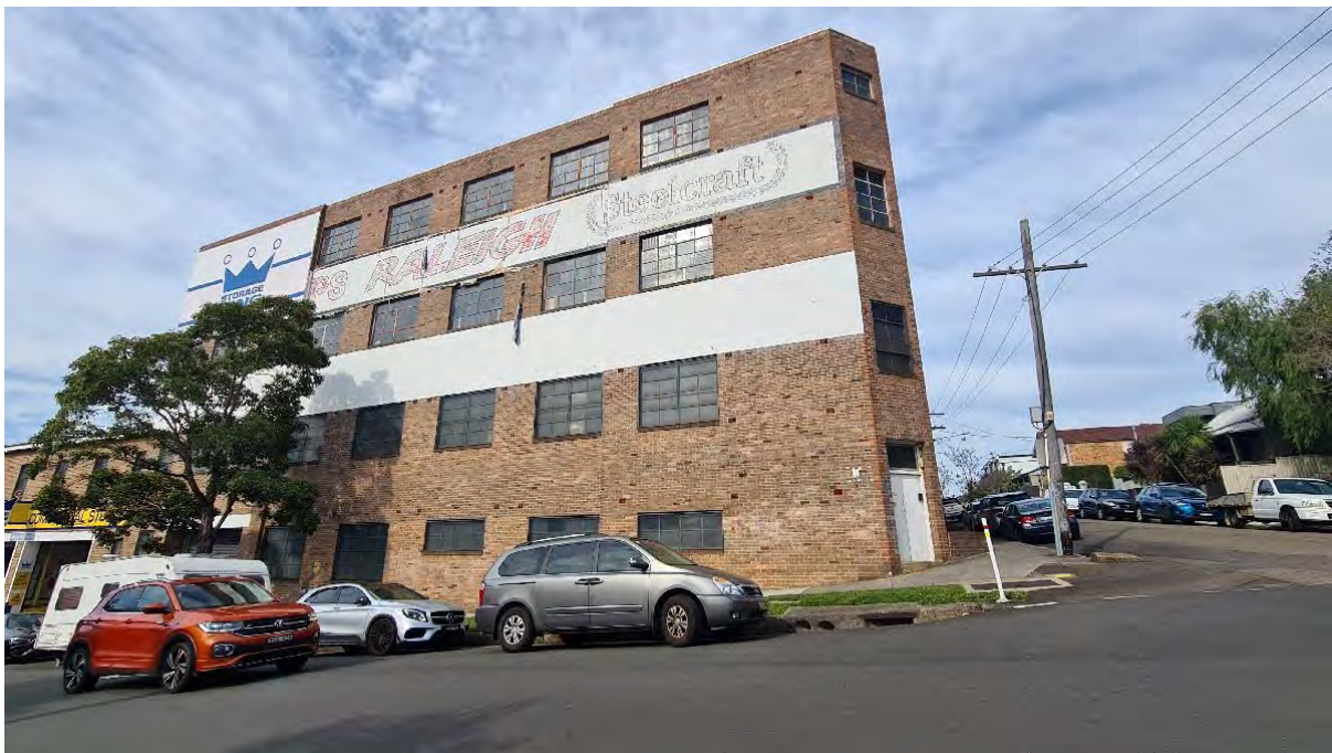
Figure 13 South-east facing view of the northern elevation of the north-western warehouse.
