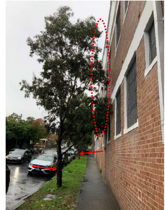
6: Trees G9 – branches to be pushed back for scaffolding installation. Minor pruning (where required) to be supervised and guided by the Project Arborist
