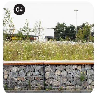
Reuse of site material in walls and seating
