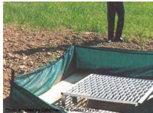
Figure 22 - Fabric drop inlet protection
