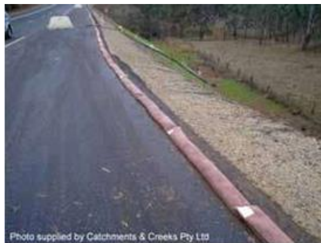
Figure 3 -Flow Control Berm
