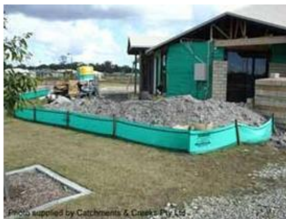
Figure 18 - Sediment fence stockpile control
