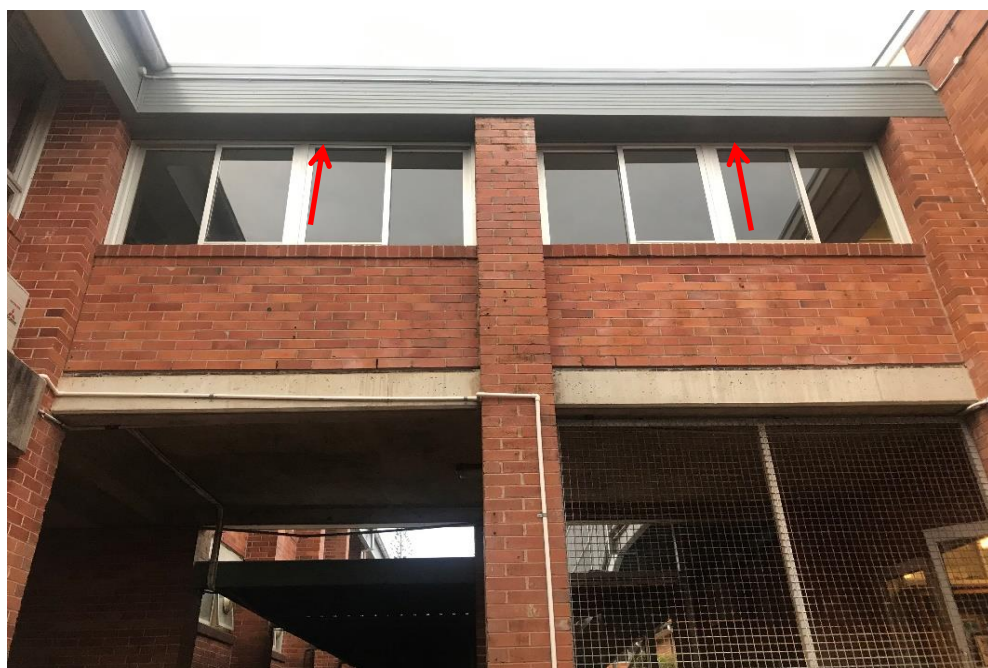
Photograph 2: B00B, BR0020 / BR1023, eaves, assumed fibre cement sheeting, asbestos (assumed).
