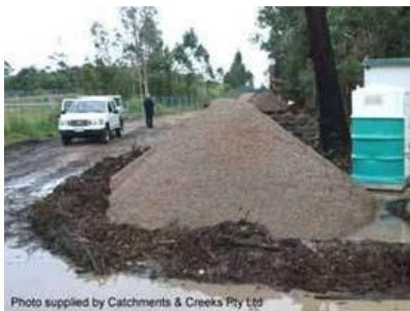
Figure 17 - Mulch berm stockpile control
