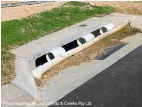
Figure 19 - Kerb Inlet sediment trap
