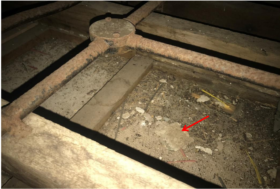
Photograph 17: B00B, BR1021, top of ceiling, minor fibre cement sheeting debris, asbestos (assumed).
