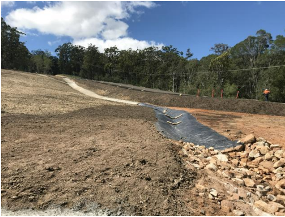
Figure 1 – Plastic-lined catch drain
