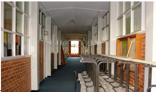
The first floor corridor displays the original materials of the building in good condition, with acoustic ceiling treatment, exposed brick walls and timber framed windows and doors.
