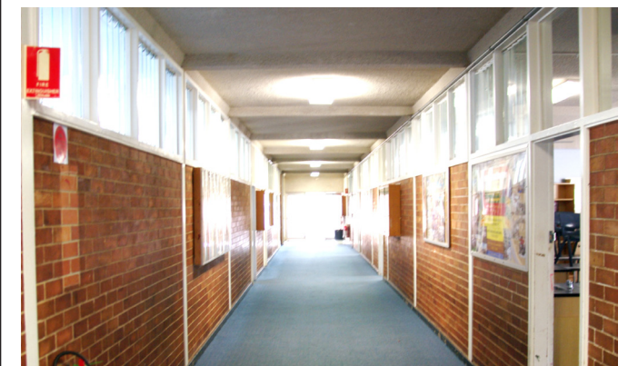
Ground floor corridor showing vermiculite ceiling, face brick walls, timber door and window frames and vertical glass louvres.
