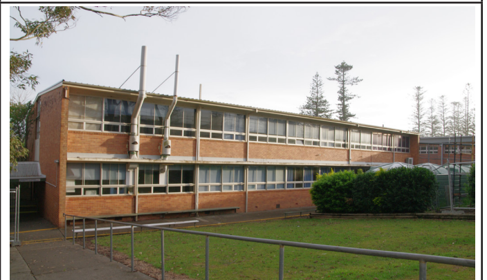
Intrusive additions of ventilation equipment are apparent on the southern elevation. The building is partially obscured by plantings and water tanks at the rear of B00U. Relocation of these later elements would enhance the presentation of the building from the main entrance to the school.
