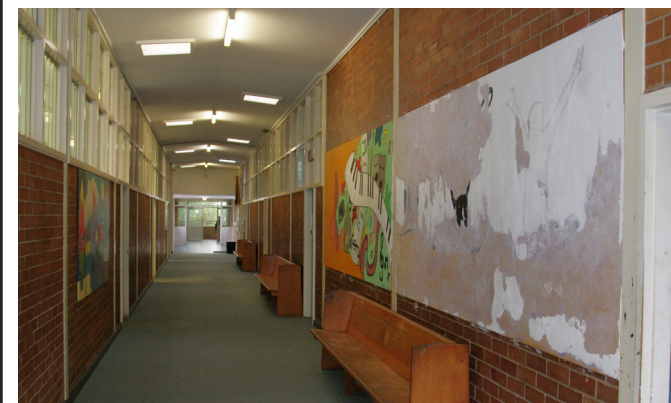
First floor corridor, with original skylights, and double-height windows. Note there are no windows to the corridor for the Music Room (right) to improve acoustic performance.
