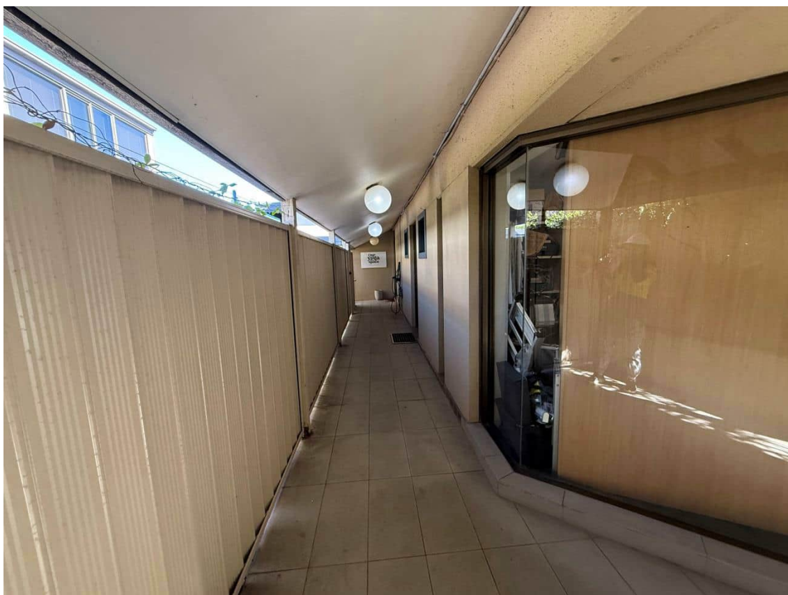
Photograph 11: Gap between front and rear structures, 52 Ourimbah Road (15 April 2026).
