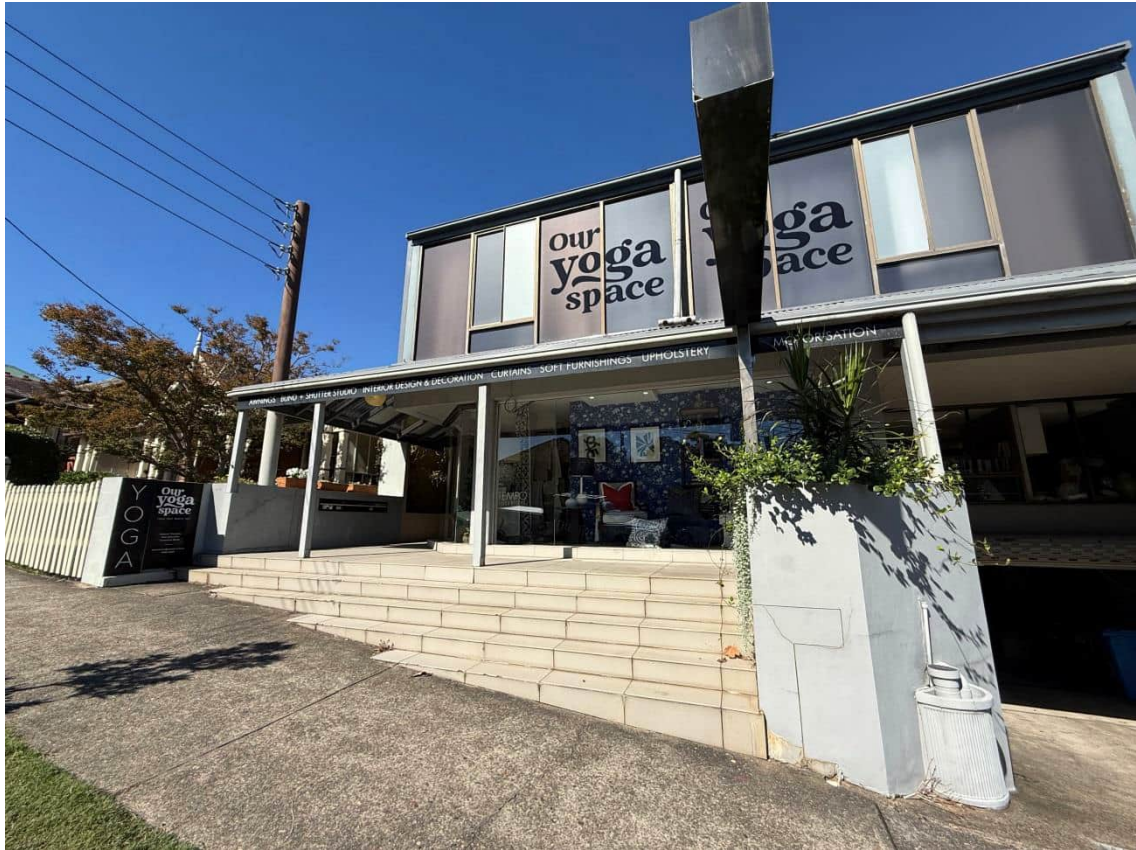
Photograph 9: 52 Ourimbah Road (15 April 2026).
