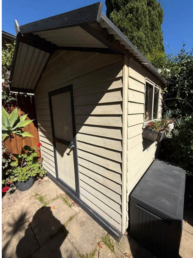
Photograph 13: Timber shed located at 56 Ourimbah Road (15 April 2026).
