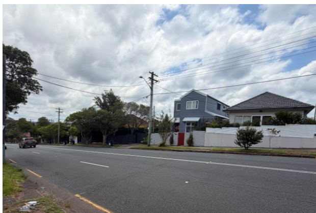
Figure 2 Image of 81A and 83 Ourimbah Road, looking north-west. Source: Gyde
