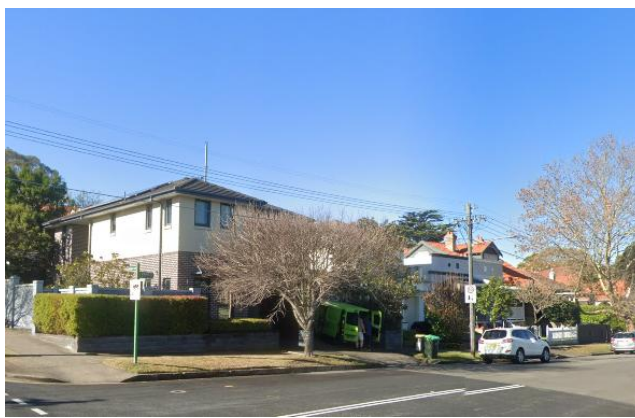
Figure 3 Image of 37 and 37A Bond Street looking south-east. Source: Google Streetview 2024
