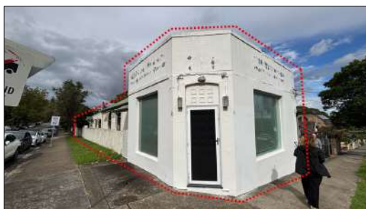
Figure 11: The shopfront and dwelling to the rear, outlined in red, on the corner of Ourimbah Road and Bond Street.
