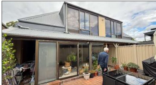
Figure 19: The principal elevation of the townhouse dwellings to the rear of No. 52 Ourimbah Road.
