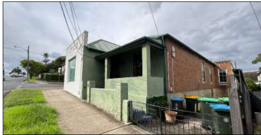
Figure 12: The principal and western elevations of No. 42 Ourimbah Road, Mosman.
