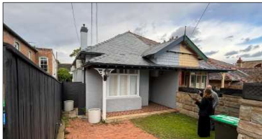
Figure 13: No. 44 Ourimbah Road, Mosman. The gable, chimney and tiled front verandah are in view.
