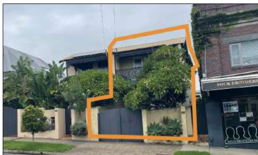
Figure 21: The principal elevation of No. 56 Ourimbah Street, Mosman (outlined in brown).
