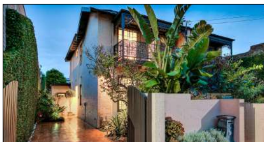
Figure 20: The principal and eastern elevations of No. 54 Ourimbah Road Mosman. Realestate.com.au, accessed 2026.
