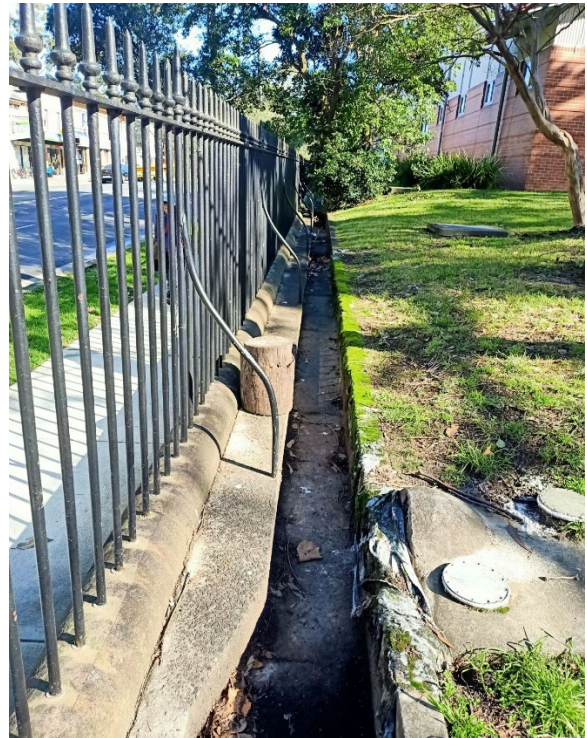
Figure 4.9: Concrete drainage channel constructed against the rear of the sandstone heritage wall along Bay Road. Source: Curio, 2021.
