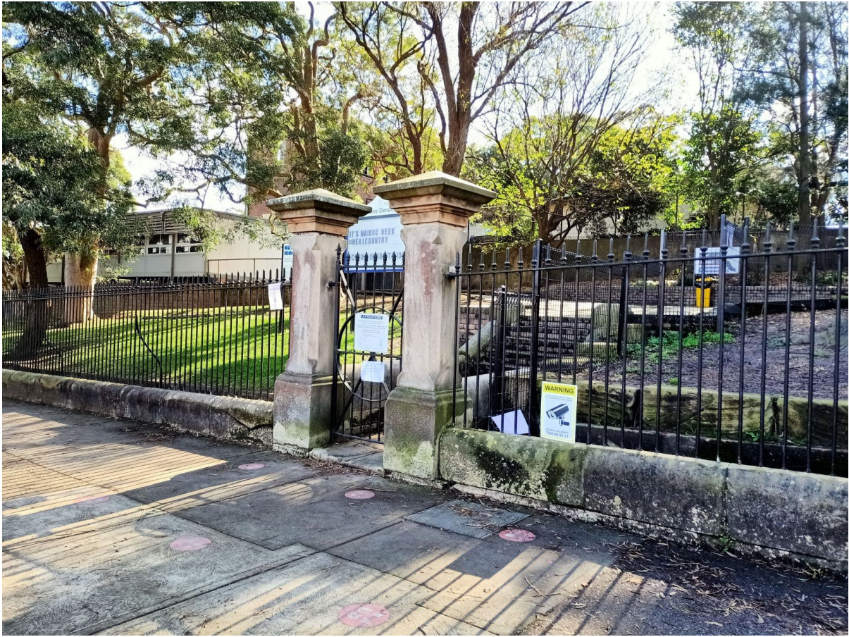
Figure 4.10: Former Crows Nest House, secondary entrance gates from Bay Road. Source: Curio, 2021.
