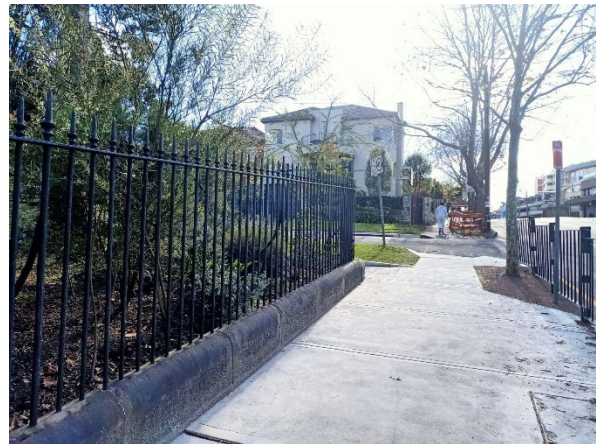
Figure 4.6: Heritage boundary wall/fence on the corner of Pacific Highway and McHatton Street (view north). Source: Curio, 2021.
