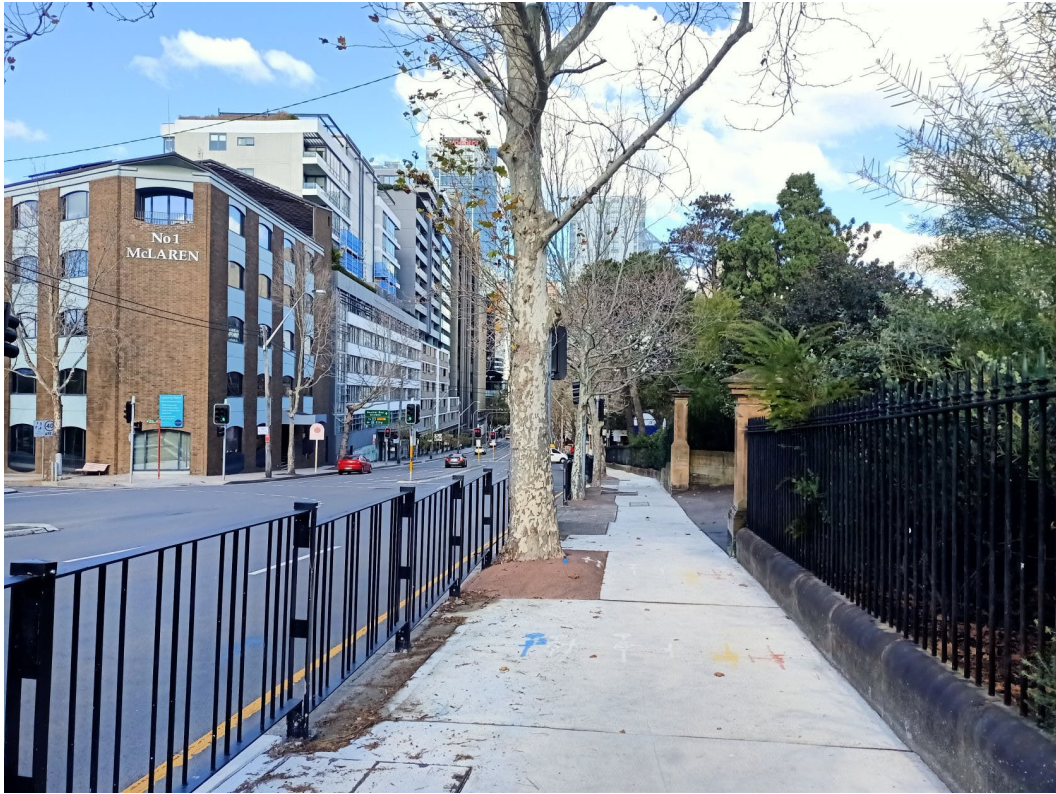
Figure 4.16: View south along Pacific Highway from McHatton St intersection, Crow's Nest gates and fence form part of the streetscape, along with overarching character of mature trees and plantings within the NSPS Site (Curio 2021)
