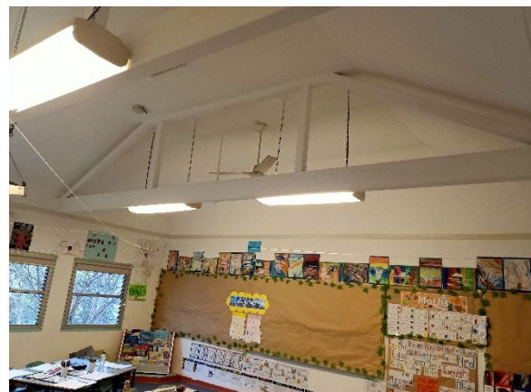
Figure 4.67: Timber beam trusses and suspended lighting in eastern classroom (Curio 2021)
