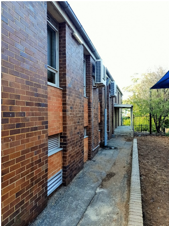
Figure 4.51: Western elevation showing recessed contrasting brickwork panels with upper aluminium windows and lower aluminium vents, rear entrance porch in background of image (Curio 2021)
