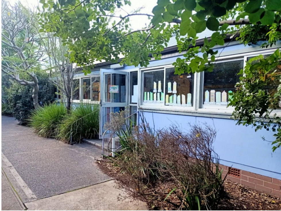
Figure 4.59: The Haven, northern elevation, fibre-board and timber clad connecting corridor constructed on brick foundations (Curio 2021)
