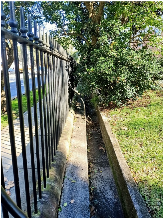
Figure 4.44: Concrete drainage channel constructed against the rear of the sandstone heritage wall along Bay Road (Curio 2021)
