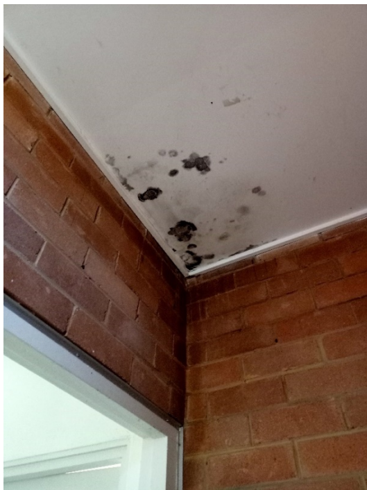
Figure 4.57: Mould on the ceiling in the southwestern corner of the hall, near the stage, reflective of ongoing issues with roof leakage and water damage (Curio 2021)
