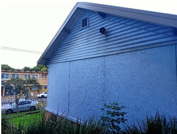
Figure 4.60: Eastern elevation, concrete panels and timber gables, Bay Street visible in background (Curio 2021)
