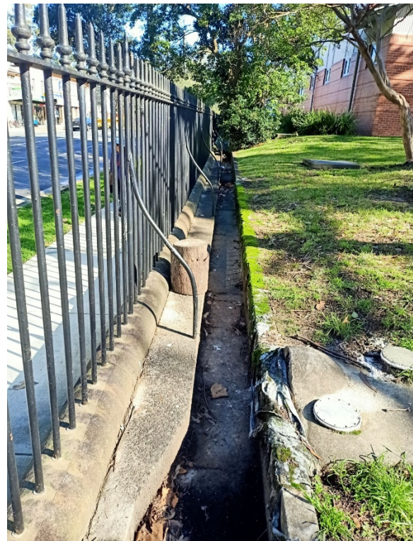
Figure 4.45: Concrete drainage channel constructed against the rear of the sandstone heritage wall along Bay Road (Curio 2021)
