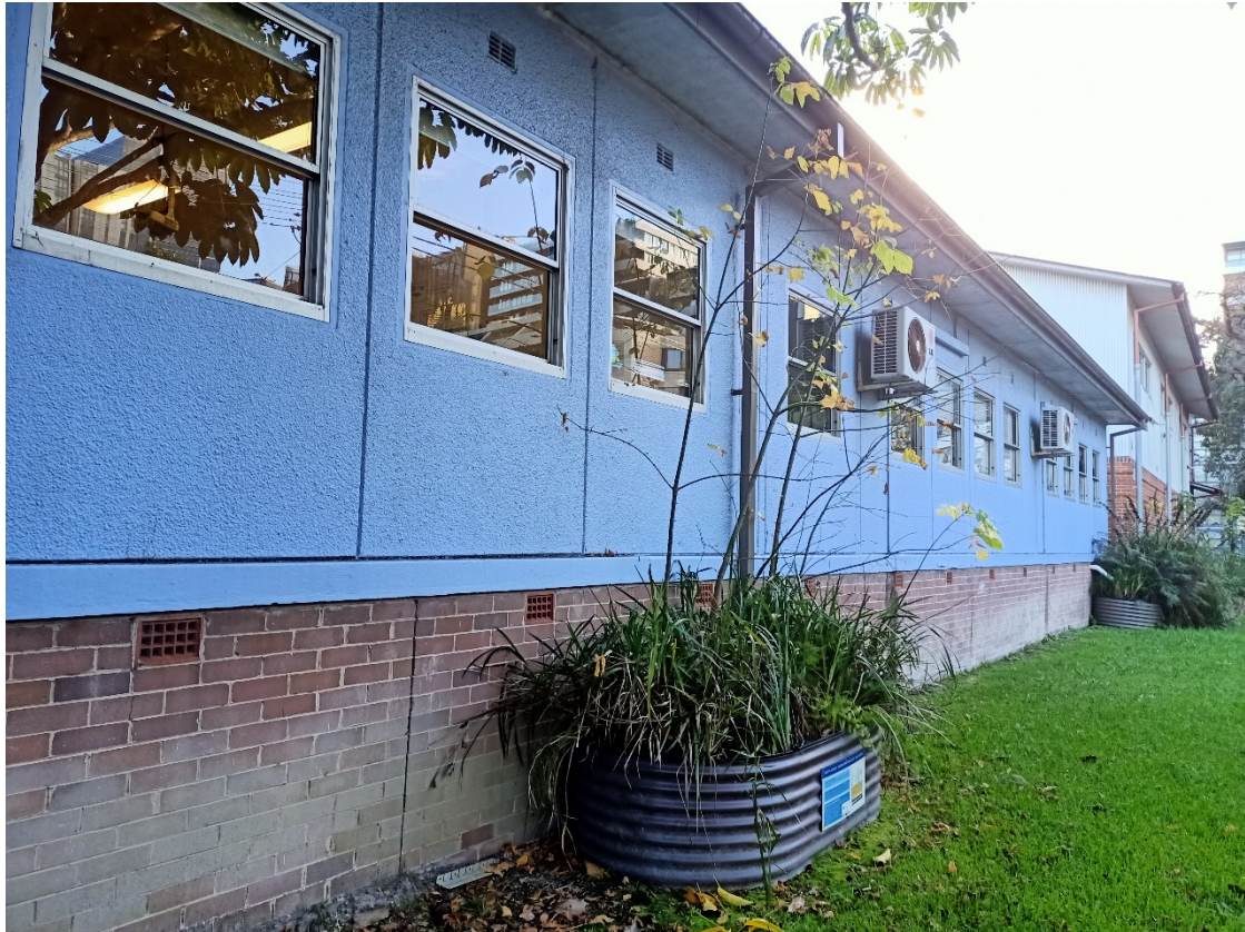
Figure 4.62: Haven southern elevation, pre-cast concrete panels apparent, with aluminium framed double hung windows and brick foundations. Building G (library) visible in background to east of building (Curio 2021)
