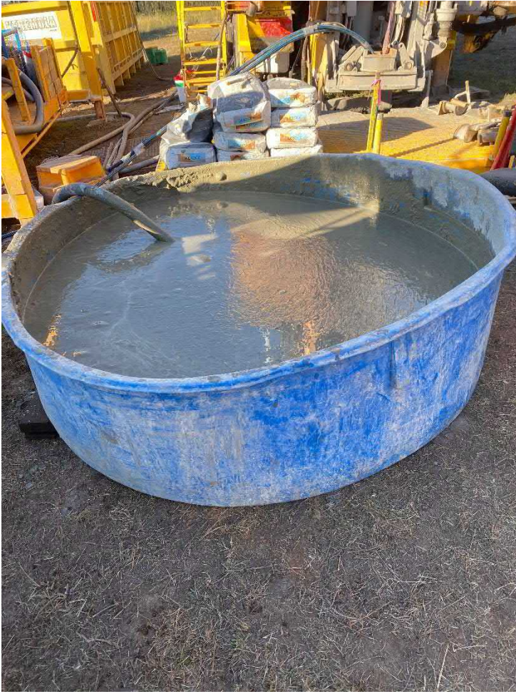
Figure A 2.3 VWP grout mix consistency (VWP CHES_016 grout mix shown)
