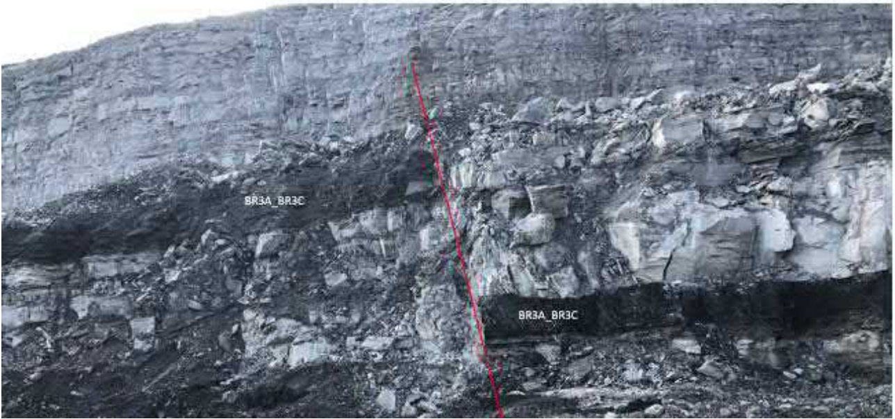
Figure 4.12 Carrington Pit Fault
