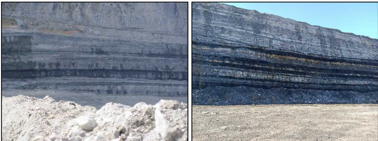
Figure 6.8 Groundwater seepage from coal seams in Cheshunt Pit (left) and Carrington Pit (right)
