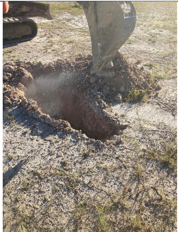
Photograph 24 – Test pitting on the soil mound.
