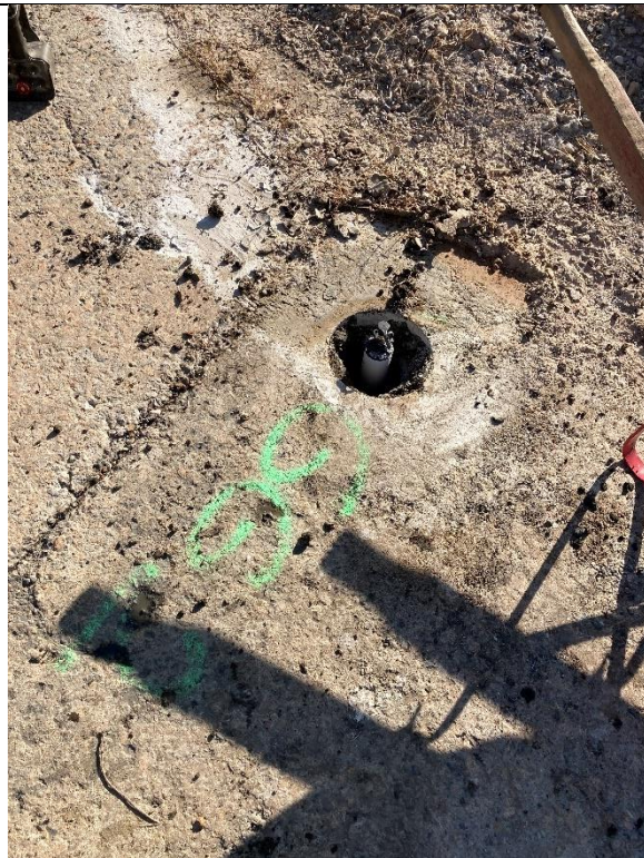
Photograph 11 – installed well with plug (before cap was installed).
