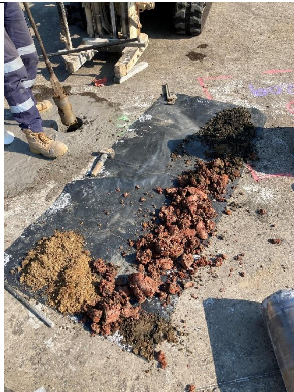
Photograph 7 – Concrete coring and hand auguring.
