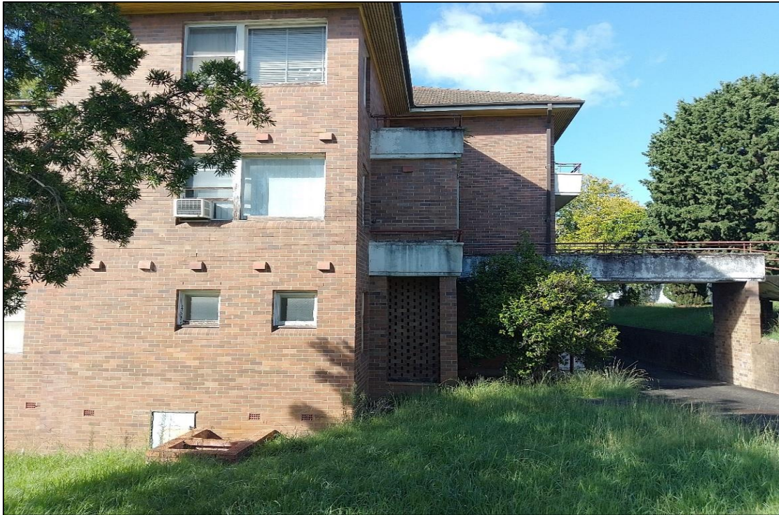
Photograph 3 - Drainage pit on northern side of nurses quarters at 72 Menangle Road.
