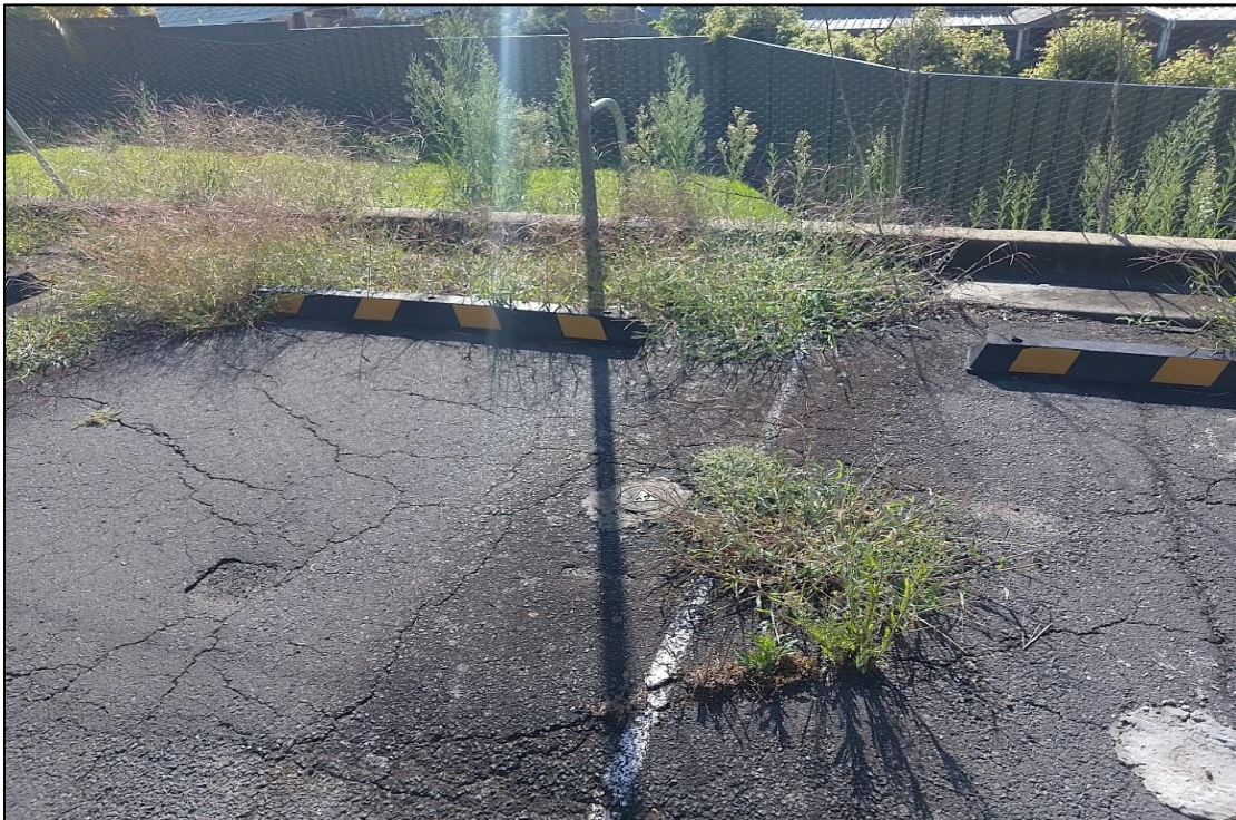
Photograph 6 - Groundwater monitoring wells in carpark to the northeast of nurses quarters
