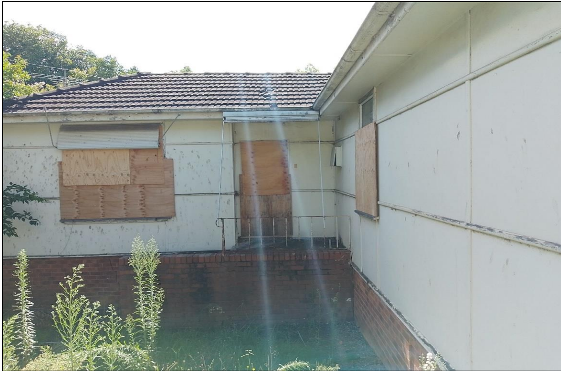
Photograph 15 - Building at 86 Menangle Road
