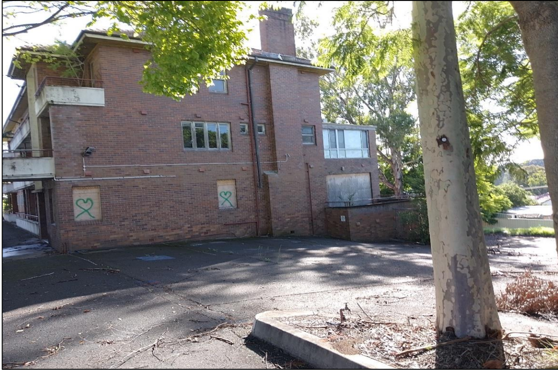
Photograph 5 - Southern side of nurses quarters at 72 Menangle Road.
