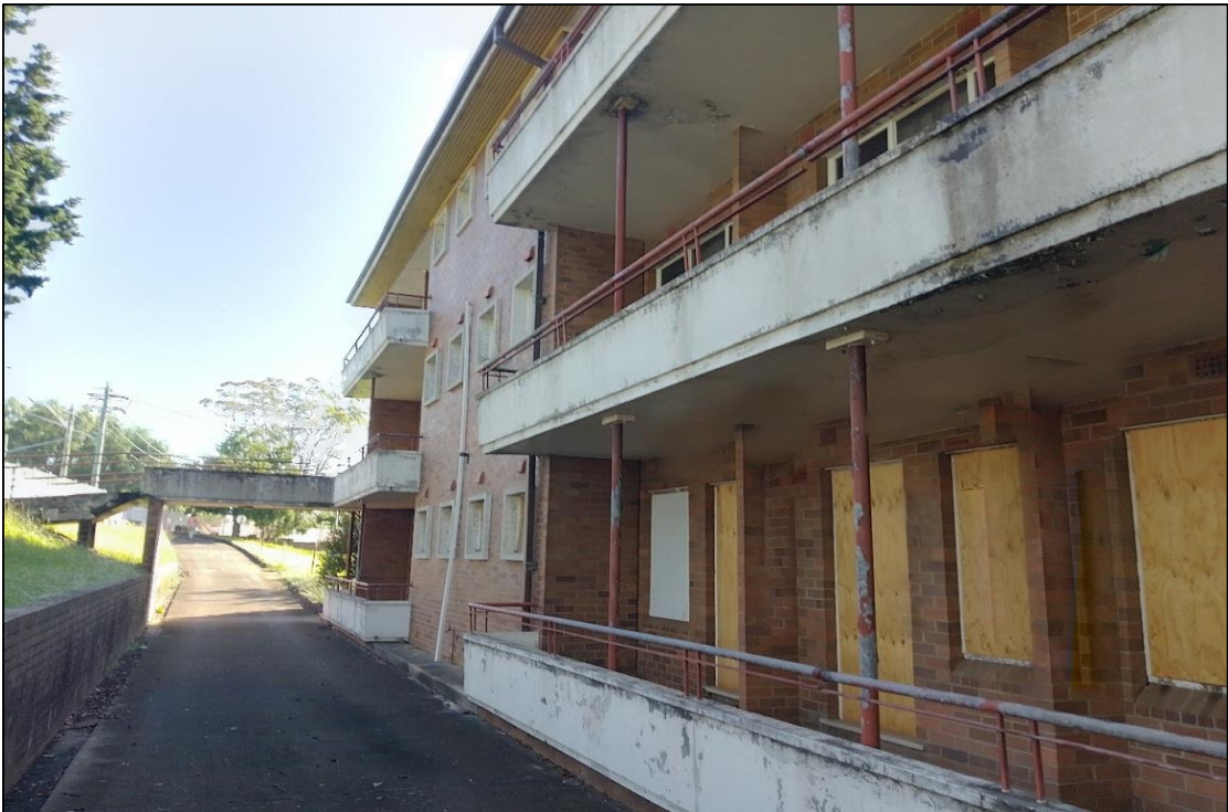
Photograph 4 - Potential fill to the immediate north of the nurses quarters at 72 Menangle Road.
