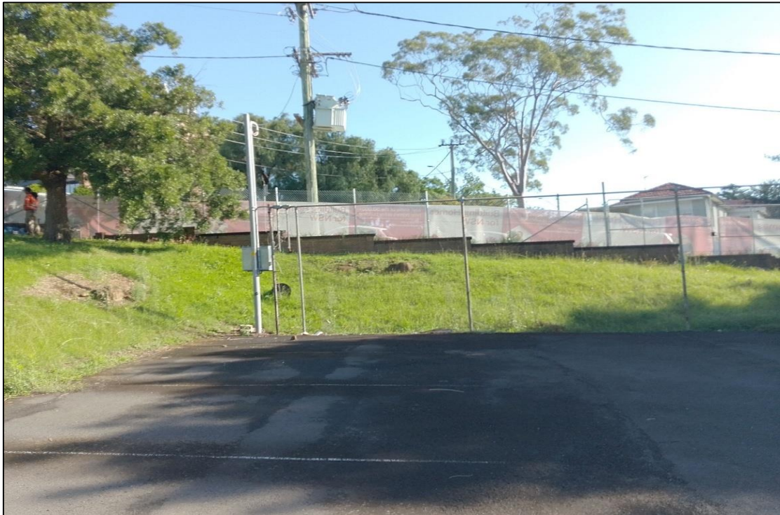
Photograph 2 - Potential fill at northern end of 72 Menangle Road.
