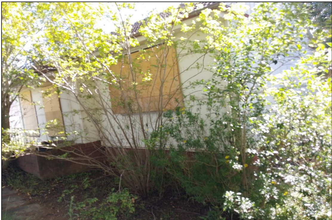
Photograph 10 - Building at 84 Menangle Road constructed of PACM sheeting
