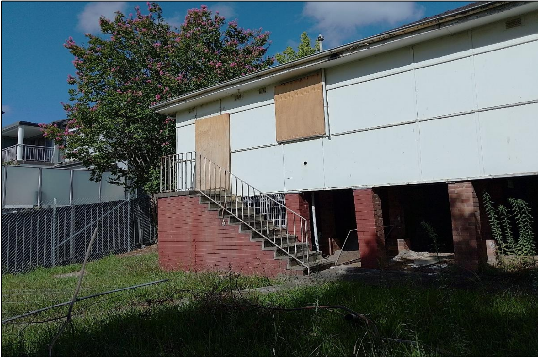
Photograph 13 - Building at 86 Menangle Road constructed of PACM sheeting
