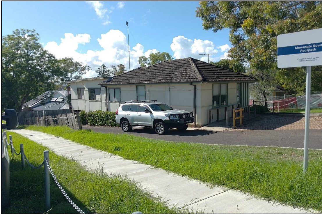
Photograph 7 - Health services building at 82 Menangle Road.
