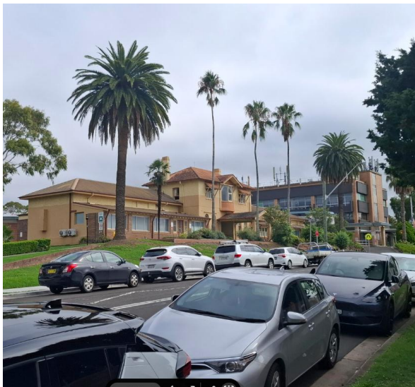
Figure 21: View towards Camden Hospital
