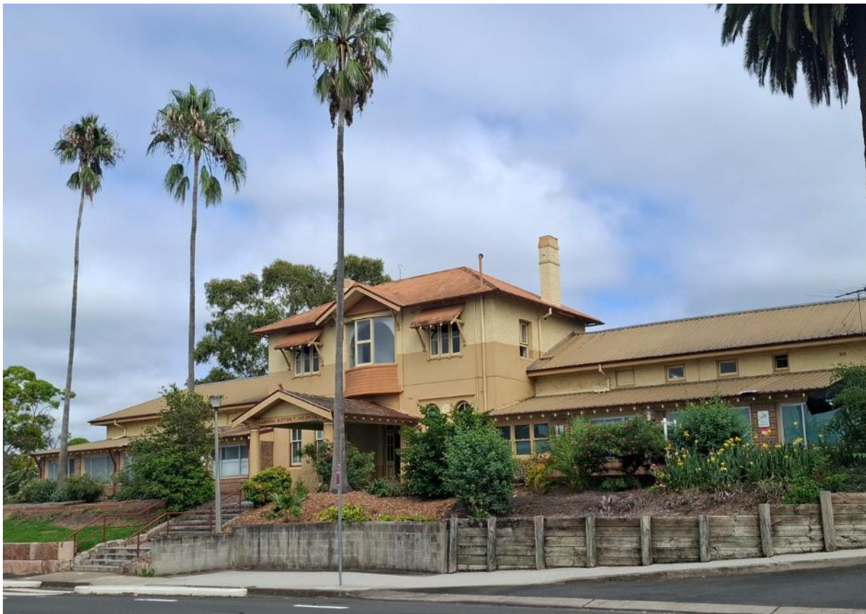
Figure 35: Front façade of Camden District Hospital
