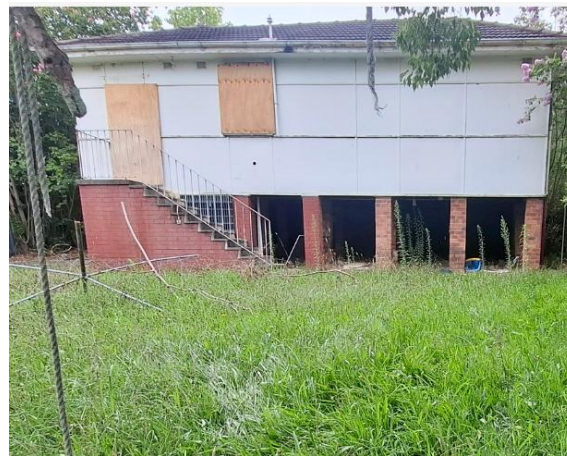
Figure 34: Rear elevation of number 86 Menangle Road
