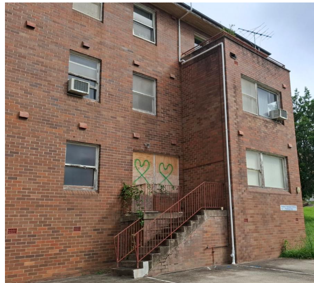
Figure 28: View of a section of the rear of the former nurses quarters.
