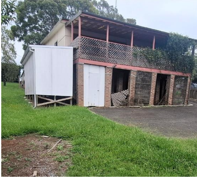
Figure 31: View to the rear of 82 Menangle Road
