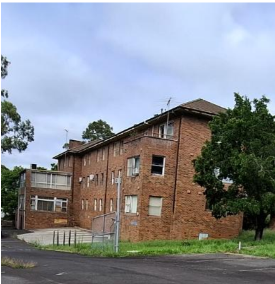
Figure 27: View of the rear and side of the former nurses quarters taken from the driveway at the rear of the building
