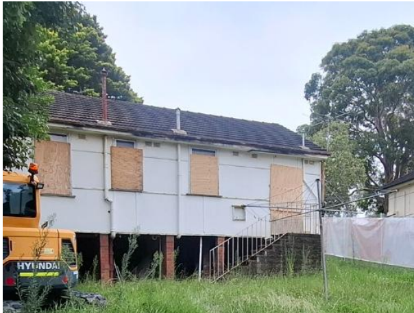
Figure 33: Rear elevation of 84 Menangle Road
