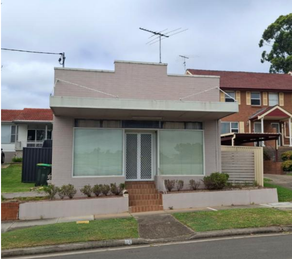
Figure 23: Front façade of locally listed 'Corner Shop' located on Macquarie Avenue
