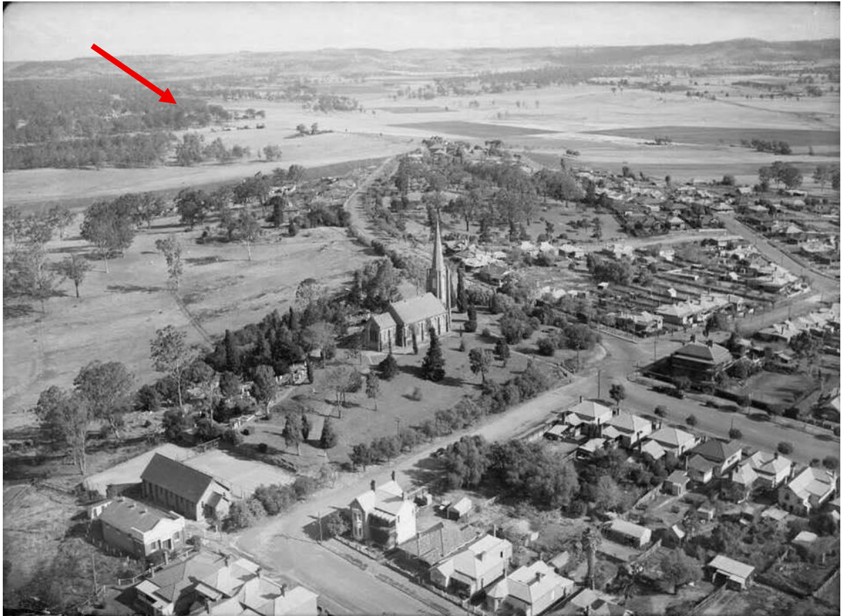
Figure 15: An aerial view of Camden township in 1940 taken by plane that took off at Camden airfield. St John's Church is at the centre of the image; indicative location of study area pointed out (Source: Camden Library)
