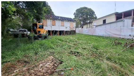
Figure 8: Rear of the property at 86 Menangle Road, facing northwest.
