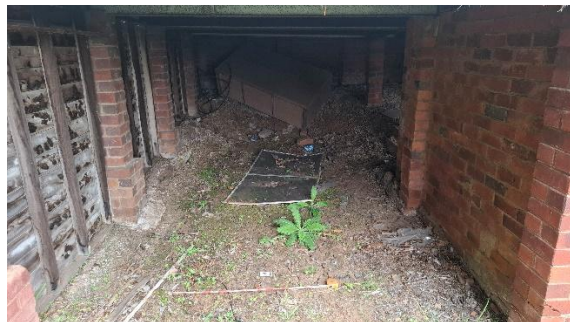
Figure 9: Exposure under dwelling at 86 Menangle Road, facing west.
