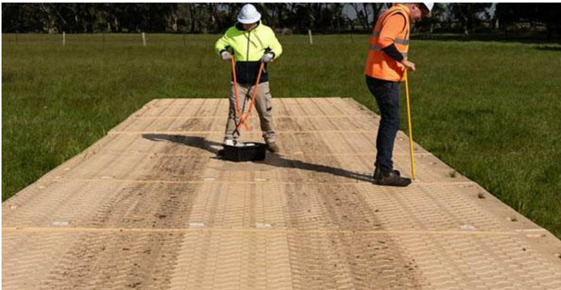
Figure 3.2 – Example of acceptable Tree Protection Area ground protection (Source: Samson)
