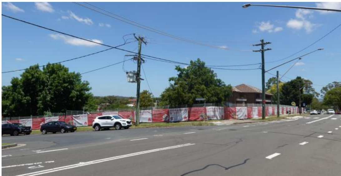
Figure 1.2 – View of the site looking south-east from the corner of Menangle Rd and Gilbulla Ave showing typical site conditions. (Photo: Arterra 17 December 2025)
