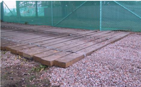
Example image of acceptable ground protection rumble boards
