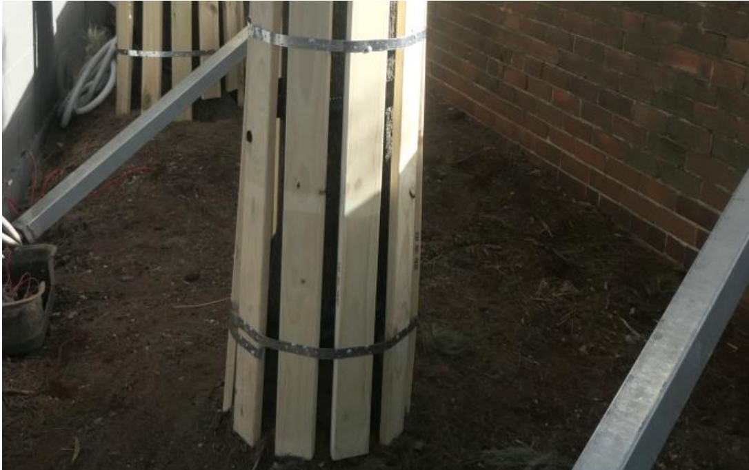
Figure 3.3 – Acceptable Trunk Protection batten installation – height of boards to be at least 2.4m or to the first branches. (Photo: Arterra)
