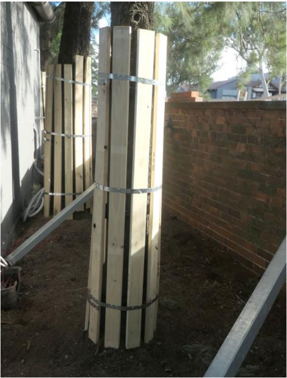
Example image of acceptable trunk protection battens
