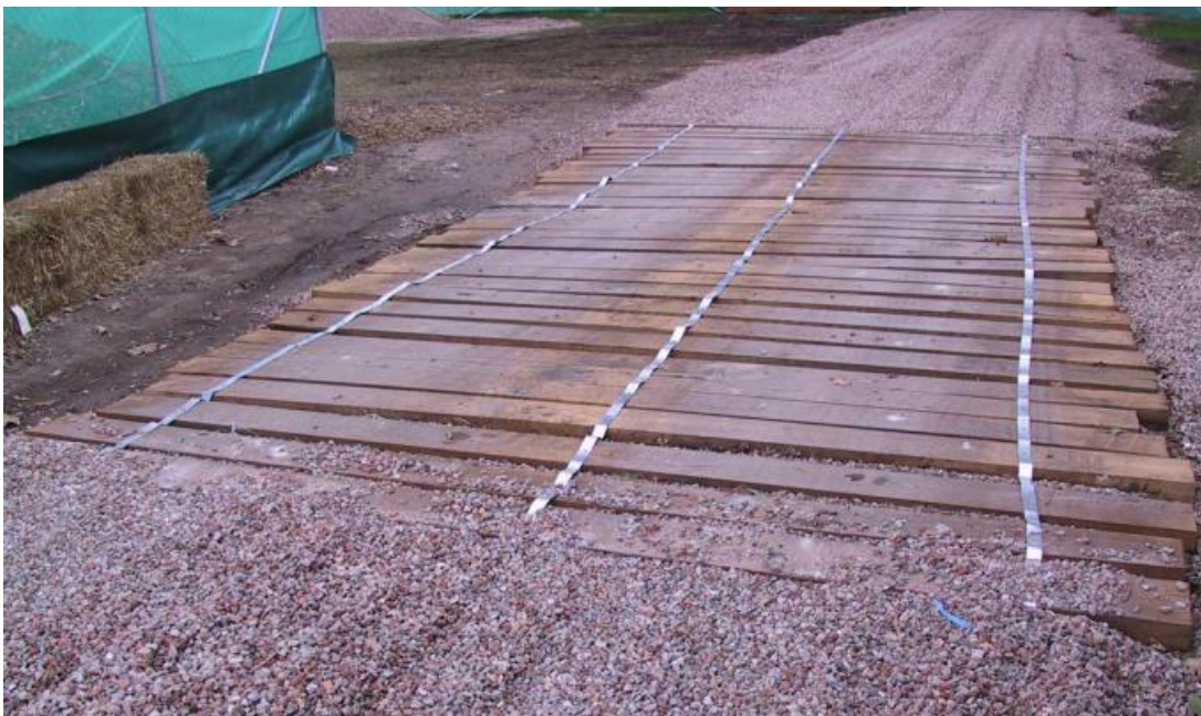
Figure 3.1 – Example of acceptable Tree Protection Area ground protection (Photo: Arterra)
