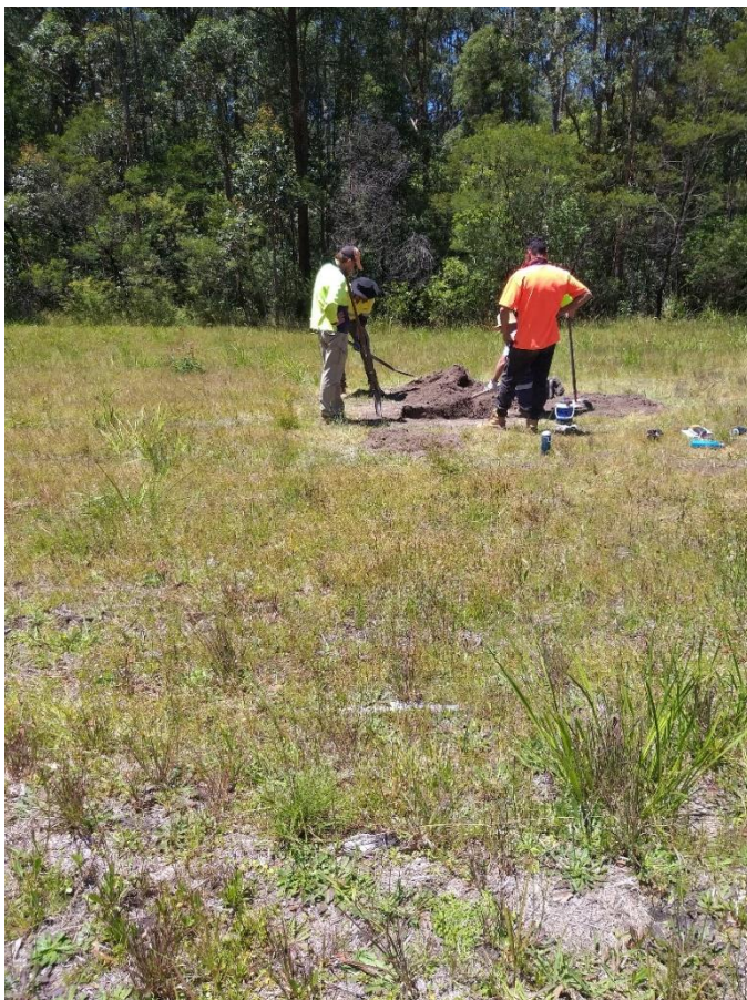
Plate 12 Excavation detention basin 2
