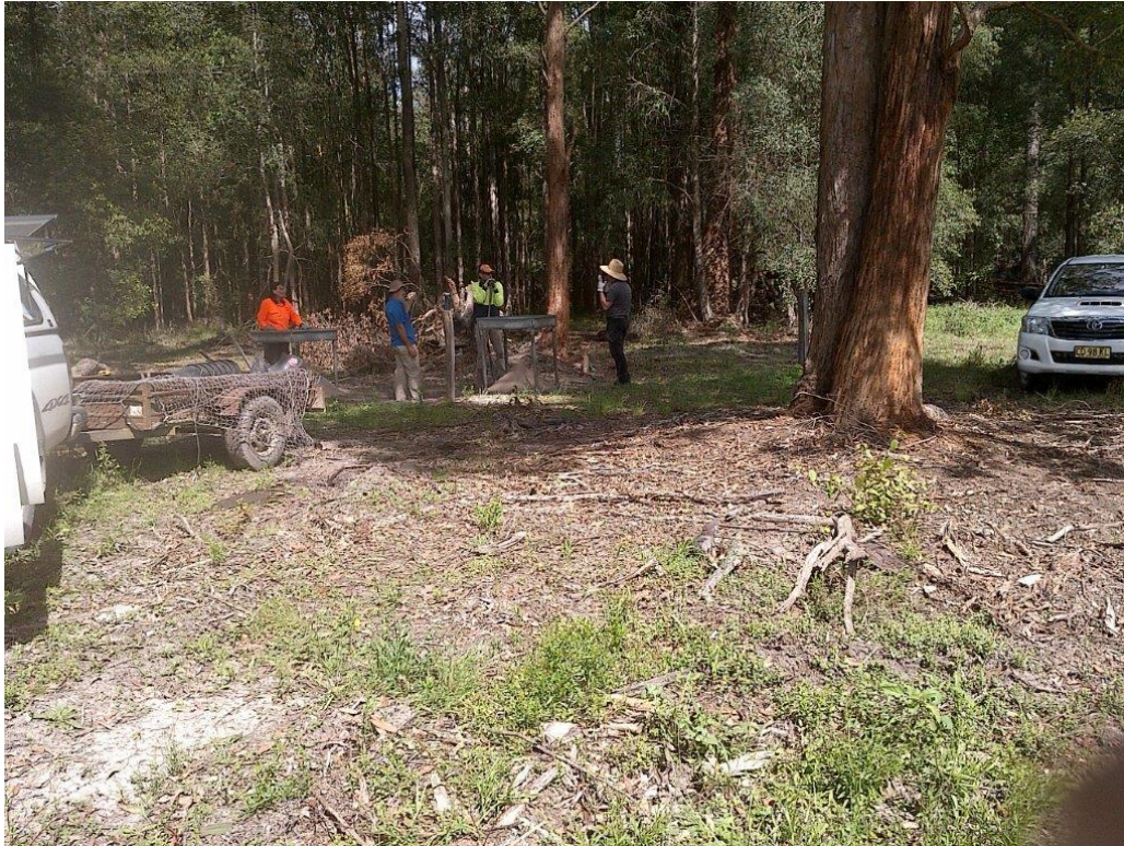
Plate 11 Excavation area below the primary stockpile
