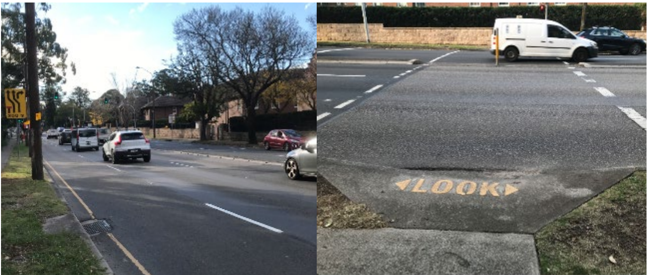
Photograph 18: Rhyolite in the traffic lights braking area before a School Crossing on the Pacific Hwy A1, Wahroonga 24-6-2021.
