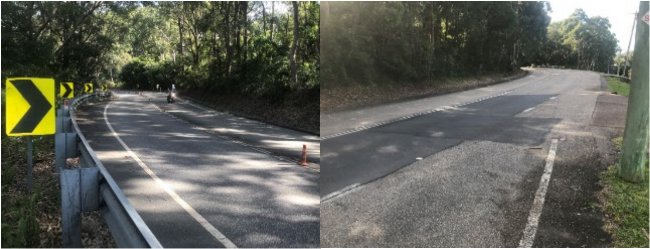
Photograph 13: Rhyolite on bends Warners Bay Road, Charlestown, sections are in poor condition or replaced with general asphalt (possibly slag) taken on 23-6-2021.
