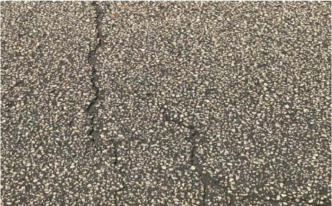
Photograph 6: Close up of the lighter coloured pavement, showing light coloured rhyolite aggregate within a bitumen matrix
