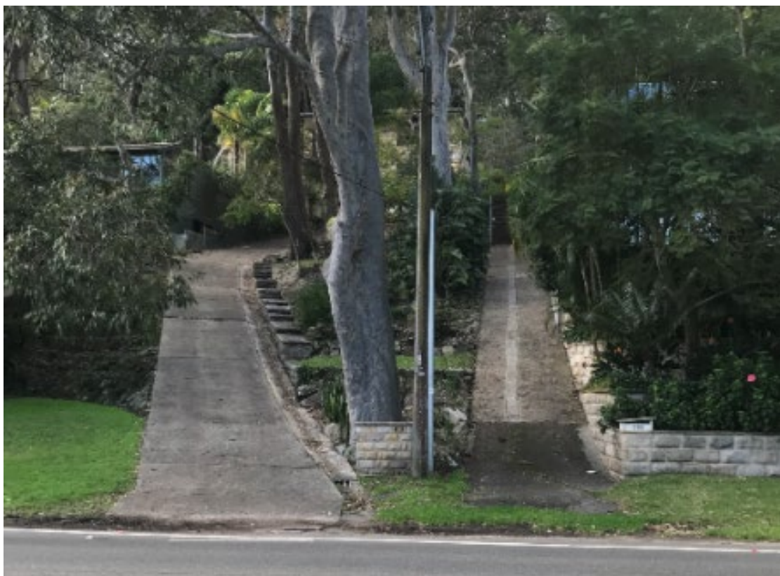
Photograph 20: Steep driveways where high PAFV materials would assist in a domestic environment.
