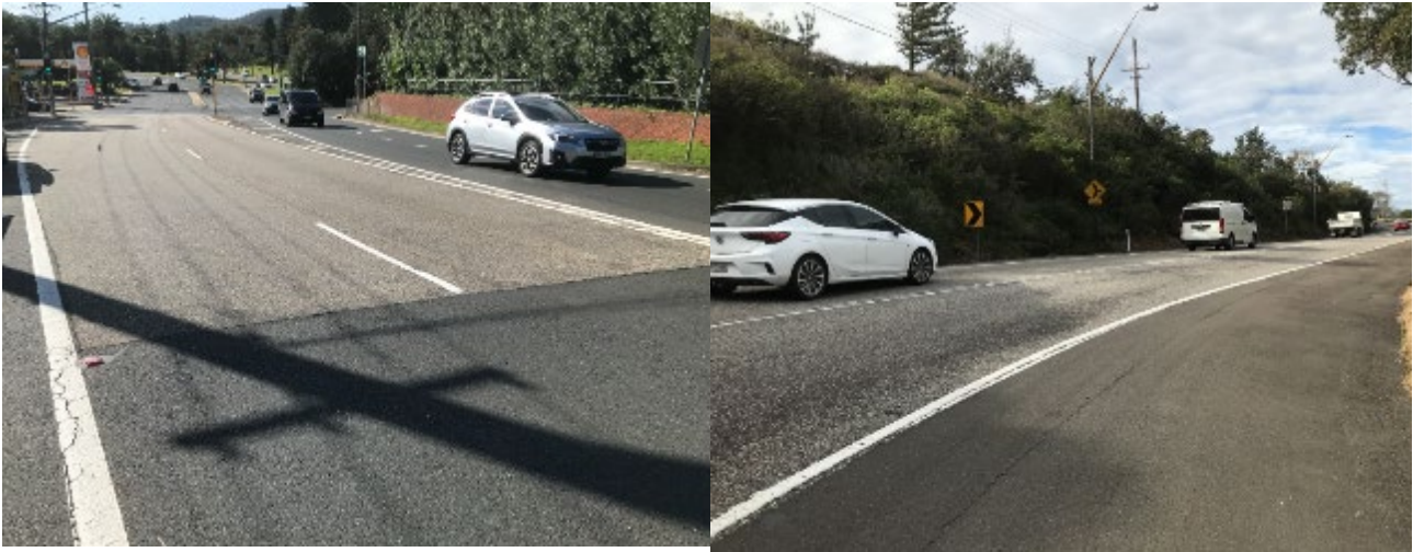
Photograph 17: Rhyolite in traffic lights braking area Barrenjoey Road, Avalon Beach 24-6-2021 in good condition. and on bends Barrenjoey Road, Bilgola Beach 24-6-2021 in reasonable condition.
