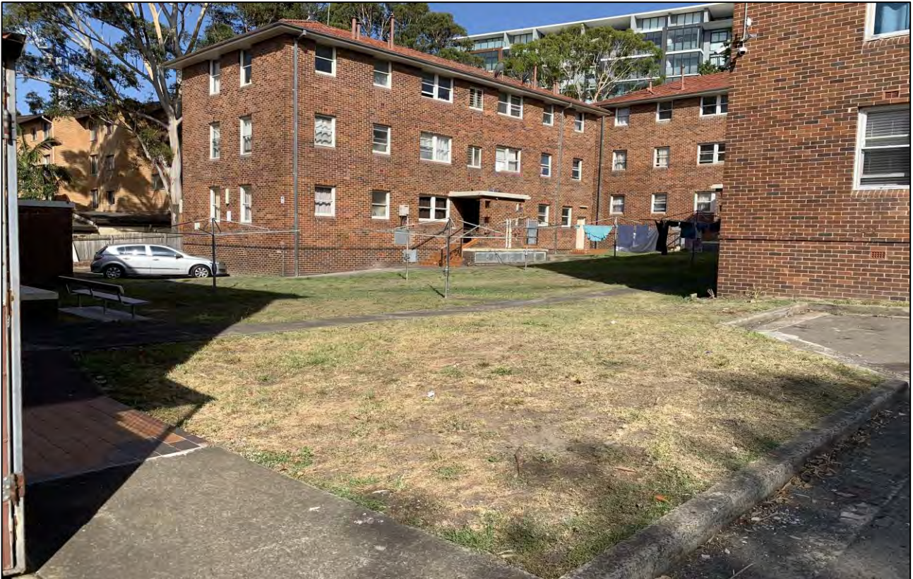
Photograph 1. Blocks 8, 7, 6 and communal gardens of the northern portion of the subject site (facing north east). Date: 01.12.2020.
