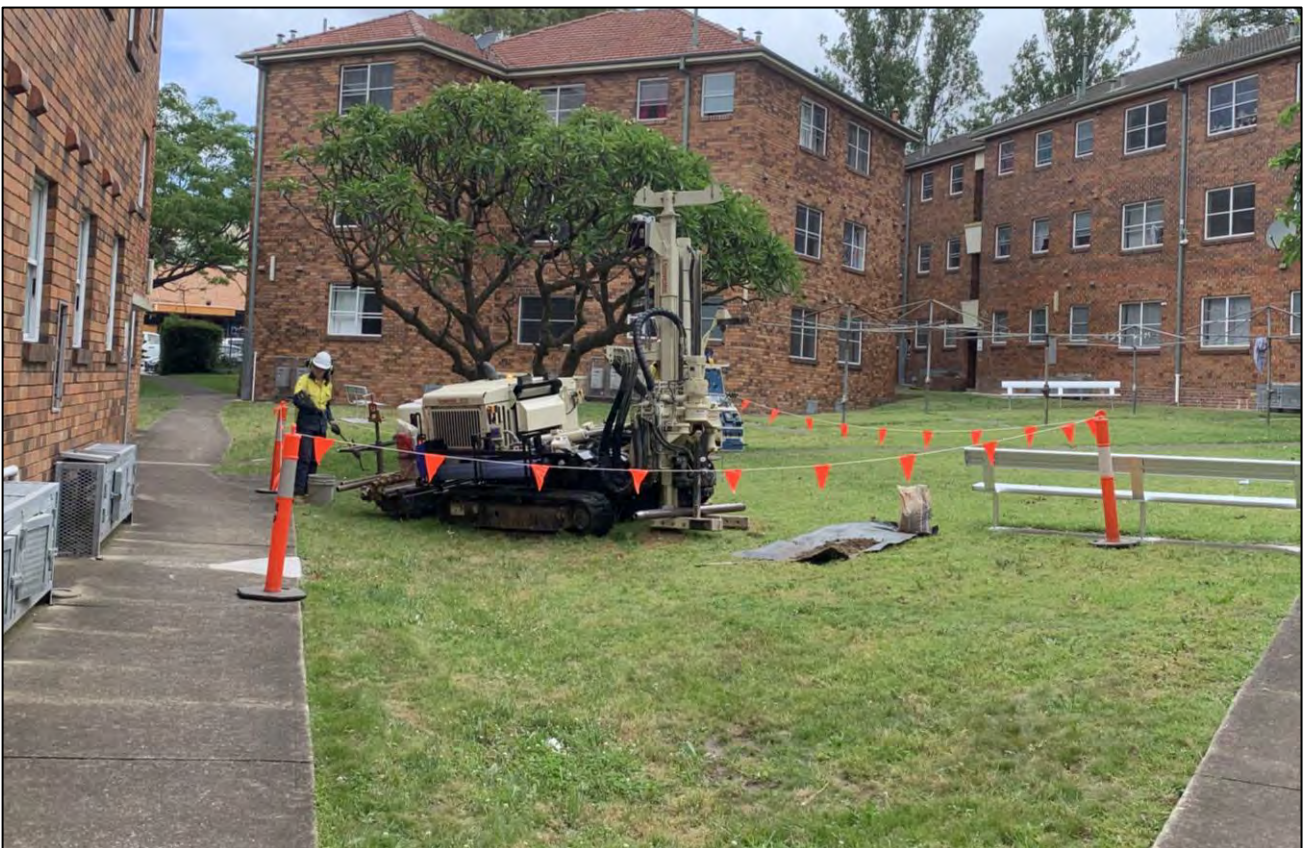
Photograph 4. Drill rig setup and work zone delineation area. Date: 30.12.2020.
