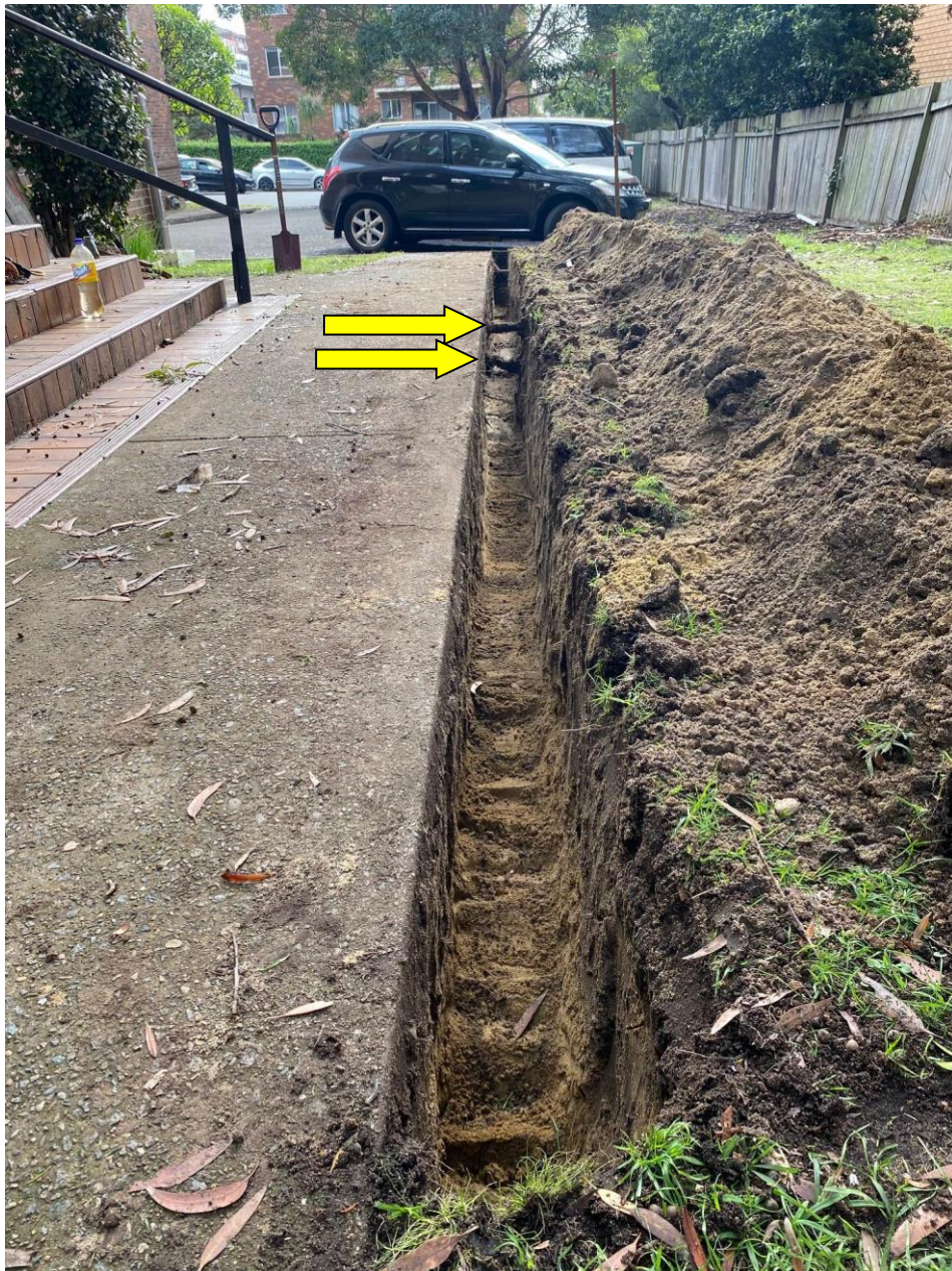
Figure 1: Root investigation trench within TPZ of Tree 109. Arrows show location of roots.
