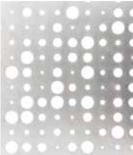
Perforated metal to the podium balconies
