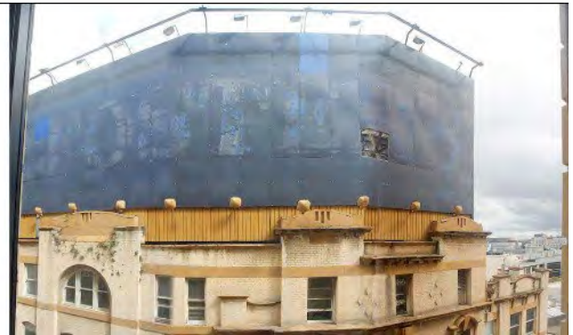
Existing situation – view from adjoining hotel
