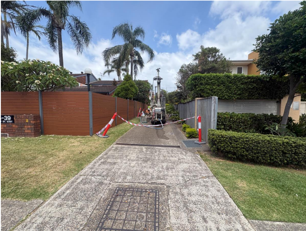
Photograph 1 View of residential buildings at 35-39 Darley Street East, with concrete driveway, Looking south-west.
