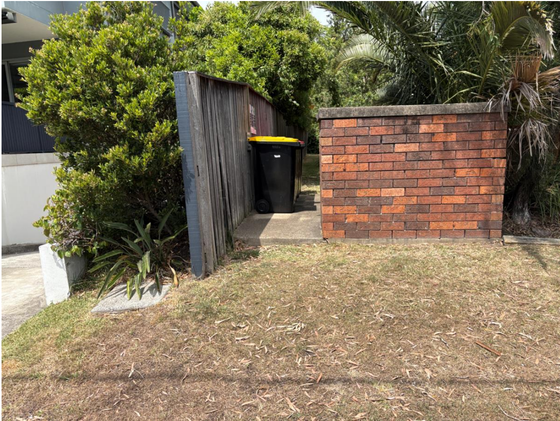
Photograph 4 Residential waste storage area (garbage bins) located adjacent to the building along the north-eastern boundary
