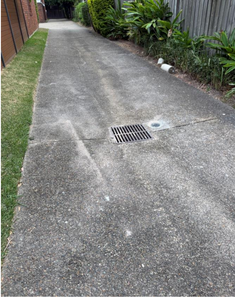
Photograph 3 View of the concrete driveway with associated stormwater drainage and a groundwater monitoring well (installed as part of the geotechnical investigation).
