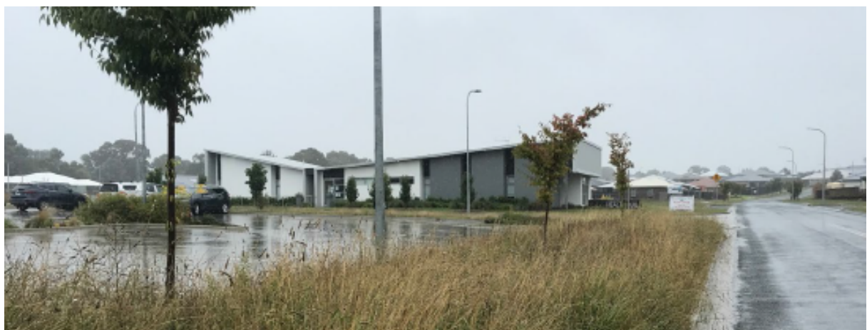
Figure 2-4 Site frontage looking west along Fairley St Source: Pedavoli Architects
