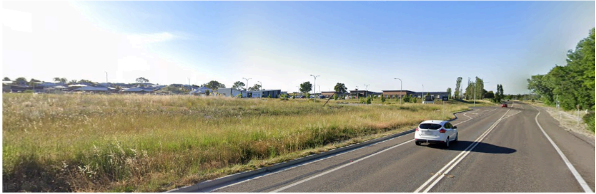
Figure 7-2 View 1: Looking NW from Barton Hwy frontage Source: Google
