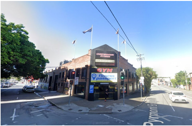
Figure 3 View of existing development as viewed from corner of Pymont Bridge Road and Mallett Street looking southwest
