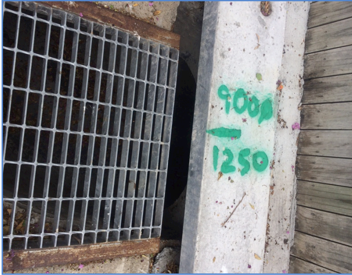
Figure 12. Storm water drain showing depth of trench and width of pipe at the end of Eurimbla Avenue
