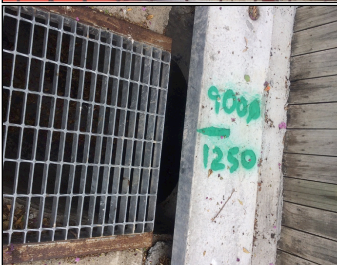
Figure 9. Storm water drain showing depth of trench and width of pipe at the end of Eurimbla Avenue
