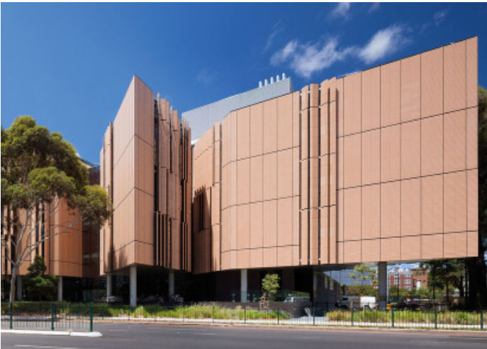
Name: Tyree Energy Technologies Building Architect: FJMT Year: 2012
