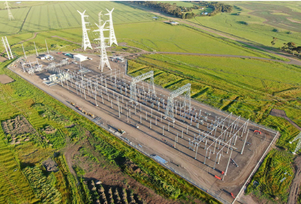
Image 2 Typical Switching Station (Source: Neoen)
