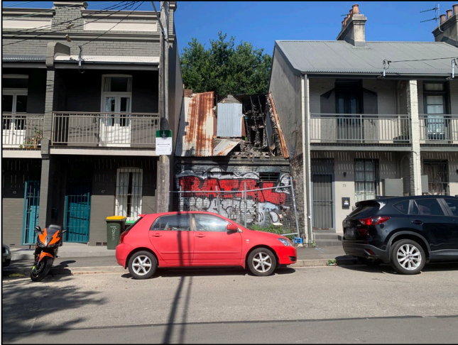
Figure 6 – Terraces Located Along Eveleigh Street
