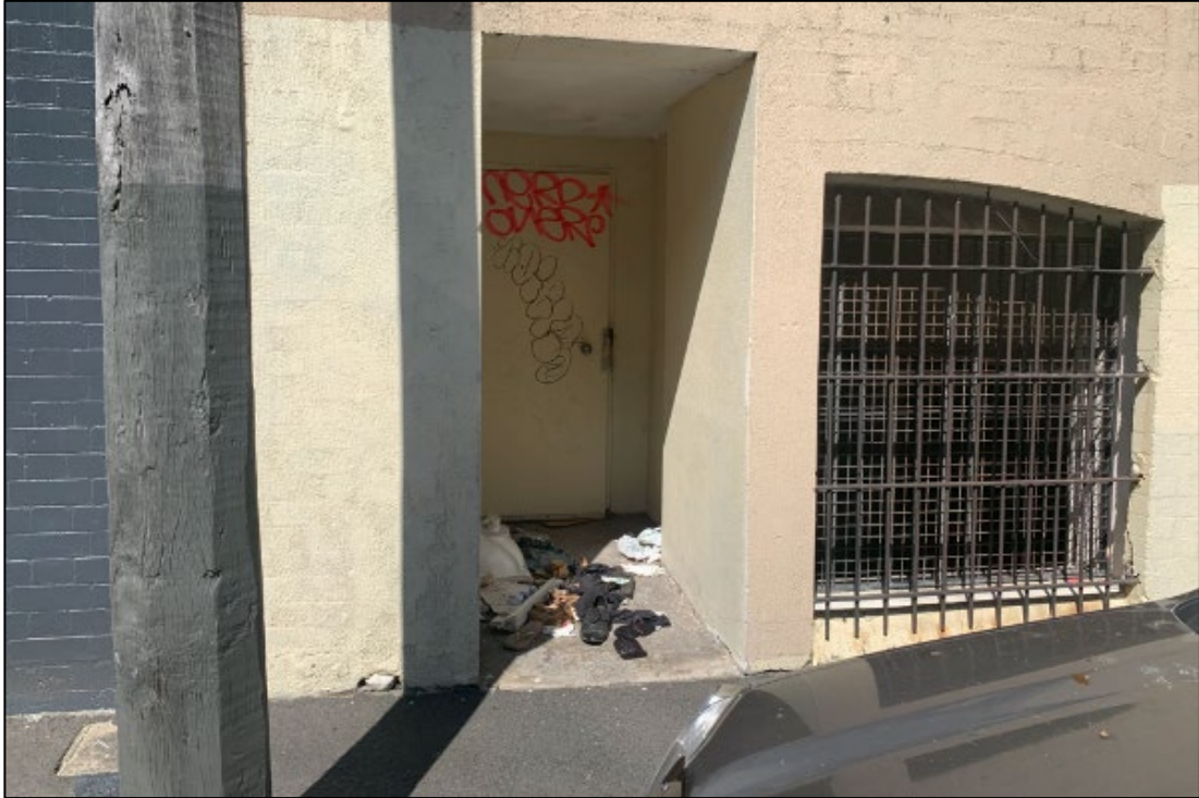
Figure 4: Eastern Elevation Fronting Eveleigh Street
