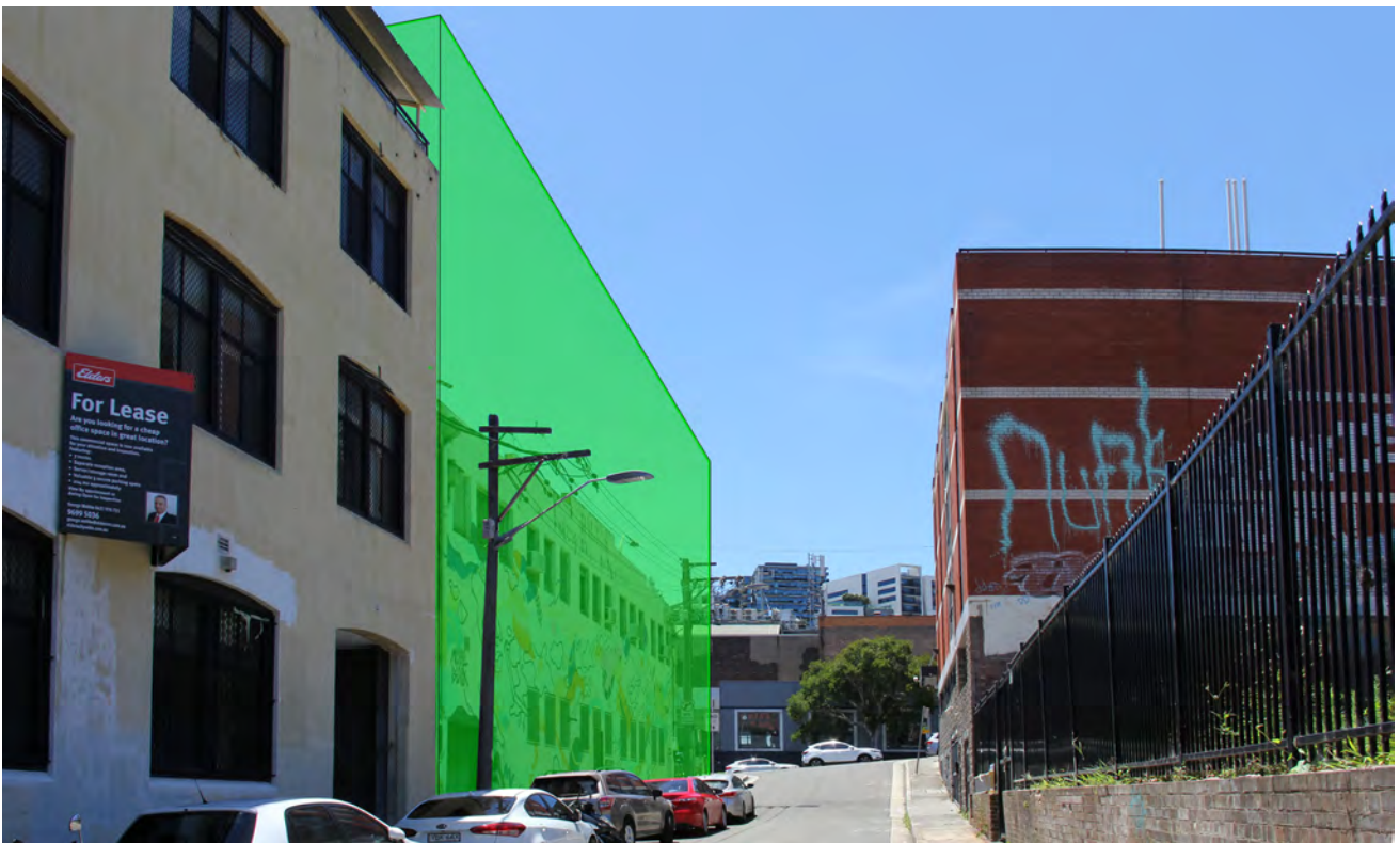
Viewpoint No.6 – Visual impact of compliant building envelope shown in green overlay
