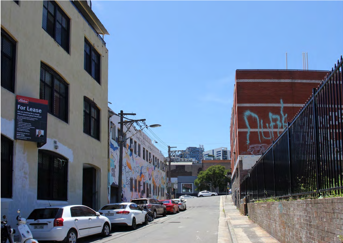
Viewpoint no.6: Existing site photo. Pavement level - standing height - to the south of the subject site. On the eastern side kerb of Woodburn Street, 57m south of the junction with Cleveland Street, adjoining 7, Woodburn Street. Distance to site boundary: 22.2m. Distance to centre of subject site: 44.8m RL of camera: + 21.74
