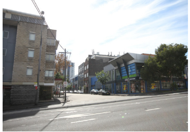
Figure 3.6 The nature of contemporary development on the northern side of Cleveland Street, directly opposite the subject site. Source: GBA Heritage
