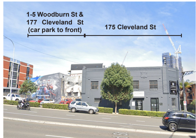
Figure 3.2 Northern elevation of 175 Cleveland Street and 1-5 Woodburn Street. 177 Cleveland Street constitutes the carpark. Source: Google Streetview 2020
