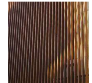
6 LOUVRE BLADES DARK BRONZE FINISH, MAY INCORPORATE ARTWORK DESIGN TO FUTURE DETAIL
