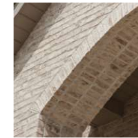
2 BRICK DETAILING TO ENTRY
