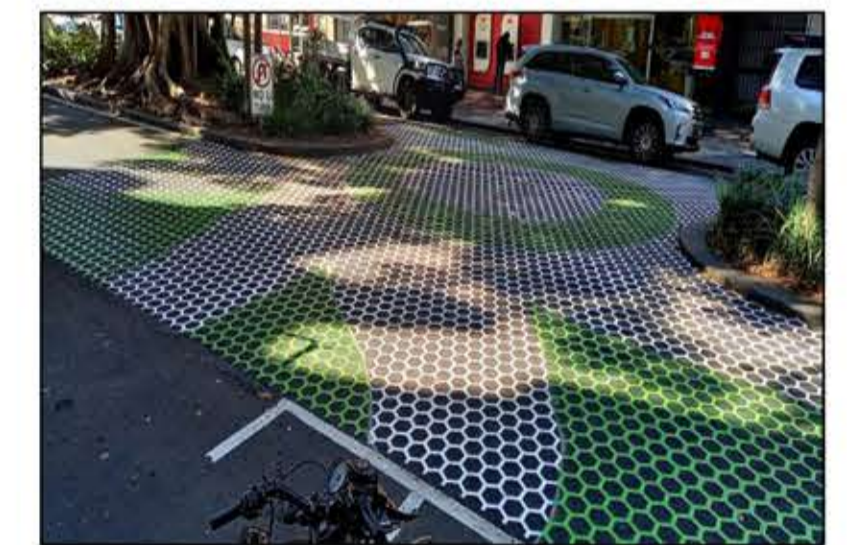
Traffic calming pavement treatment- The Corso, Manly. Suggested use to highlight focal points, intersections and way-finding.
