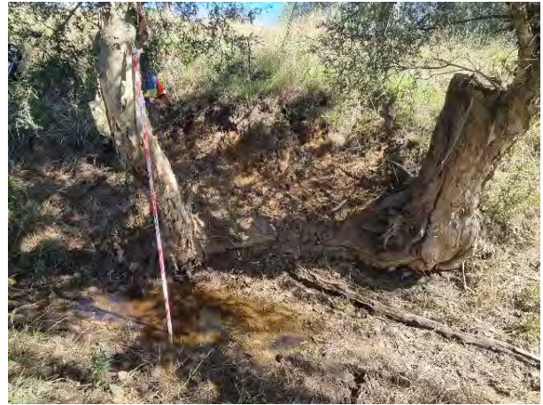
Figure 11: Soil exposure in gully erosion of minor drainage line in the north eastern corner of study area.
