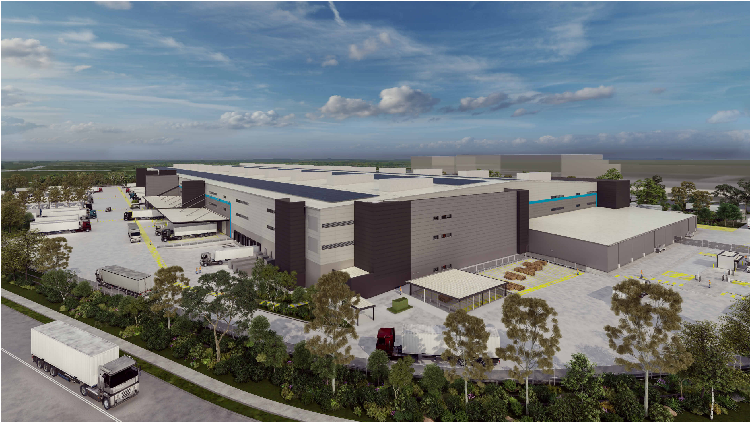
NORTHWEST VIEW - WAREHOUSE & HARDSTAND
