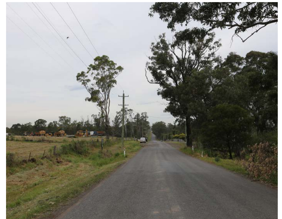
Photo 18. View south from the intersection of Lawson Road and Elizabeth Drive
