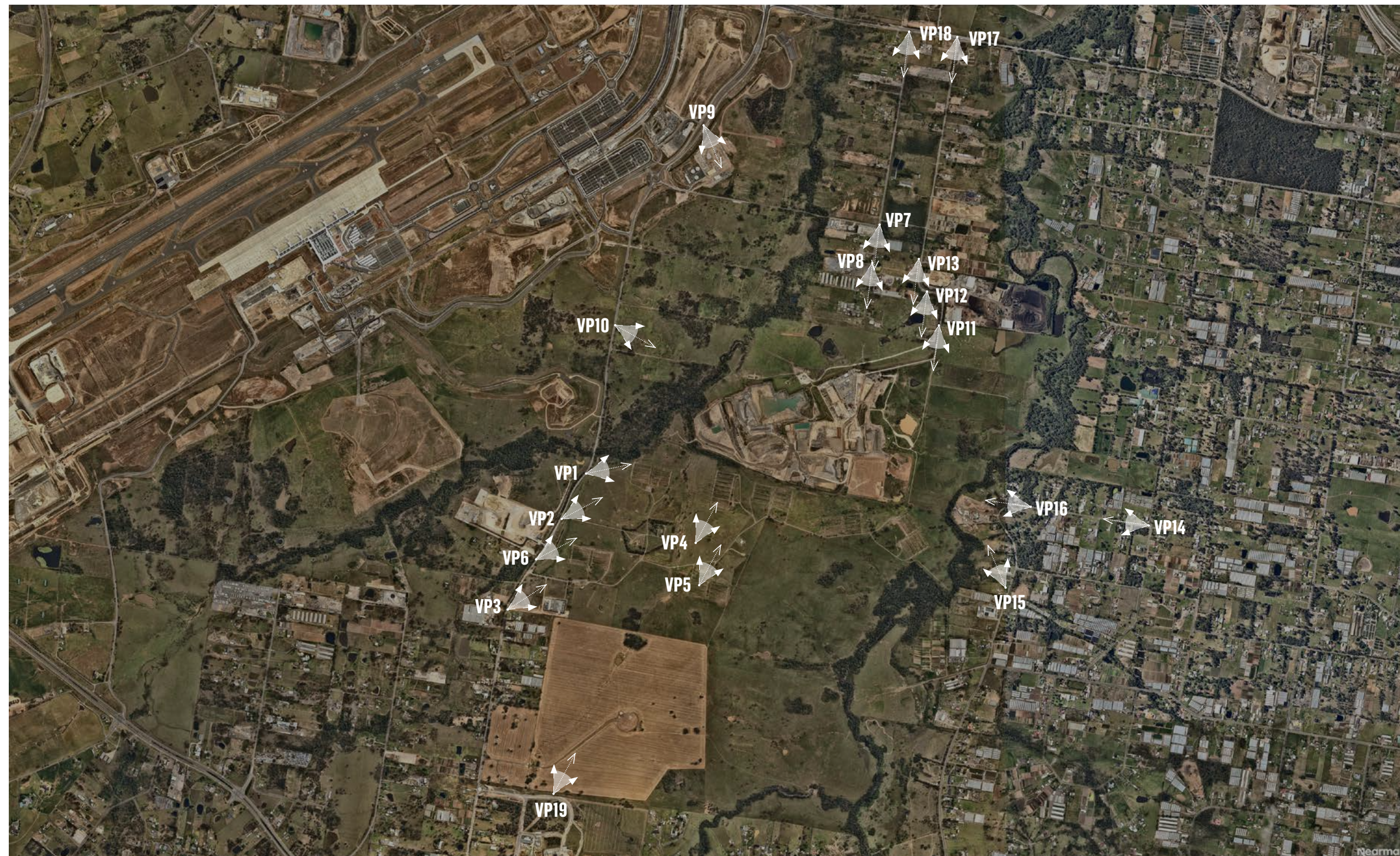
Figure 5 Locations inspected during fieldwork
