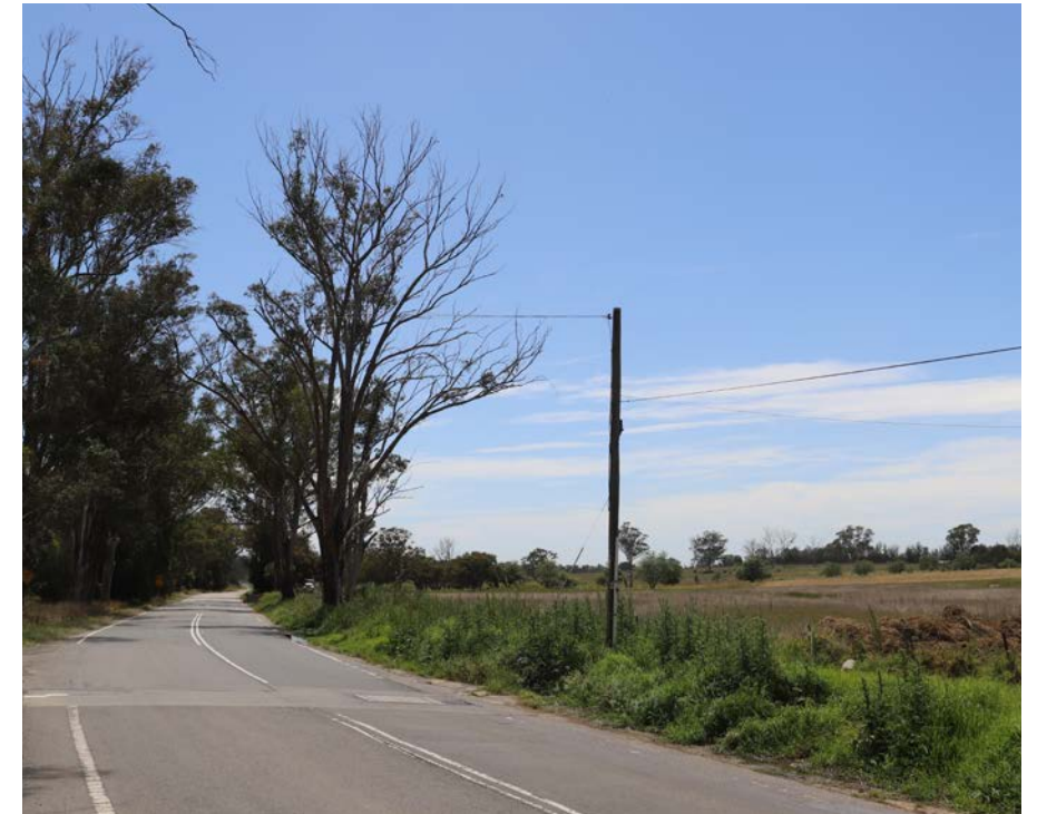
Photo 3. View north-east from 260 Badgerys Creek Road
