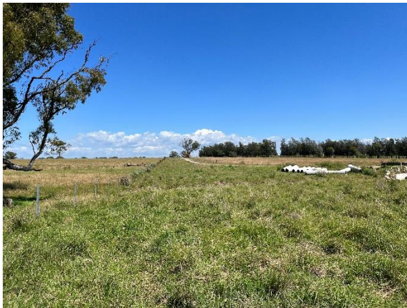
Figure 7: View of the landscape showing open grassland for grazing and drainage culvert alongside existing road
