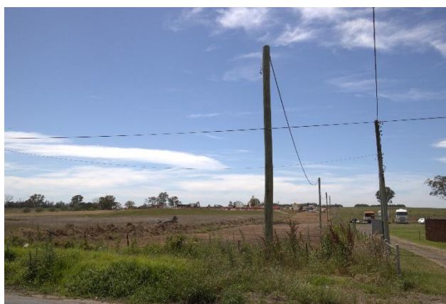
Picture 4 View of site where earthworks have commenced
