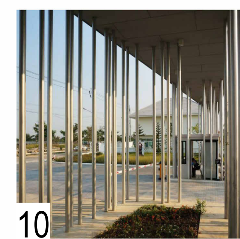
Metal columns to support canopy Colour: Light Bronze
