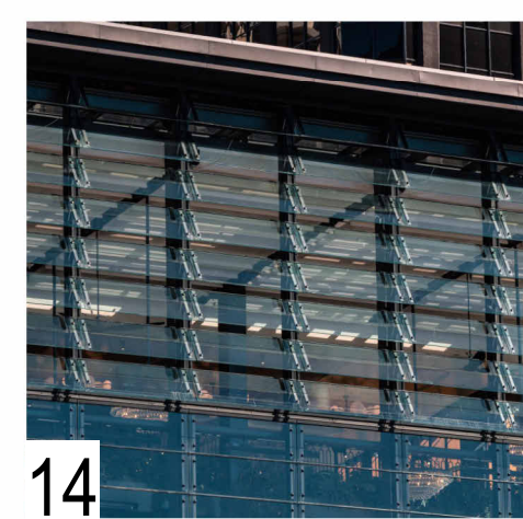
Link bridge structure with louvred glass panels.
