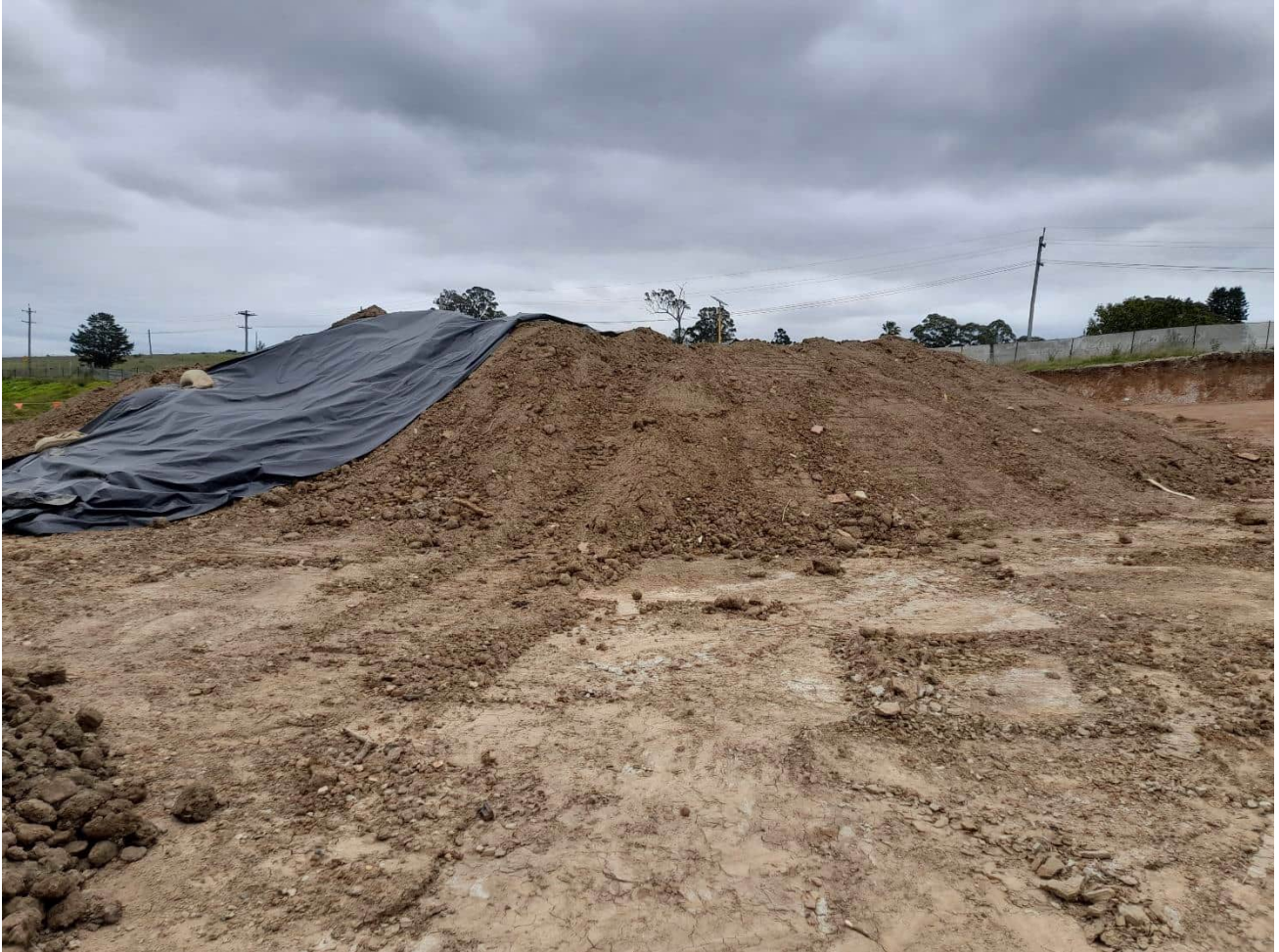
Photograph 1. Subject stockpile. Date: 09/10/2024.
