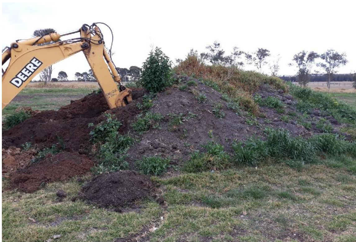
Photo 8 - AEC4D - Topsoil Fill Stockpile
