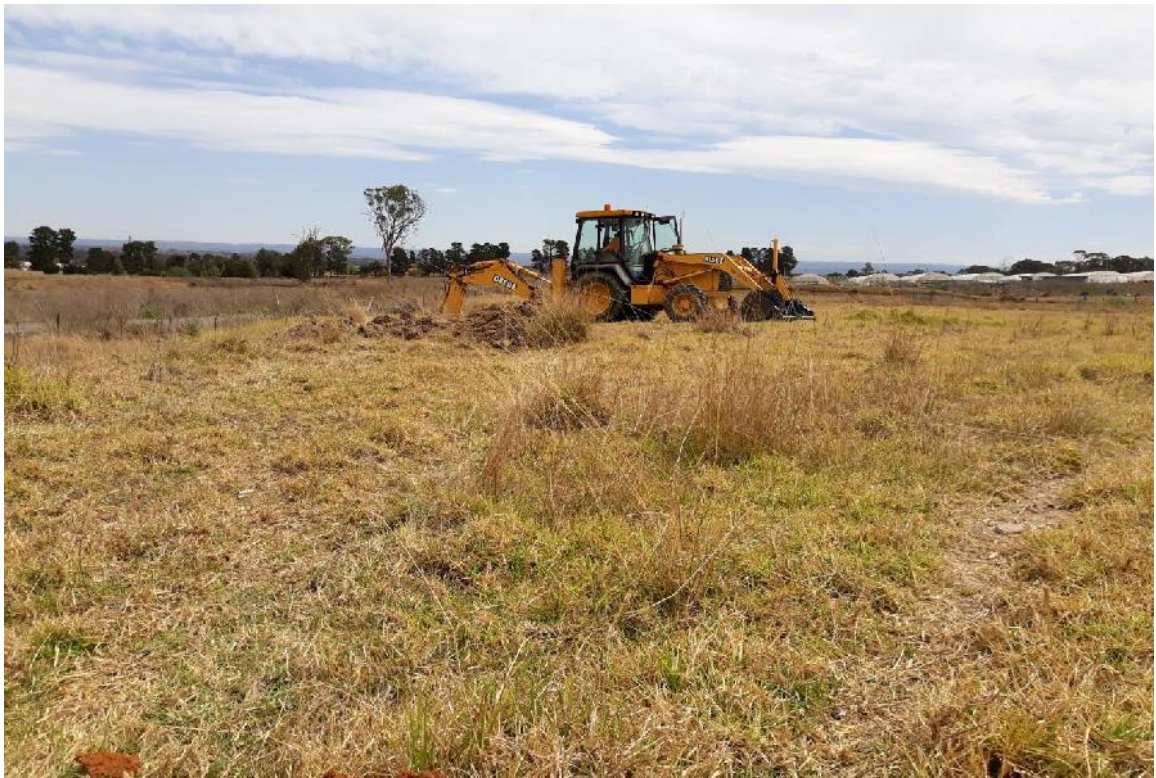
Photo 10 - AEC4J - Area of Fill
