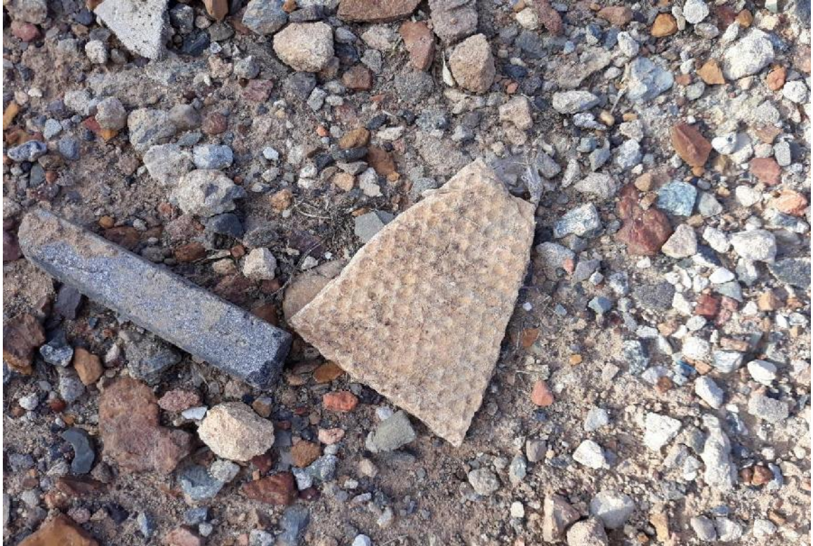
Photo 5 - Suspected ACM Fragment within AEC4C
