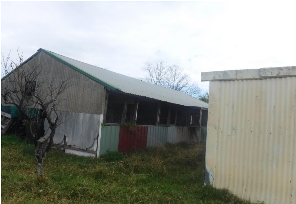
Photo 18: Small sheds in the west of Lot 20 appeared to be partially constructed of ACM (facing west)
