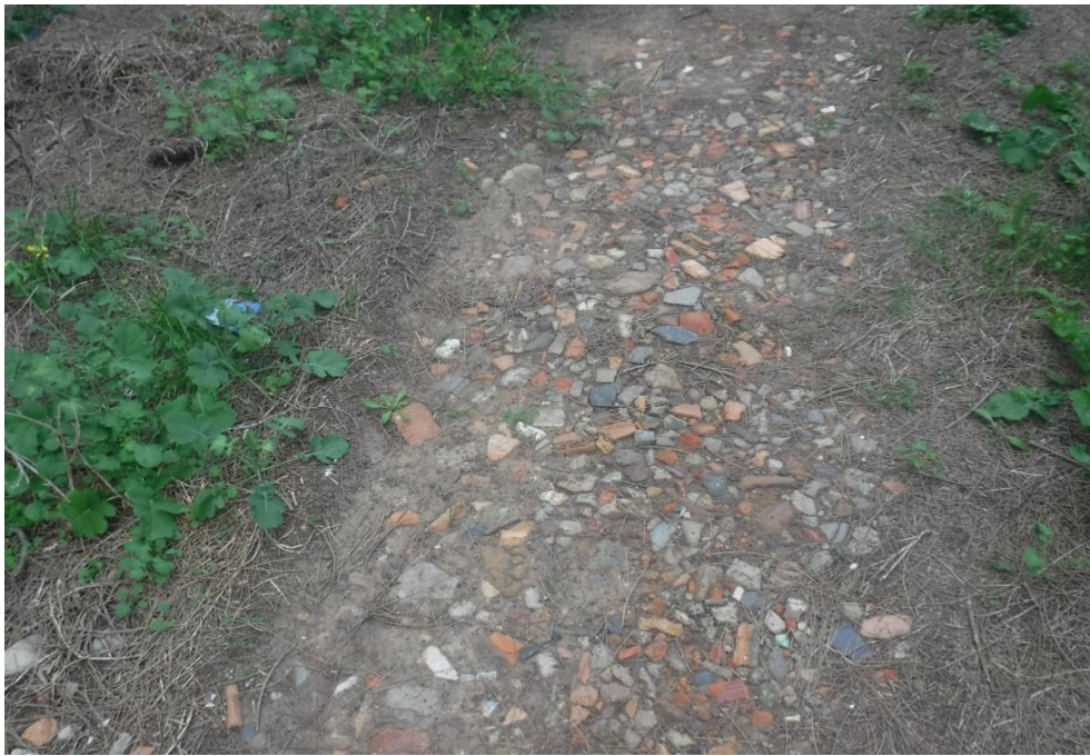
Photo 5: Brick and concrete inclusions were observed in an aggregate driveway in Lot 30
