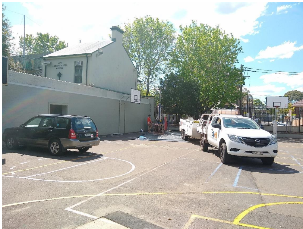
Photo 1 - AG's site investigation – drilling BH02
