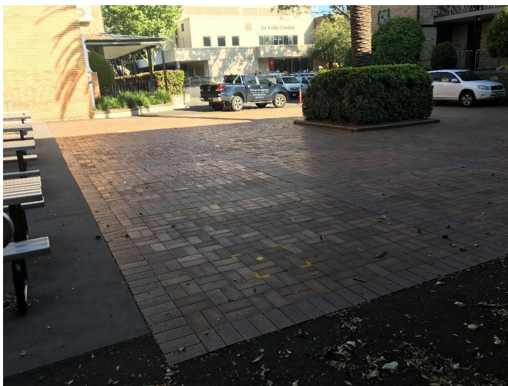
Photo 2 – AG's site investigation – looking south east
