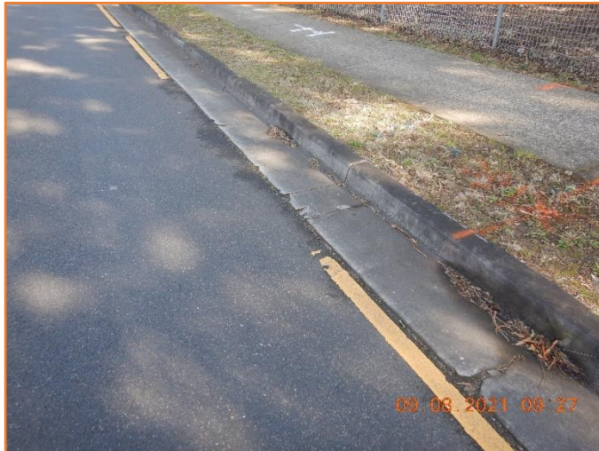
Figure 247: Reasonable - General condition of kerb and gutter.
