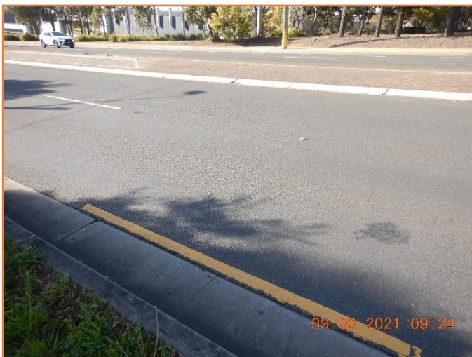
Figure 222: Good - General condition of flexible pavement.
