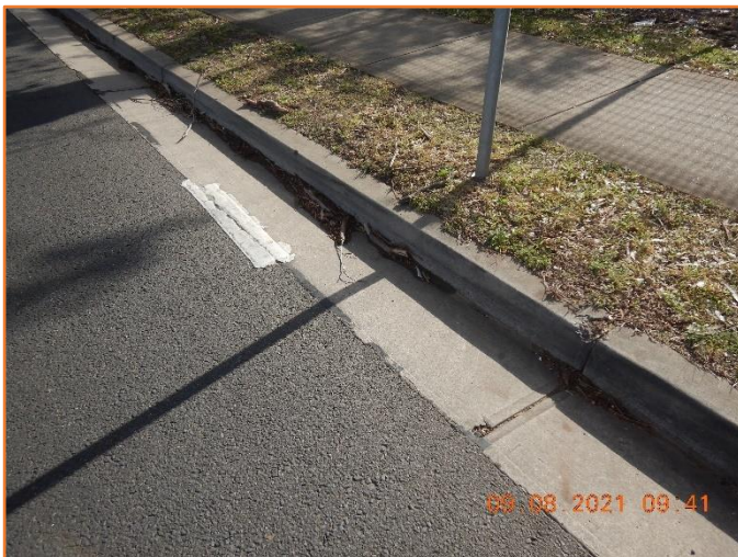
Figure 317: Reasonable - General condition of kerb and gutter. Moderate spalling observed.
