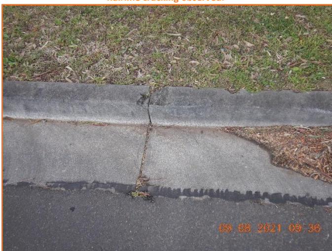
Figure 300: Reasonable - General condition of kerb and gutter. Moderate spalling observed.
