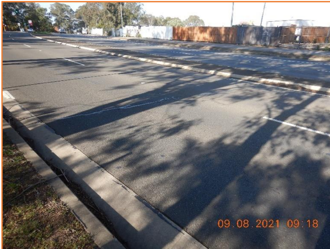
Figure 175: Reasonable - General condition of flexible pavement. Minor previous repair observed.
