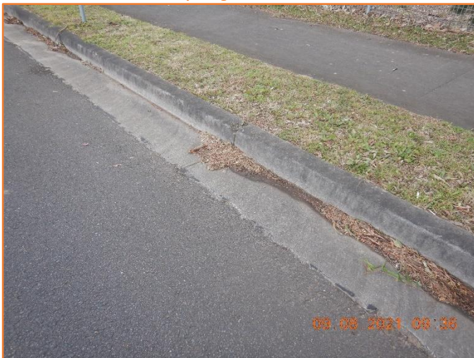
Figure 302: Reasonable - General condition of kerb and gutter.
