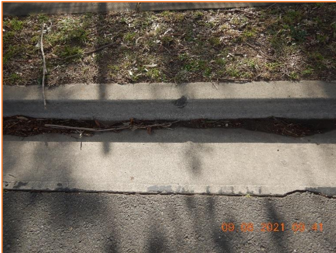
Figure 319: Reasonable - General condition of kerb and gutter. Minor spalling observed.
