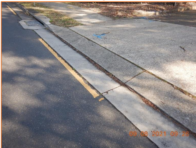
Figure 239: Reasonable - General condition of driveway crossover. Minor hairline cracking observed.
