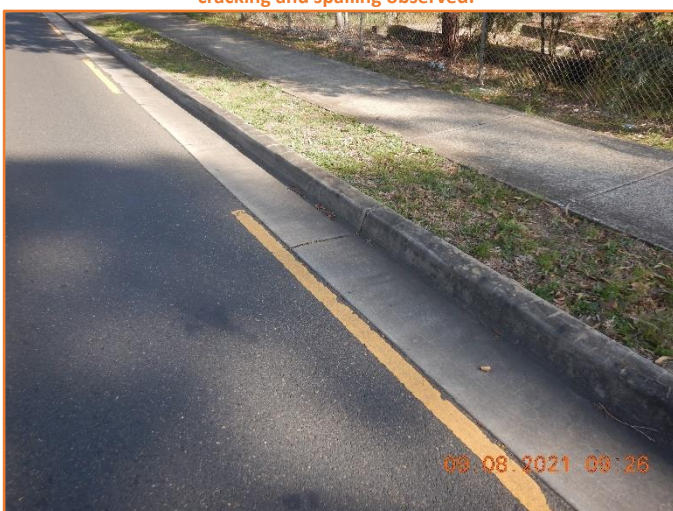
Figure 231: Reasonable - General condition of kerb and gutter.
