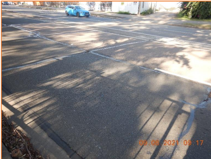
Figure 169: Reasonable - General condition of flexible pavement. Moderate previous repair observed.
