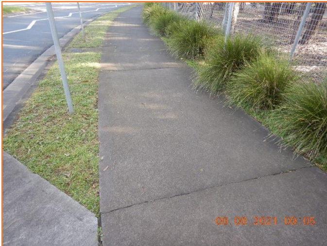
Figure 58: Reasonable - General condition of footpath. Moderate cracking observed.
