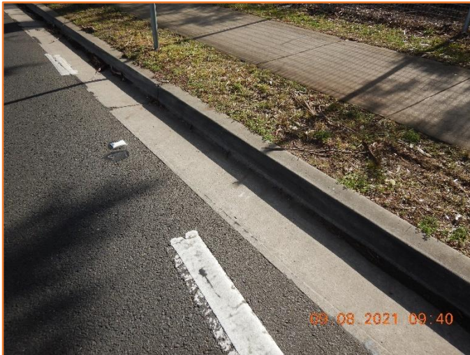
Figure 316: Reasonable - General condition of kerb and gutter.
