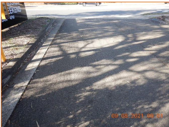
Figure 15: Reasonable - General condition of flexible pavement. Moderate cracking observed.
