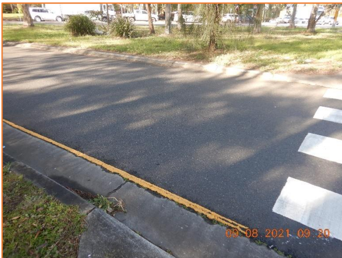
Figure 194: Good - General condition of flexible pavement.
