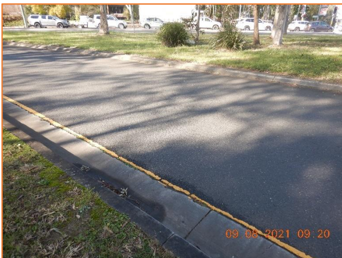
Figure 195: Good - General condition of flexible pavement.
