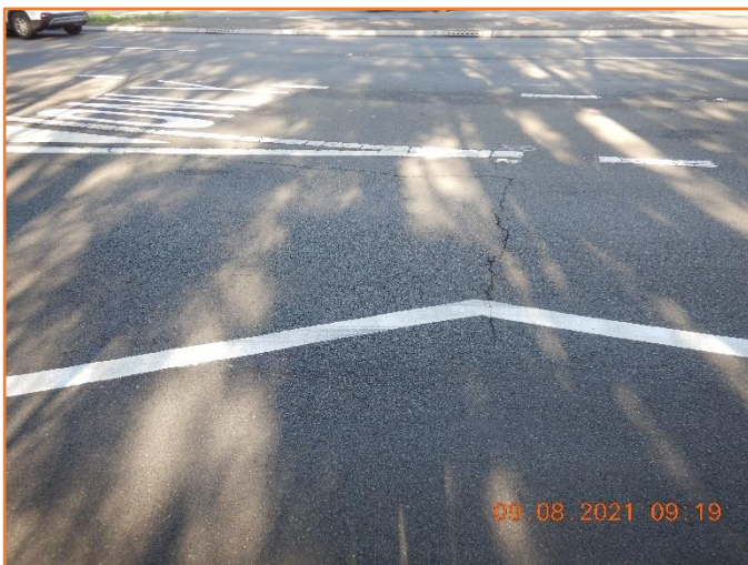
Figure 186: Poor - General condition of flexible pavement. Moderate cracking observed.
