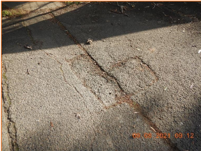
Figure 136: Reasonable - General condition of driveway crossover. Moderate cracking observed.
