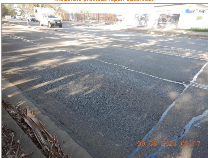
Figure 171: Reasonable - General condition of flexible pavement. Moderate previous repair observed.
