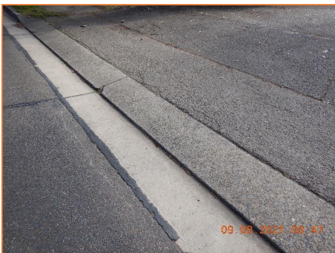
Figure 348: Reasonable - General condition of driveway crossover. Minor cracking observed.
