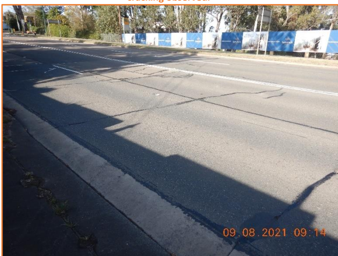
Figure 153: Reasonable - General condition of flexible pavement. Moderate previous repair observed.
