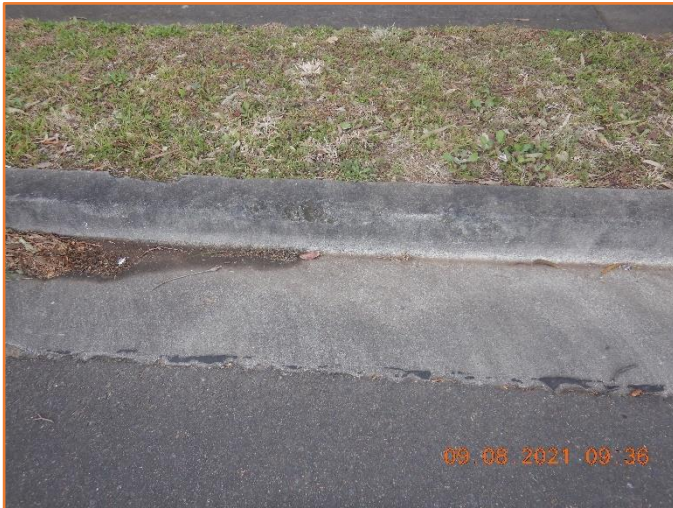
Figure 301: Reasonable - General condition of kerb and gutter. Minor spalling observed.
