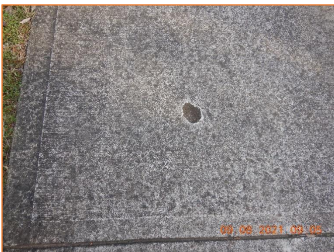
Figure 54: Reasonable - General condition of footpath. Minor physical damage observed.
