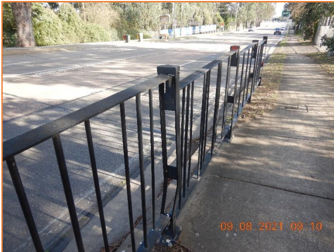
Figure 112: Reasonable - General condition of crash barrier. Moderate physical damage observed.
