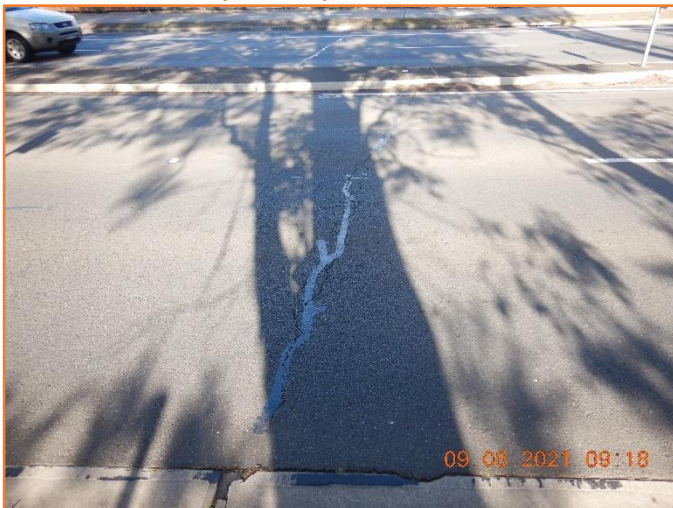
Figure 176: Reasonable - General condition of flexible pavement. Moderate cracking observed.
