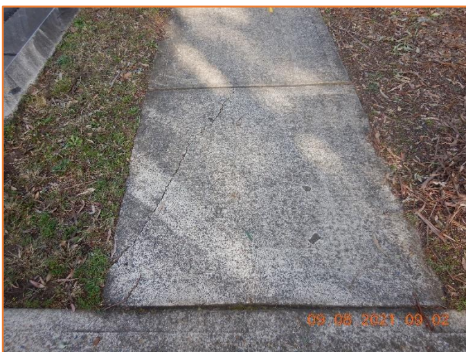
Figure 21: Defective - General condition of footpath. Major cracking and vertical displacement observed.
