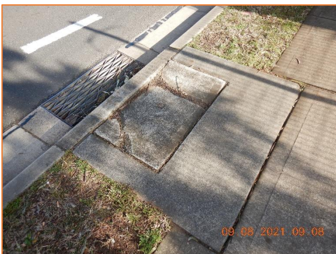
Figure 87: Defective - General condition of kerb inlet pit. Extensive cracking observed.
