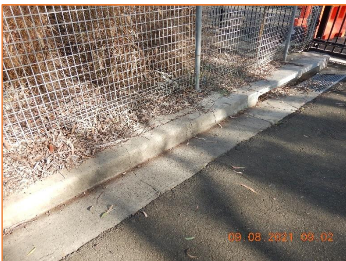
Figure 18: Reasonable - General condition of kerb and gutter. Minor hairline cracking observed.
