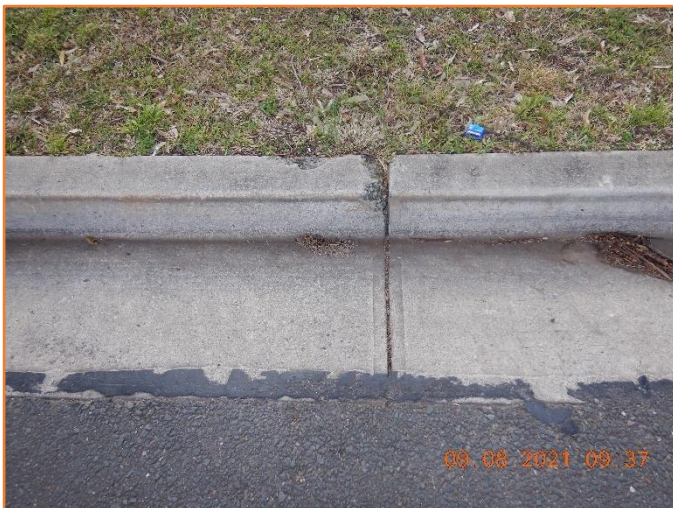
Figure 311: Reasonable - General condition of kerb and gutter. Minor spalling observed.
