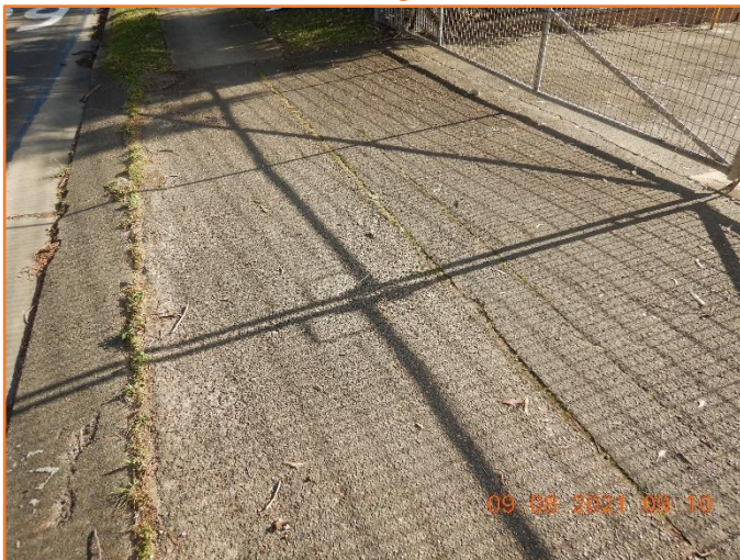
Figure 122: Reasonable - General condition of driveway crossover. Moderate cracking observed.
