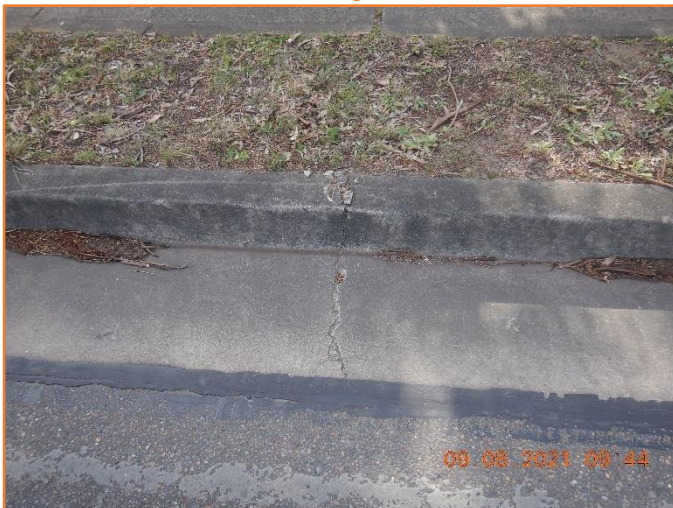
Figure 335: Reasonable - General condition of kerb and gutter. Moderate hairline cracking observed.
