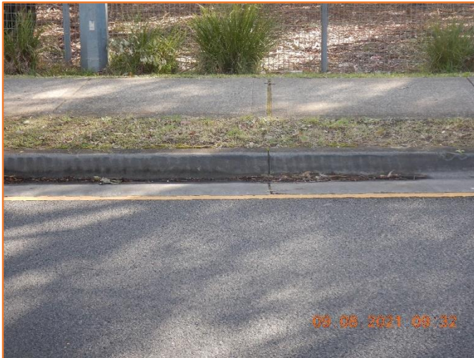
Figure 277: Reasonable - General condition of kerb and gutter.
