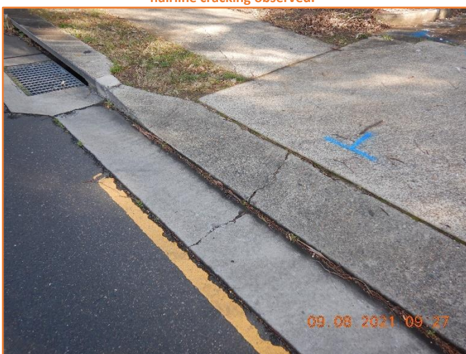
Figure 240: Reasonable - General condition of driveway crossover. Moderate cracking observed.
