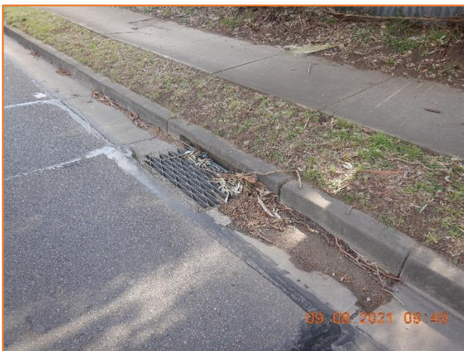
Figure 357: Poor - General condition of kerb inlet pit. Extensive debris build-up observed.
