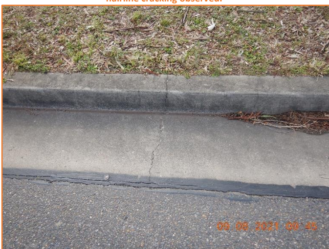
Figure 336: Reasonable - General condition of kerb and gutter. Minor hairline cracking observed.
