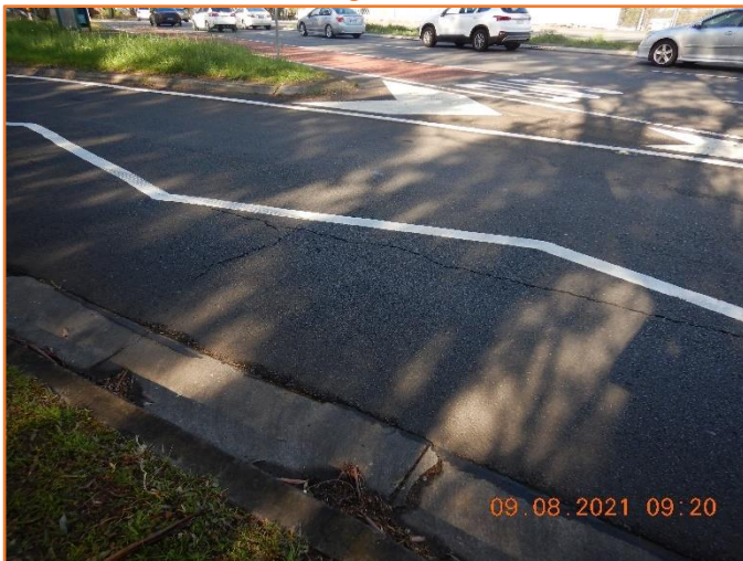
Figure 188: Poor - General condition of flexible pavement. Moderate cracking observed.
