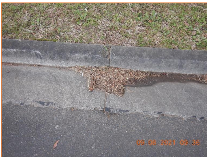
Figure 303: Reasonable - General condition of kerb and gutter. Minor spalling observed.
