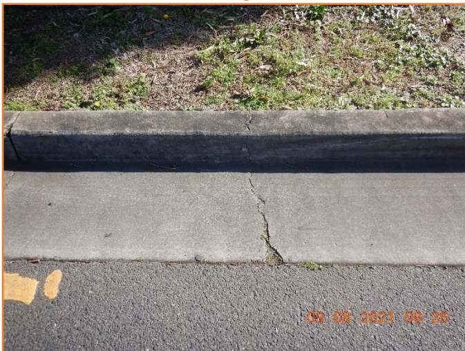
Figure 233: Reasonable - General condition of kerb and gutter. Minor hairline cracking observed.
