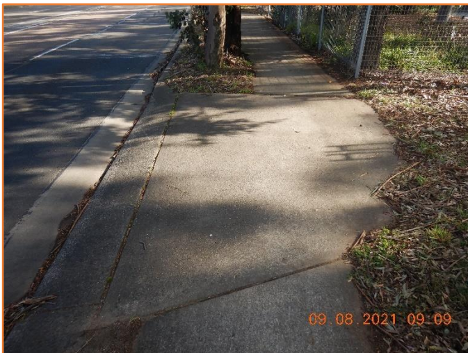
Figure 101: Reasonable - General condition of driveway crossover.
