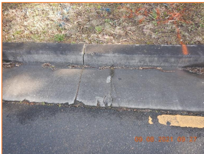
Figure 248: Reasonable - General condition of kerb and gutter. Minor hairline cracking observed.
