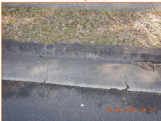
Figure 249: Poor - General condition of kerb and gutter. Moderate cracking and spalling observed.
