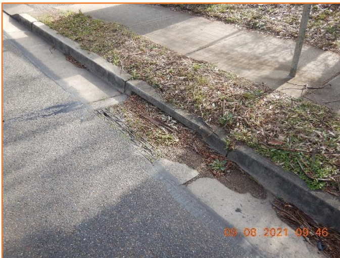
Figure 344: Poor - General condition of kerb inlet pit. Extensive debris build-up observed.
