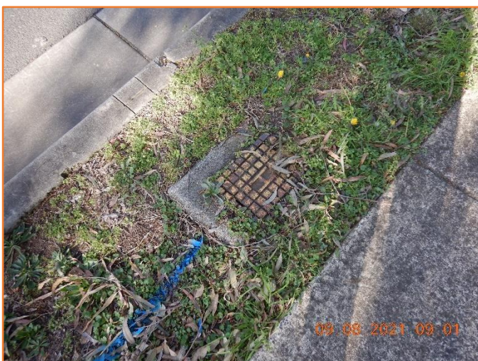
Figure 9: Reasonable - General condition of service pit.
