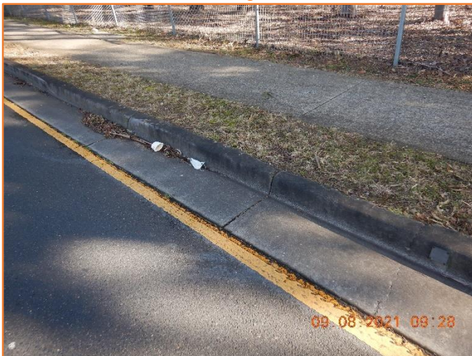
Figure 260: Reasonable - General condition of kerb and gutter. Minor hairline cracking observed.
