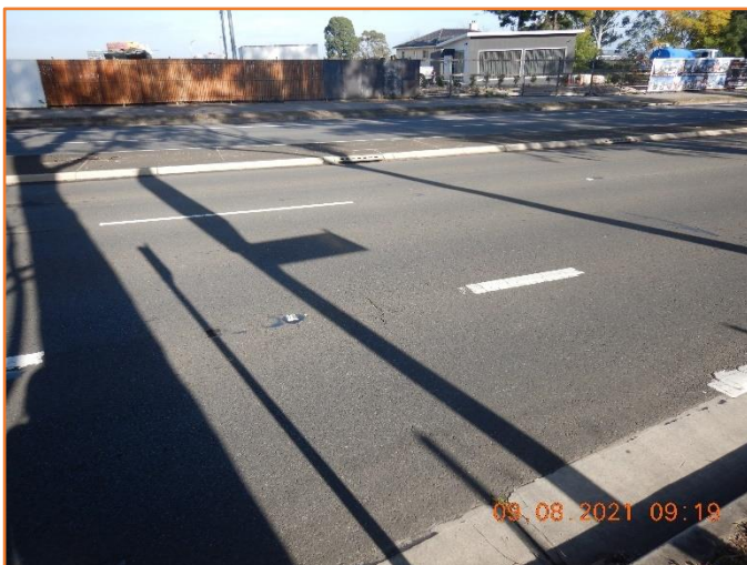
Figure 180: Reasonable - General condition of flexible pavement. Minor cracking observed.
