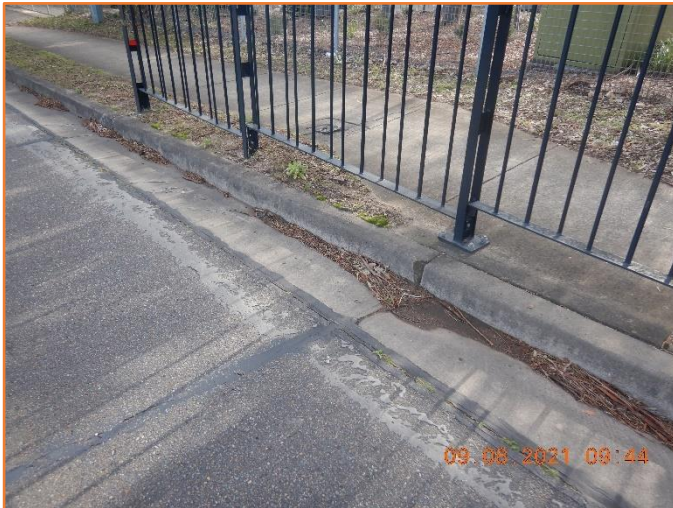
Figure 331: Reasonable - General condition of kerb and gutter.
