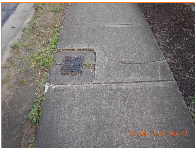
Figure 152: Poor - General condition of footpath and service pit. Moderate cracking observed.
