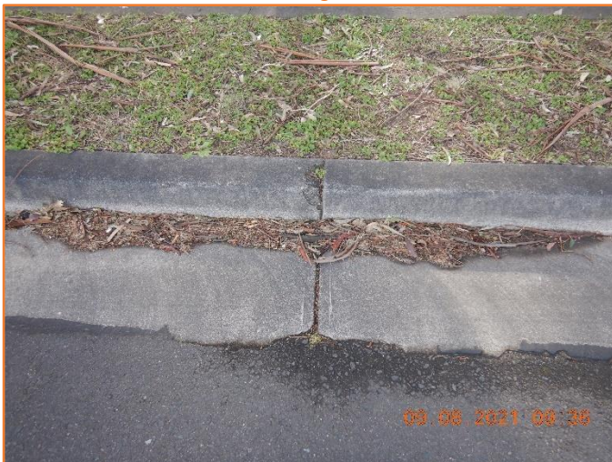
Figure 293: Reasonable - General condition of kerb and gutter. Minor loss of material observed.
