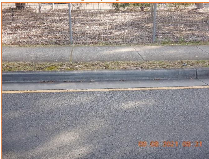
Figure 269: Reasonable - General condition of kerb and gutter.
