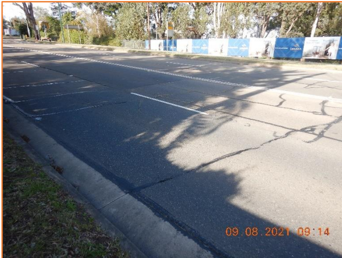
Figure 154: Reasonable - General condition of flexible pavement. Moderate previous repair observed.
