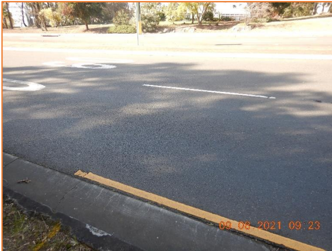
Figure 214: Good - General condition of flexible pavement.
