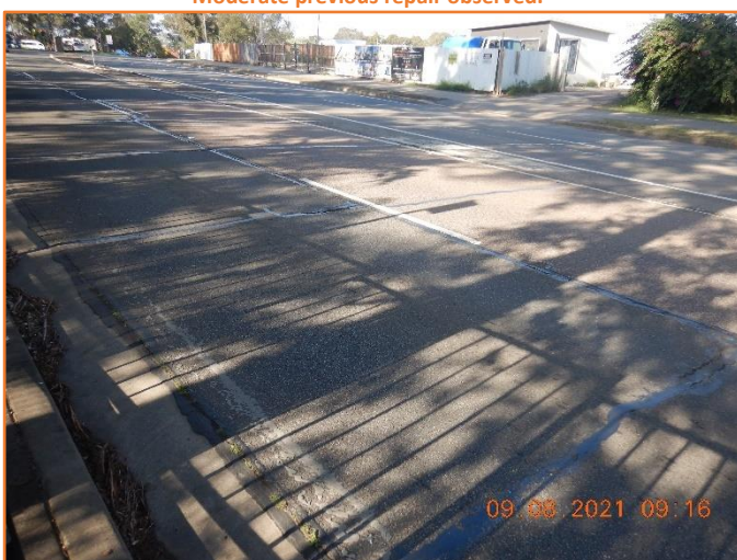
Figure 168: Reasonable - General condition of flexible pavement. Moderate previous repair observed.
