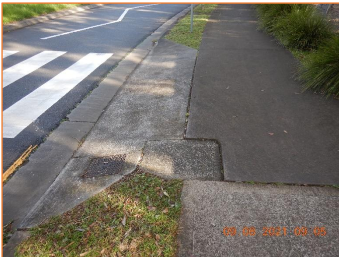
Figure 56: Reasonable - General condition of driveway crossover and service pit. Moderate cracking observed.
