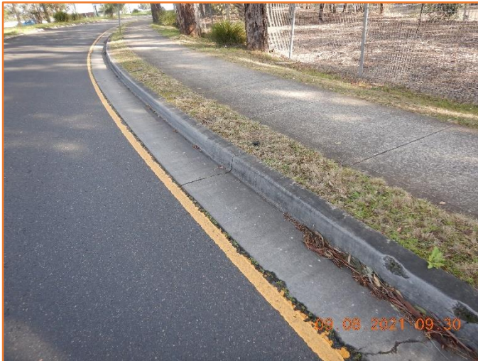
Figure 268: Reasonable - General condition of kerb and gutter. Moderate cracking and spalling observed.
