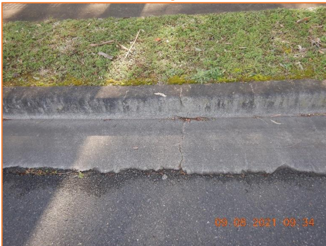
Figure 287: Reasonable - General condition of kerb and gutter. Minor hairline cracking observed.
