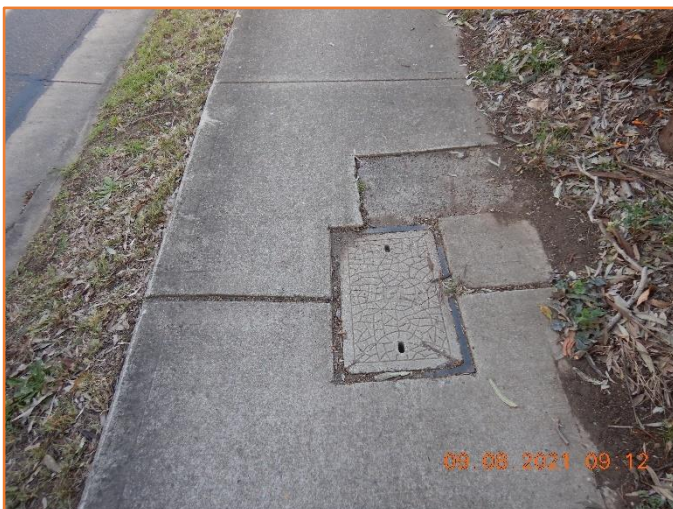
Figure 147: Reasonable - General condition of footpath and service pit.
