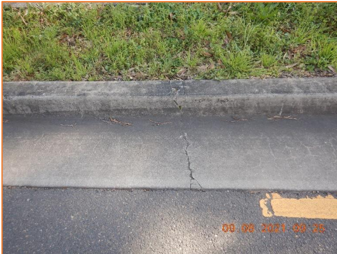
Figure 229: Reasonable - General condition of kerb and gutter. Minor hairline cracking observed.
