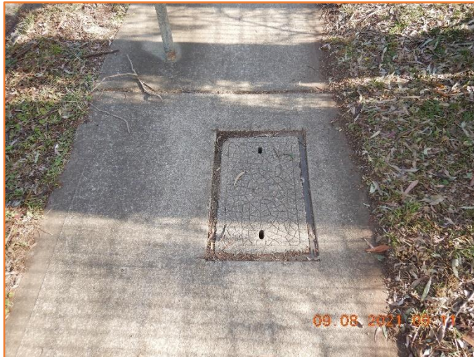
Figure 127: Reasonable - General condition of service pit.
