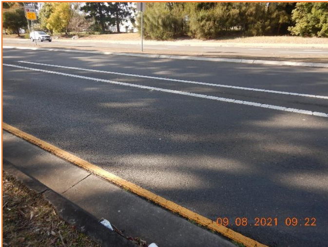
Figure 208: Good - General condition of flexible pavement.
