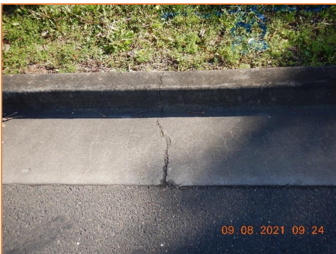
Figure 225: Reasonable - General condition of kerb and gutter. Minor hairline cracking observed.
