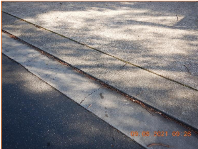
Figure 238: Reasonable - General condition of driveway crossover. Minor hairline cracking observed.
