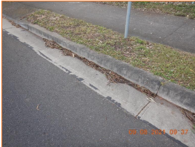
Figure 307: Reasonable - General condition of kerb and gutter.
