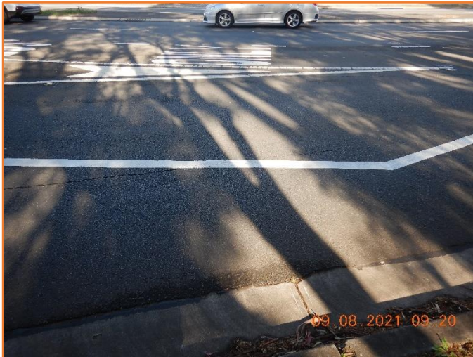
Figure 187: Poor - General condition of flexible pavement. Moderate cracking observed.
