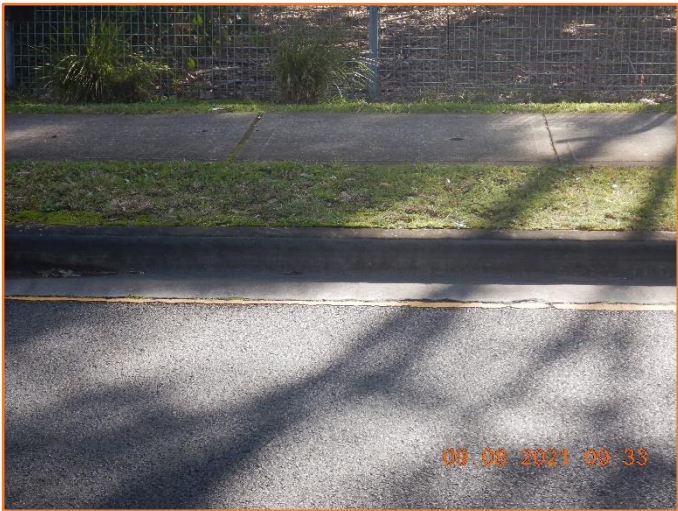
Figure 281: Reasonable - General condition of kerb and gutter.
