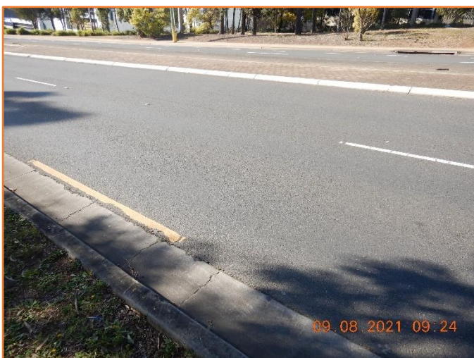
Figure 219: Good - General condition of flexible pavement.
