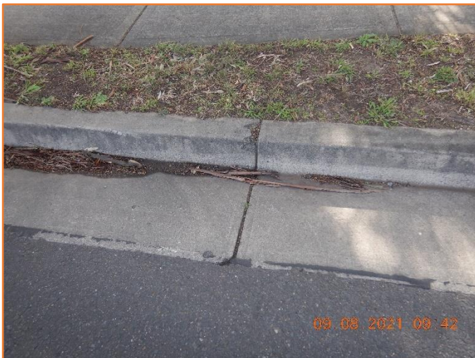
Figure 323: Reasonable - General condition of kerb and gutter. Minor spalling observed.
