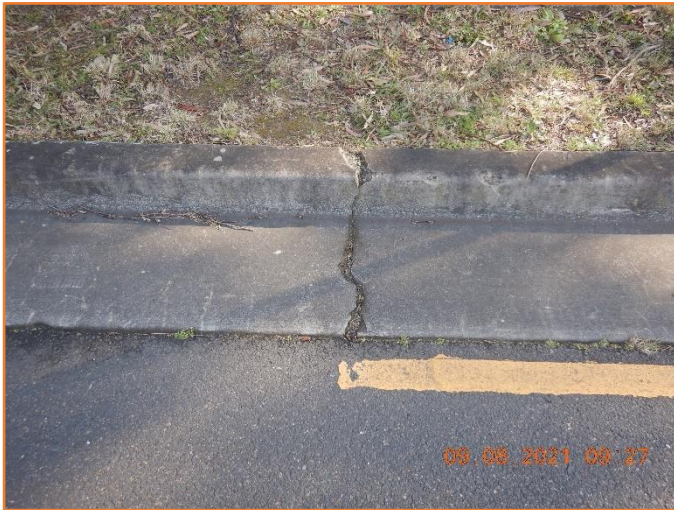
Figure 244: Poor - General condition of kerb and gutter. Moderate cracking and spalling observed.
