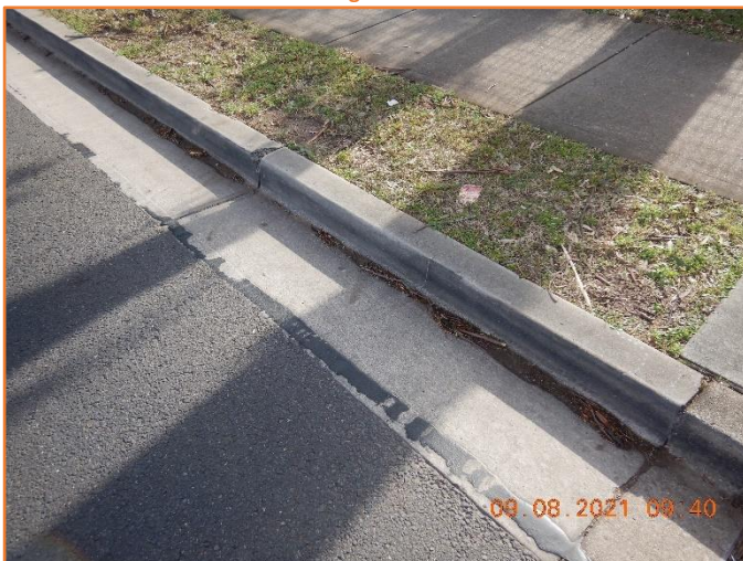
Figure 314: Reasonable - General condition of kerb and gutter. Moderate spalling observed.
