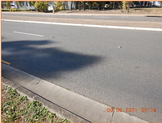
Figure 220: Good - General condition of flexible pavement.
