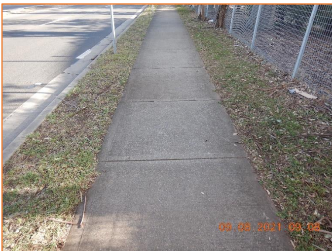
Figure 89: Good - General condition of footpath.
