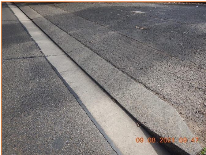
Figure 347: Reasonable - General condition of driveway crossover.
