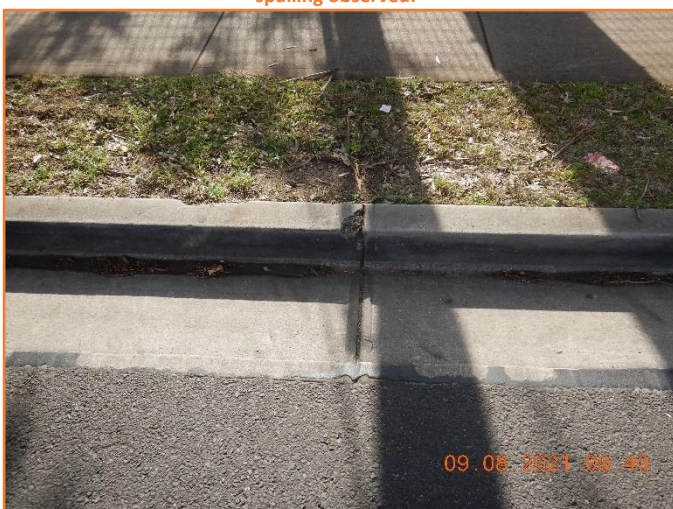
Figure 315: Reasonable - General condition of kerb and gutter. Moderate spalling observed.
