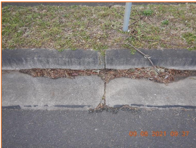
Figure 305: Reasonable - General condition of kerb and gutter. Minor spalling observed.
