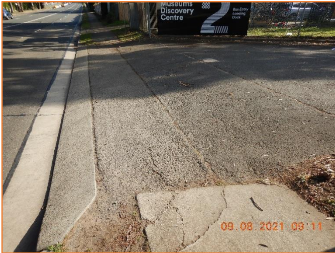
Figure 133: Reasonable - General condition of driveway crossover. Moderate cracking observed.
