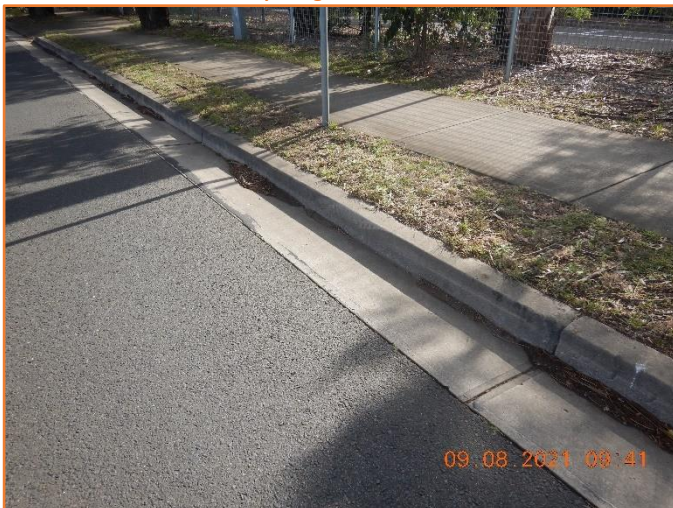
Figure 320: Reasonable - General condition of kerb and gutter.
