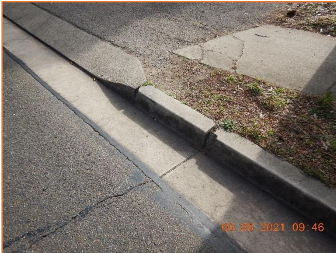
Figure 346: Reasonable - General condition of kerb and gutter and driveway splay. Moderate spalling observed.
