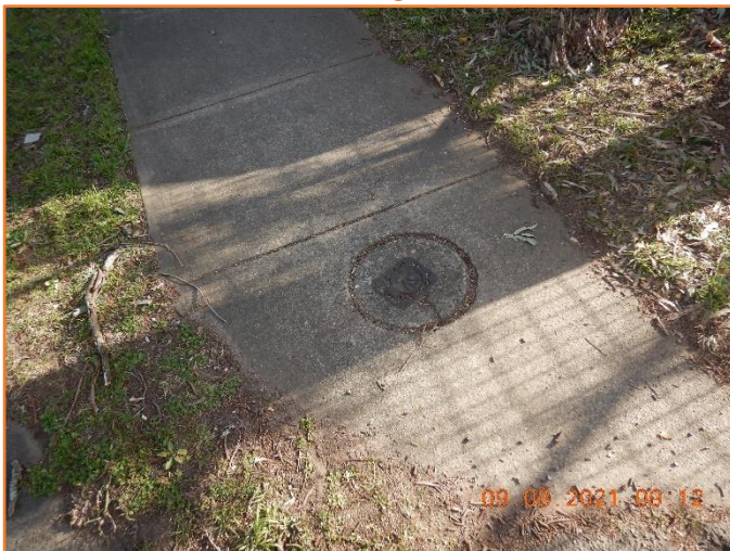
Figure 137: Reasonable - General condition of footpath and service pit.
