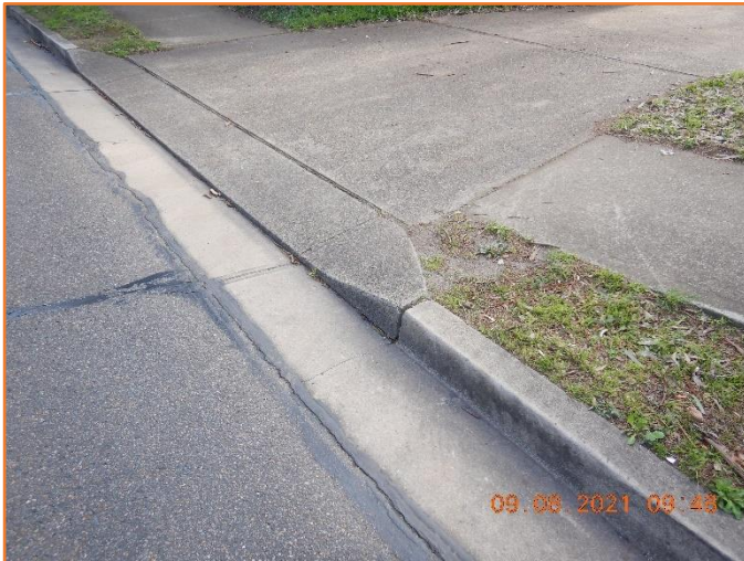
Figure 352: Reasonable - General condition of kerb and gutter and driveway splay. Minor hairline cracking observed.
