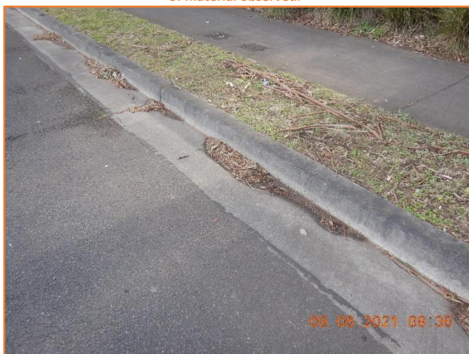
Figure 297: Reasonable - General condition of kerb and gutter.
