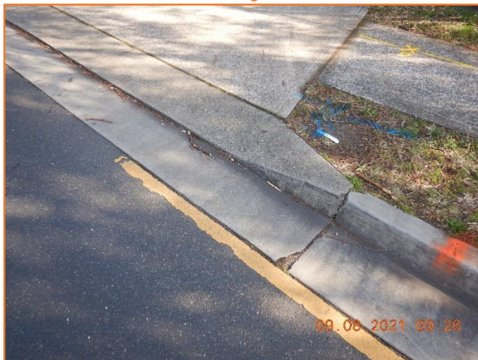
Figure 237: Reasonable - General condition of kerb and gutter and driveway splay. Moderate cracking observed.
