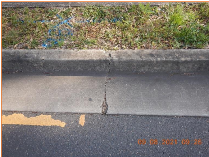
Figure 230: Reasonable - General condition of kerb and gutter. Moderate cracking and spalling observed.
