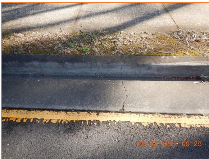
Figure 263: Reasonable - General condition of kerb and gutter. Moderate hairline cracking observed.
