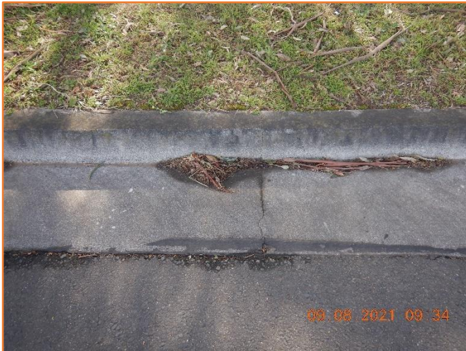
Figure 292: Reasonable - General condition of kerb and gutter. Minor hairline cracking observed.
