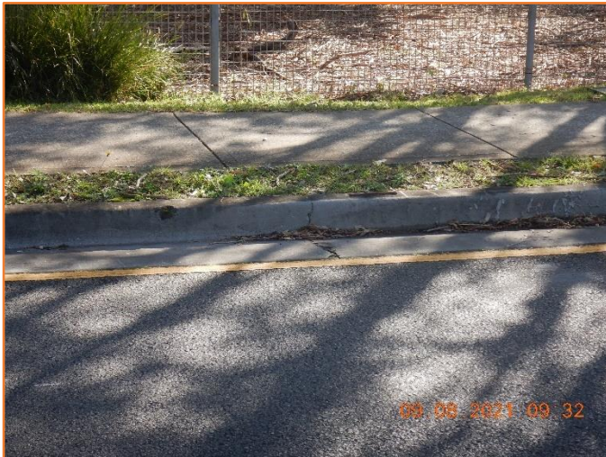
Figure 274: Reasonable - General condition of kerb and gutter. Moderate cracking observed.
