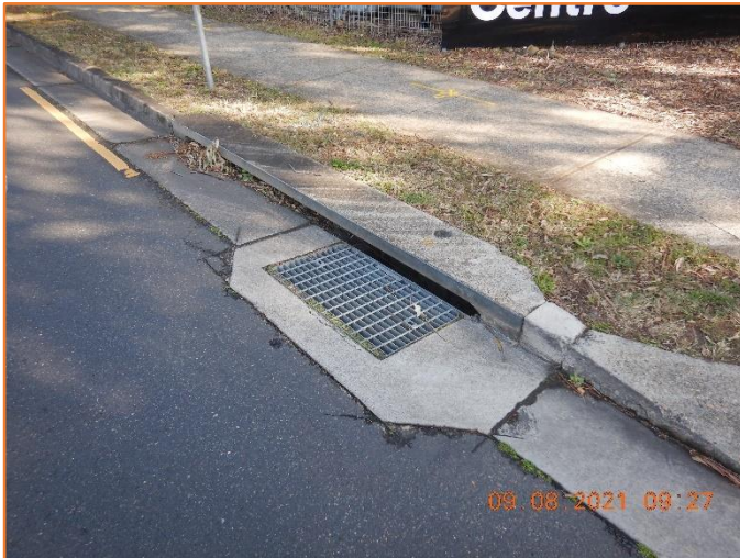
Figure 241: Reasonable - General condition of kerb inlet pit.
