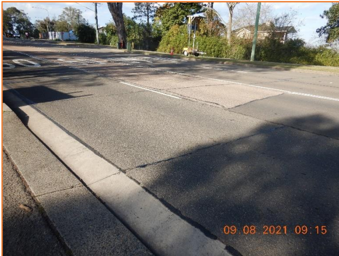
Figure 160: Reasonable - General condition of flexible pavement. Moderate previous repair observed.
