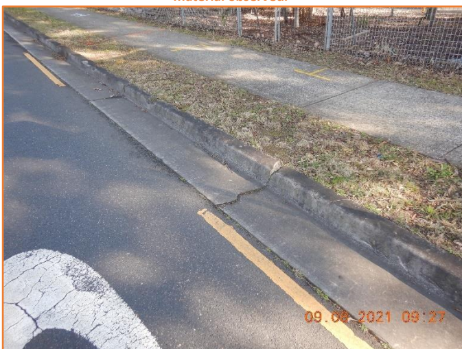
Figure 243: Poor - General condition of kerb and gutter. Moderate cracking and spalling observed.
