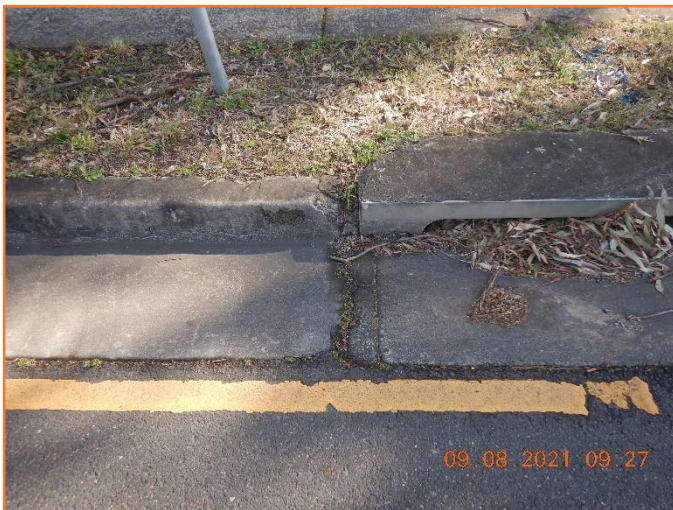
Figure 242: Poor - General condition of kerb and gutter. Moderate loss of material observed.
