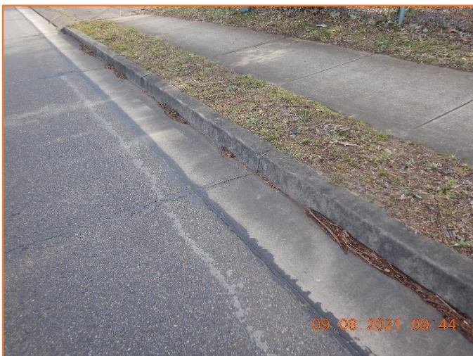
Figure 333: Reasonable - General condition of kerb and gutter.
