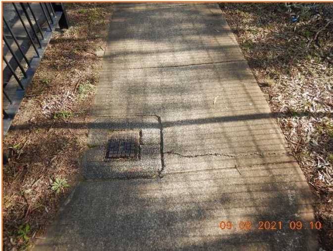
Figure 115: Defective - General condition of footpath and service pit. Major cracking observed.
