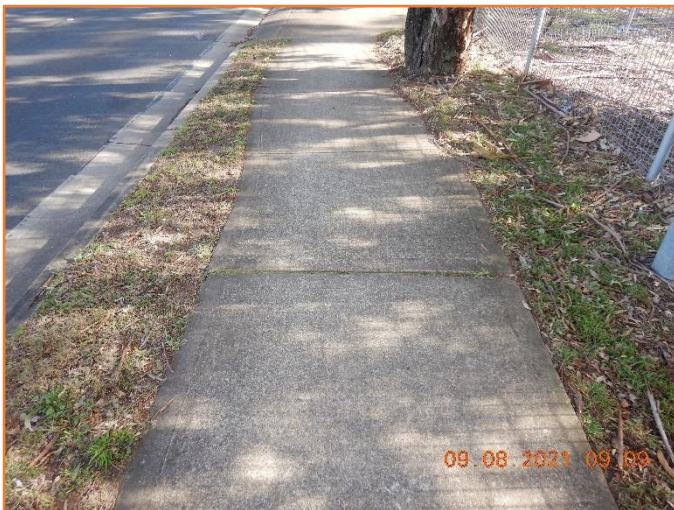
Figure 98: Reasonable - General condition of footpath. Minor differential settlement observed.
