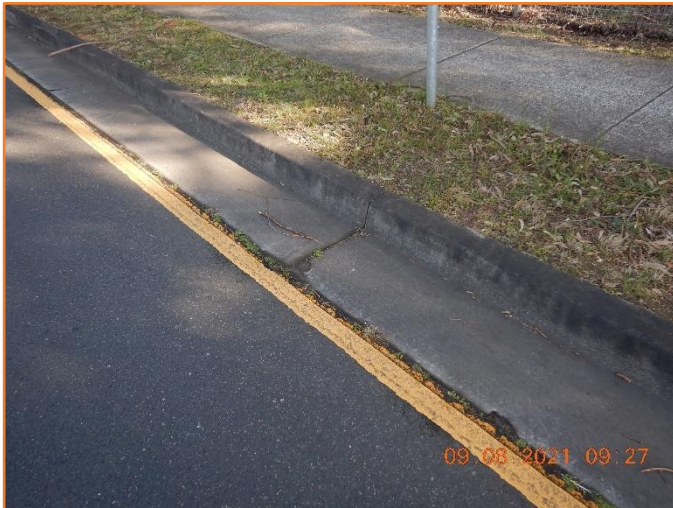
Figure 253: Reasonable - General condition of kerb and gutter.
