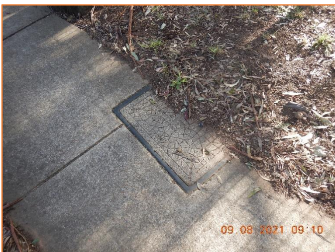
Figure 111: Reasonable - General condition of service pit.
