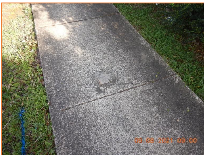
Figure 3: Reasonable - General condition of footpath. Moderate cracking and physical damage observed.
