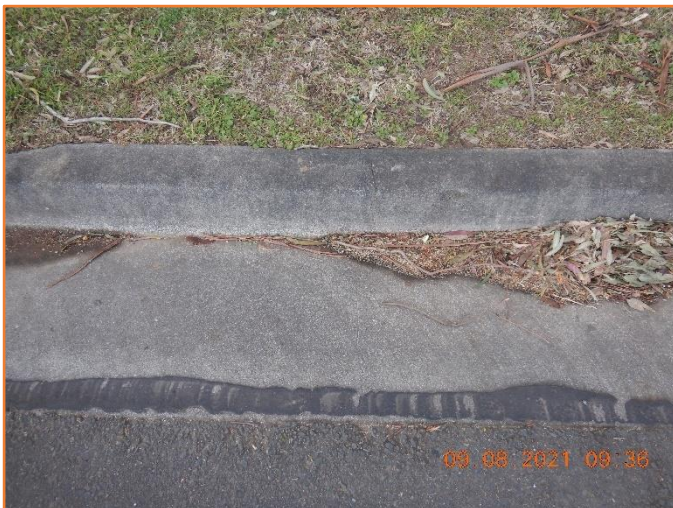
Figure 299: Reasonable - General condition of kerb and gutter. Minor hairline cracking observed.
