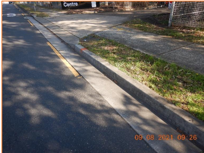
Figure 235: Reasonable - General condition of kerb and gutter.
