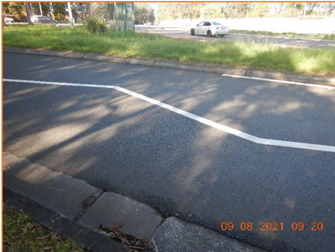
Figure 190: Good - General condition of flexible pavement.
