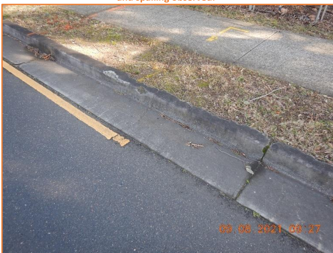
Figure 246: Poor - General condition of kerb and gutter. Moderate cracking and spalling observed.
