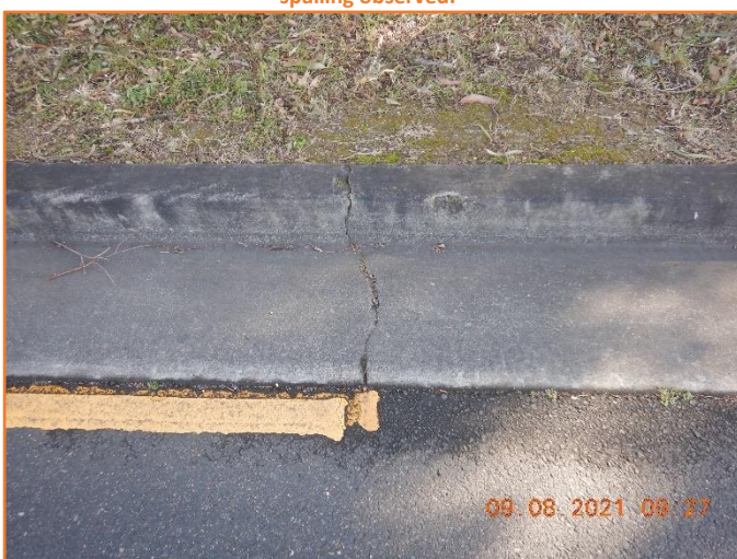
Figure 252: Reasonable - General condition of kerb and gutter. Moderate hairline cracking and spalling observed.
