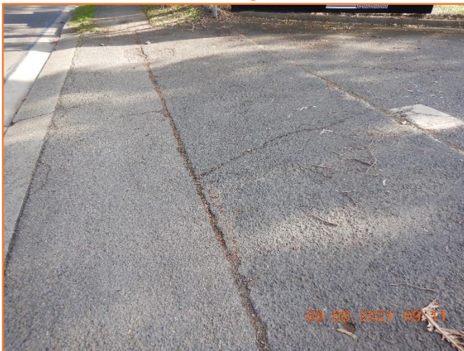
Figure 134: Reasonable - General condition of driveway crossover. Moderate cracking observed.
