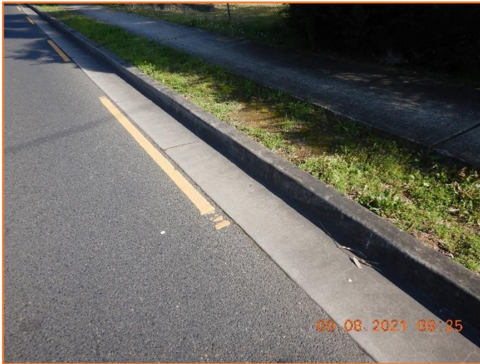
Figure 226: Reasonable - General condition of kerb and gutter.
