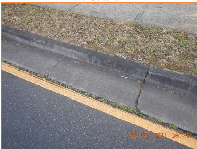
Figure 255: Reasonable - General condition of kerb and gutter. Minor hairline cracking observed.
