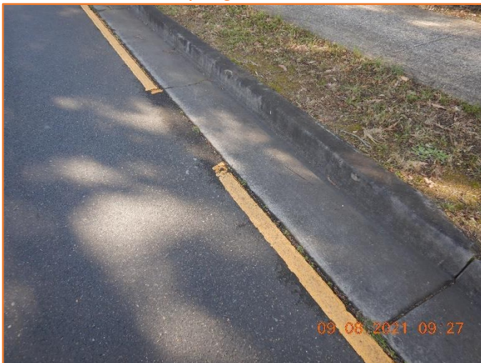
Figure 251: Reasonable - General condition of kerb and gutter. Minor spalling observed.
