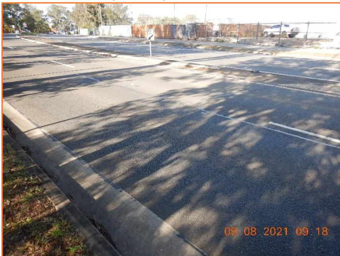
Figure 173: Reasonable - General condition of flexible pavement. Minor previous repair observed.
