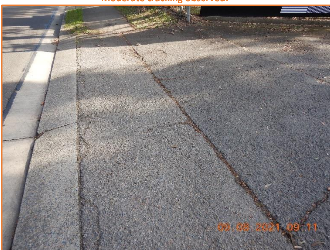
Figure 135: Reasonable - General condition of driveway crossover. Moderate cracking observed.
