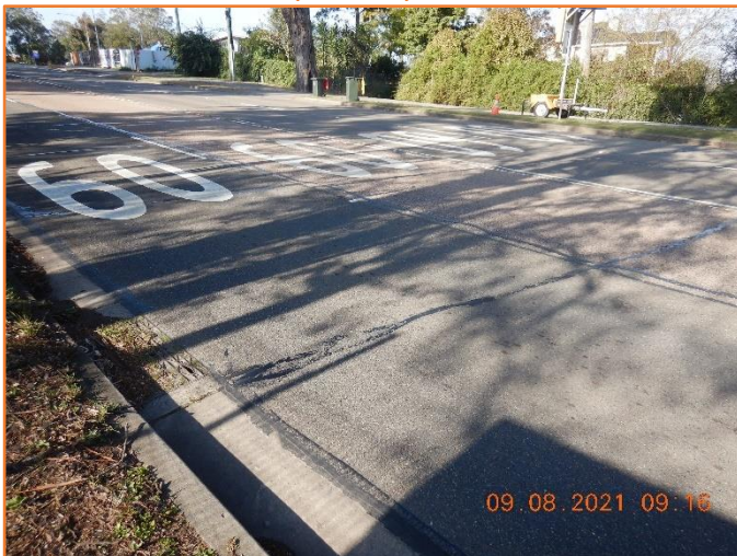
Figure 161: Reasonable - General condition of flexible pavement. Moderate previous repair observed.
