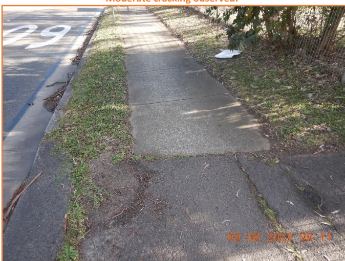
Figure 123: Reasonable - General condition of driveway crossover. Moderate cracking observed.
