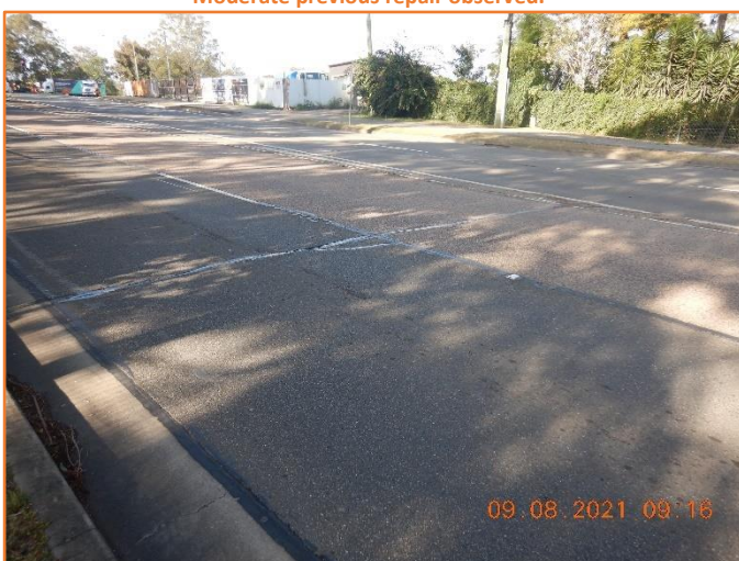
Figure 165: Reasonable - General condition of flexible pavement. Moderate previous repair observed.
