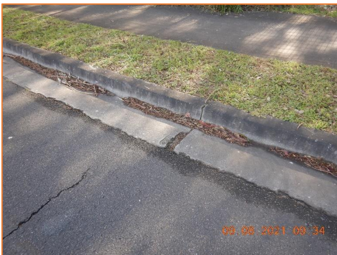
Figure 290: Reasonable - General condition of kerb and gutter. Moderate cracking and loss of material observed.
