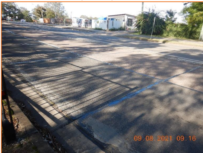
Figure 167: Reasonable - General condition of flexible pavement. Moderate previous repair observed.
