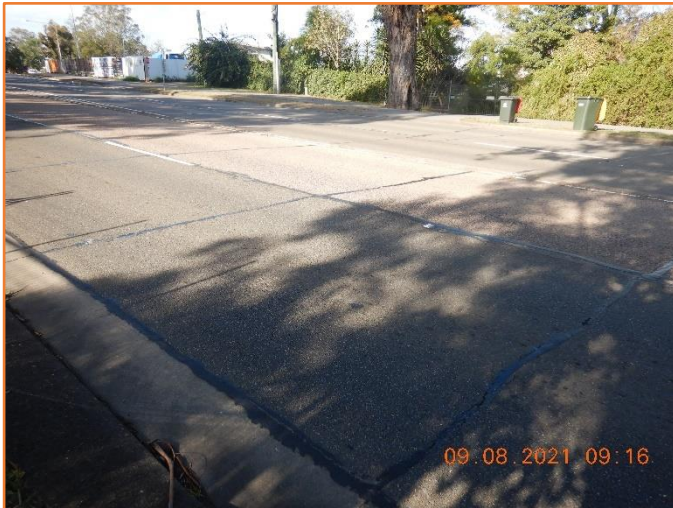
Figure 163: Reasonable - General condition of flexible pavement. Moderate previous repair observed.
