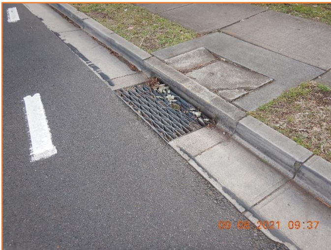
Figure 313: Defective - General condition of kerb inlet pit. Extensive cracking observed.
