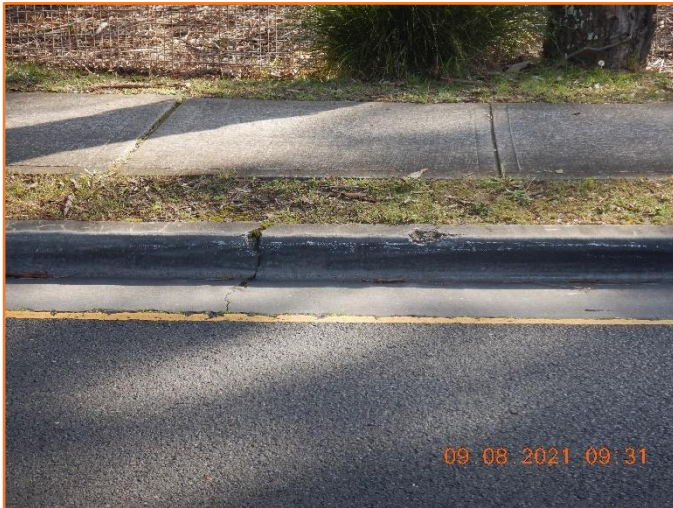
Figure 271: Poor - General condition of kerb and gutter. Moderate cracking and spalling observed.
