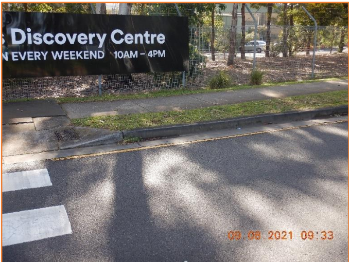
Figure 282: Reasonable - General condition of kerb and gutter and footpath splay. Moderate cracking observed.
