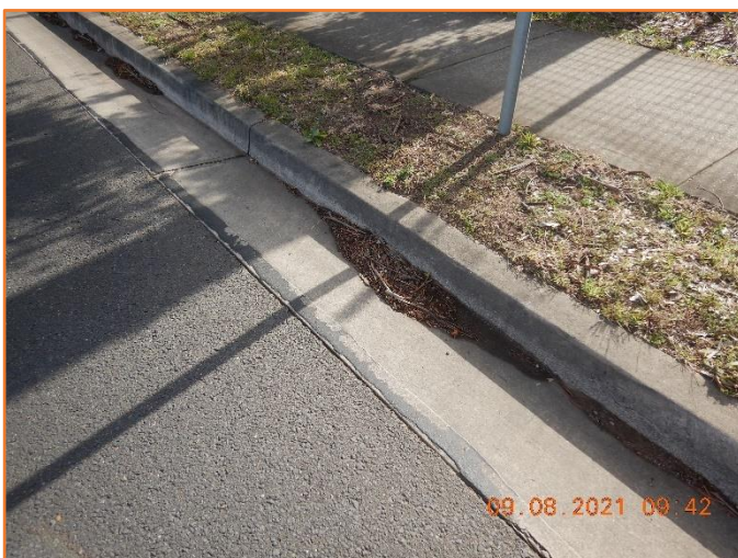
Figure 321: Reasonable - General condition of kerb and gutter.
