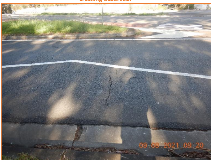
Figure 189: Reasonable - General condition of flexible pavement. Minor cracking observed.
