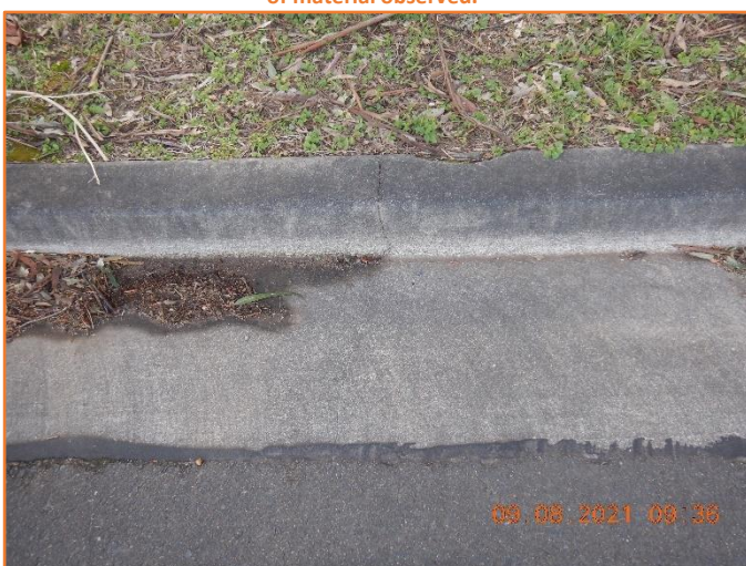
Figure 294: Reasonable - General condition of kerb and gutter. Minor hairline cracking observed.
