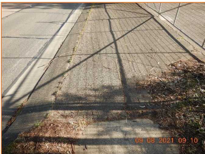
Figure 120: Reasonable - General condition of driveway crossover. Moderate cracking observed.
