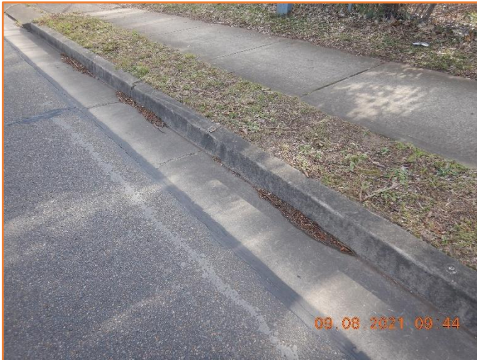
Figure 334: Reasonable - General condition of kerb and gutter. Moderate hairline cracking observed.
