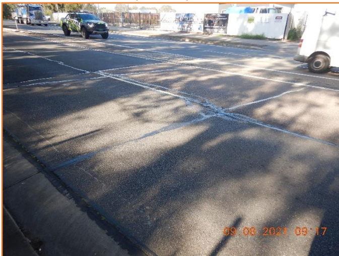
Figure 170: Reasonable - General condition of flexible pavement. Moderate previous repair observed.
