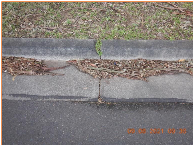
Figure 296: Reasonable - General condition of kerb and gutter. Minor loss of material observed.
