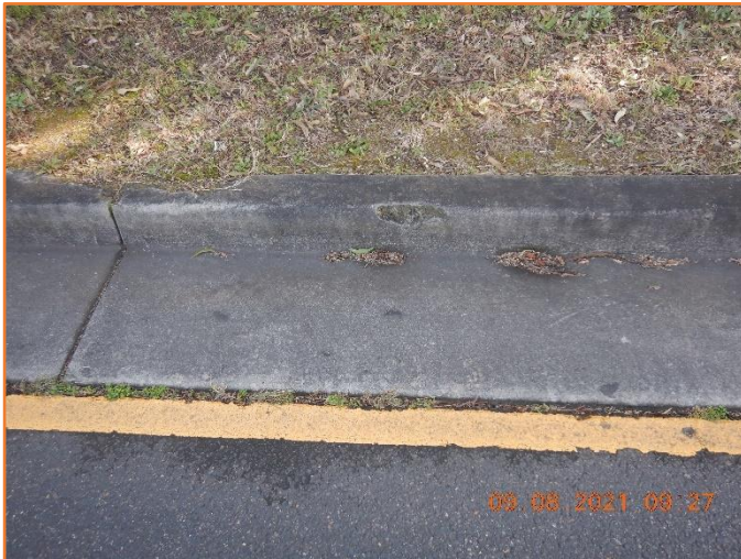
Figure 250: Reasonable - General condition of kerb and gutter. Minor spalling observed.
