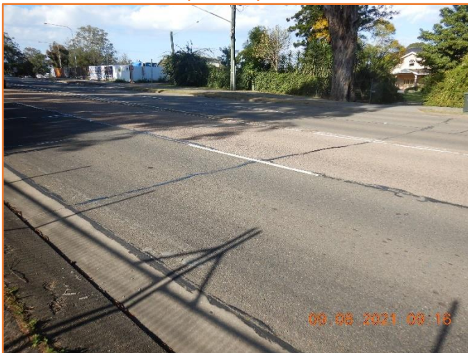
Figure 164: Reasonable - General condition of flexible pavement. Moderate previous repair observed.
