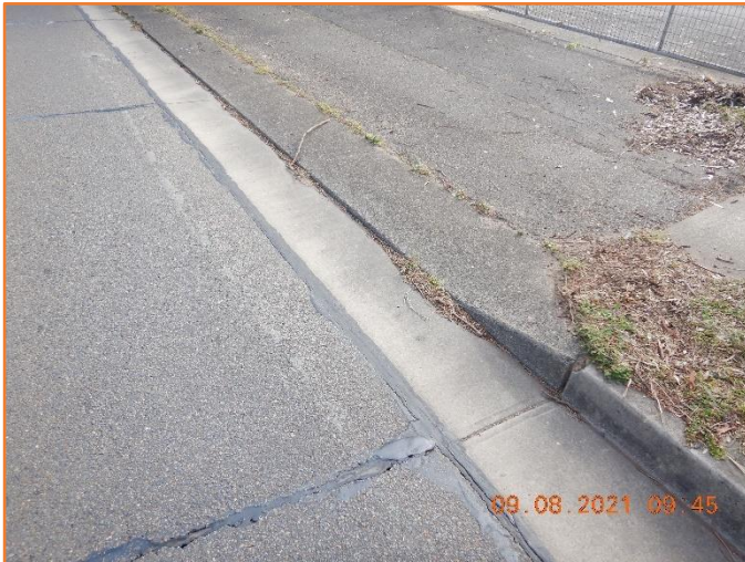
Figure 337: Reasonable - General condition of driveway splay. Minor spalling observed.
