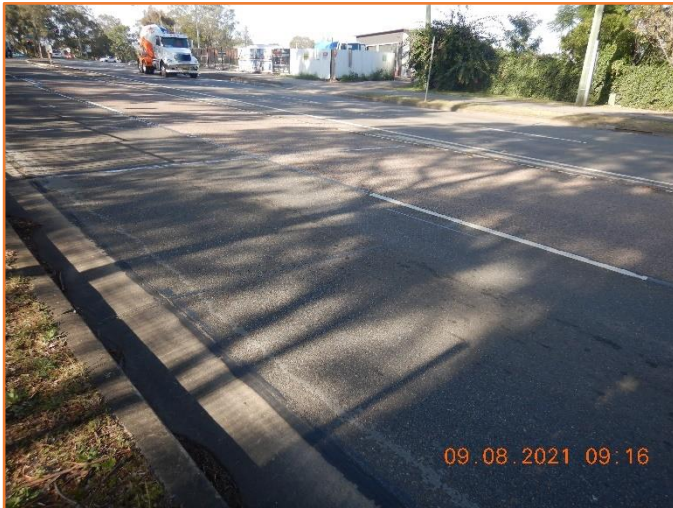
Figure 166: Reasonable - General condition of flexible pavement. Moderate previous repair observed.
