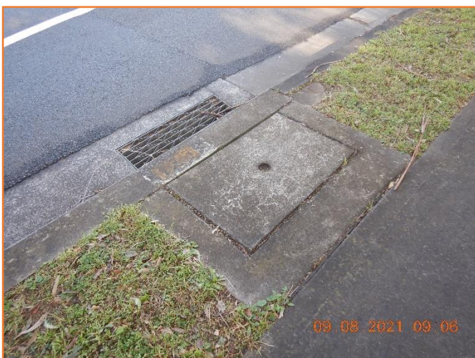
Figure 66: Reasonable - General condition of kerb inlet pit.
