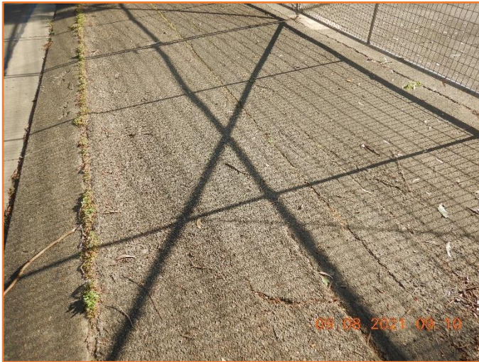
Figure 121: Reasonable - General condition of driveway crossover. Moderate cracking observed.
