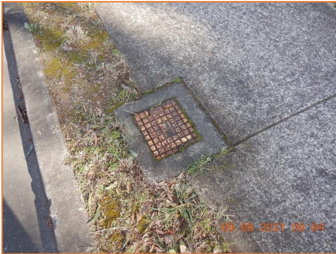
Figure 40: Reasonable - General condition of service pit.
