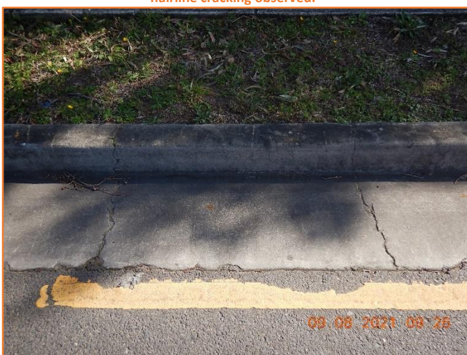
Figure 234: Reasonable - General condition of kerb and gutter. Minor hairline cracking observed.
