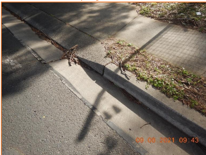
Figure 324: Reasonable - General condition of kerb and gutter and driveway splay.
