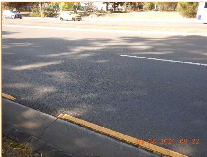
Figure 212: Good - General condition of flexible pavement.
