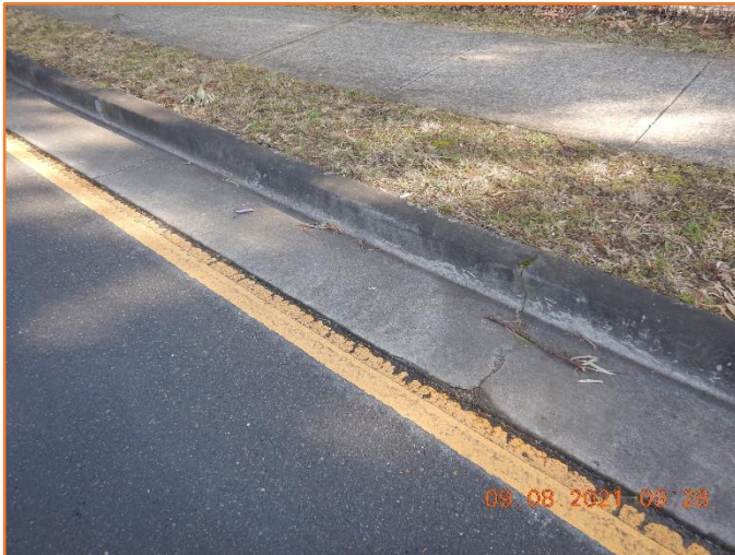
Figure 259: Reasonable - General condition of kerb and gutter. Moderate hairline cracking observed.
