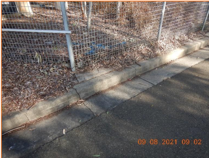
Figure 19: Reasonable - General condition of kerb and gutter. Moderate cracking observed.
