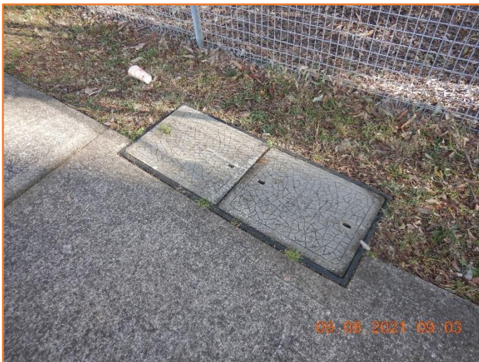
Figure 35: Good - General condition of service pits.
