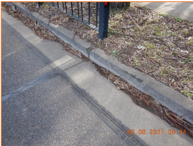
Figure 329: Reasonable - General condition of kerb and gutter. Moderate spalling observed.
