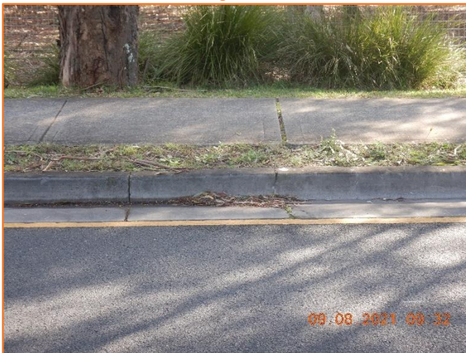
Figure 275: Reasonable - General condition of kerb and gutter. Moderate cracking observed.
