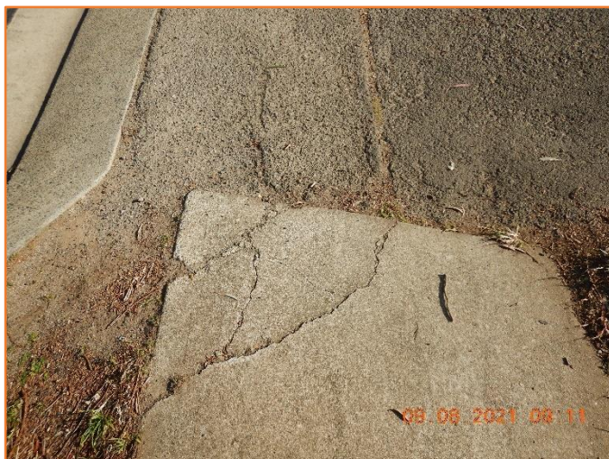
Figure 132: Defective - General condition of footpath. Extensive cracking observed.
