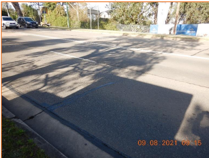
Figure 158: Reasonable - General condition of flexible pavement. Minor previous repair observed.
