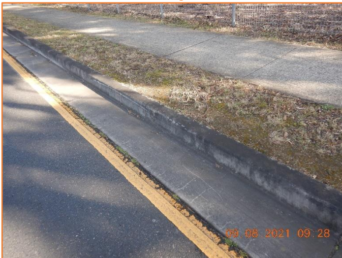
Figure 257: Reasonable - General condition of kerb and gutter. Minor hairline cracking observed.
