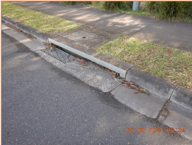
Figure 289: Reasonable - General condition of kerb inlet pit.
