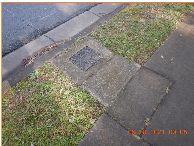
Figure 62: Reasonable - General condition of service pit.
