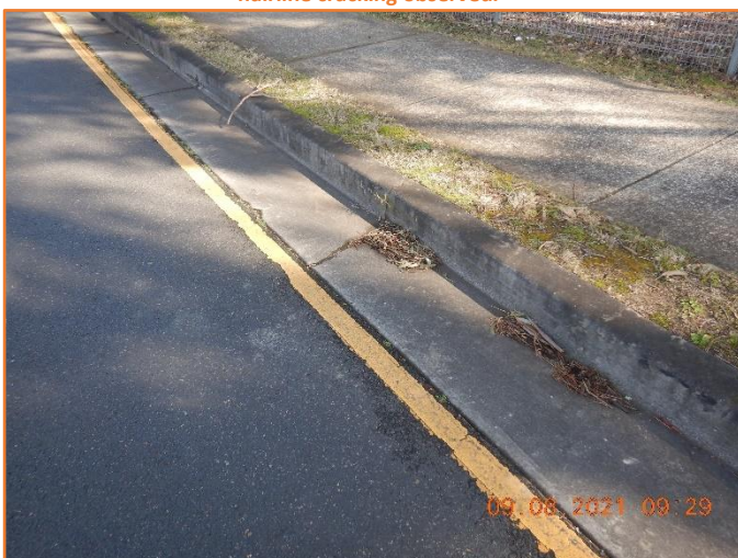
Figure 264: Reasonable - General condition of kerb and gutter. Minor hairline cracking observed.
