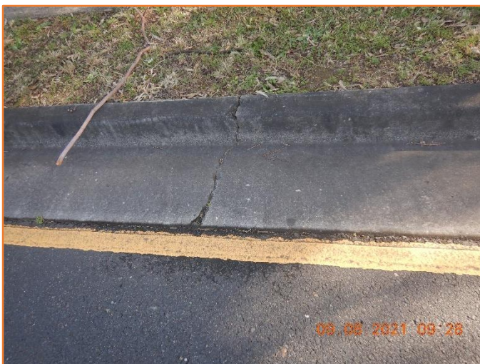
Figure 254: Reasonable - General condition of kerb and gutter. Moderate cracking observed.
