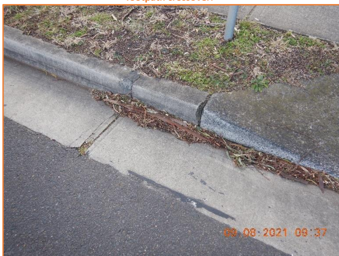
Figure 309: Reasonable - General condition of footpath splay. Moderate cracking observed.
