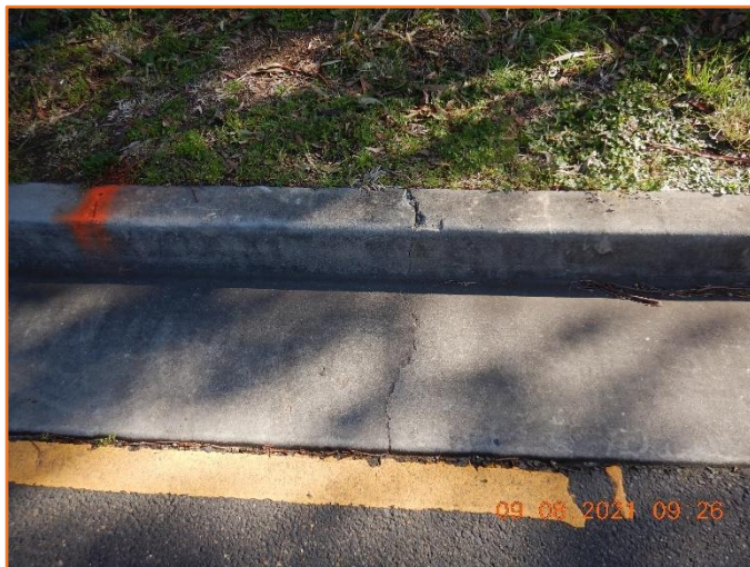
Figure 236: Reasonable - General condition of kerb and gutter. Minor hairline cracking observed.
