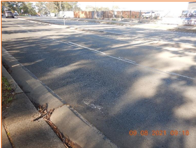
Figure 172: Reasonable - General condition of flexible pavement. Minor previous repair observed.
