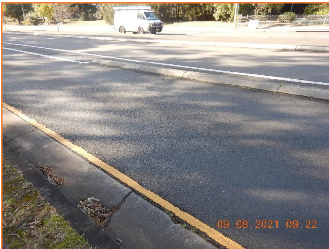
Figure 206: Good - General condition of flexible pavement.
