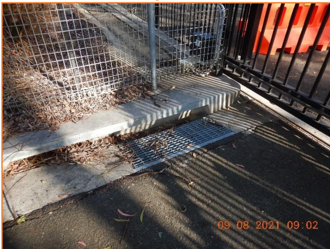
Figure 17: Good - General condition of kerb inlet pit.
