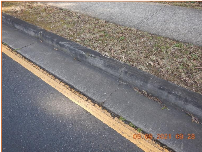
Figure 256: Reasonable - General condition of kerb and gutter. Minor hairline cracking observed.
