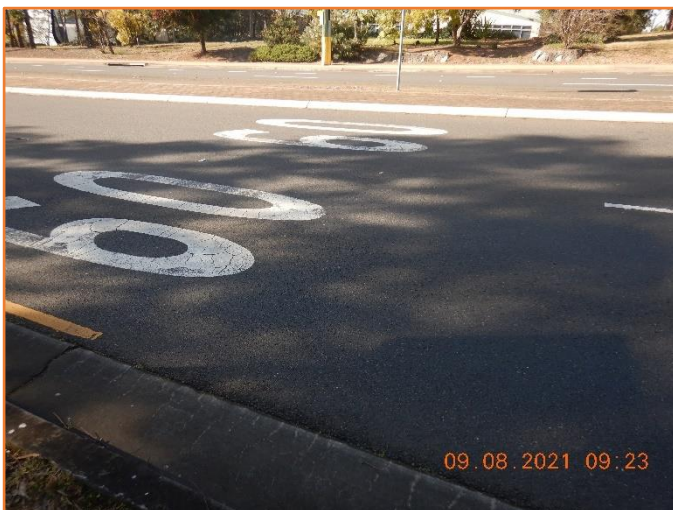
Figure 215: Good - General condition of flexible pavement.
