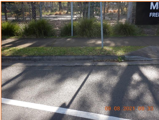
Figure 284: Reasonable - General condition of kerb and gutter and footpath splay.
