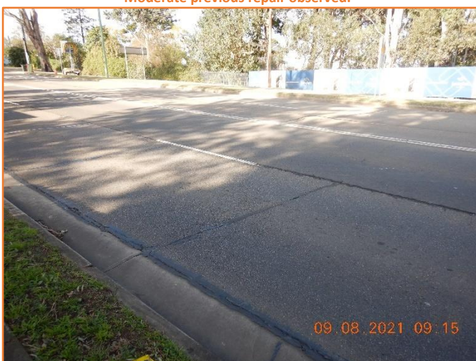
Figure 156: Reasonable - General condition of flexible pavement. Moderate previous repair observed.
