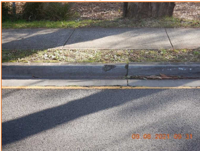
Figure 272: Reasonable - General condition of kerb and gutter. Moderate spalling observed.
