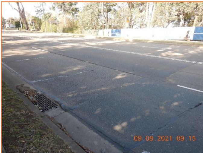
Figure 155: Reasonable - General condition of flexible pavement. Moderate previous repair observed.
