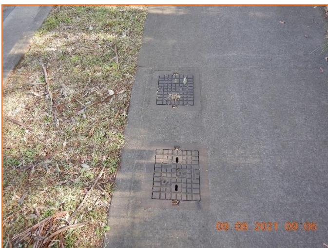
Figure 72: Good - General condition of service pits.
