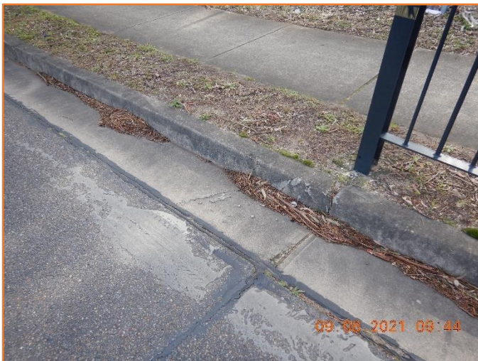
Figure 332: Reasonable - General condition of kerb and gutter.
