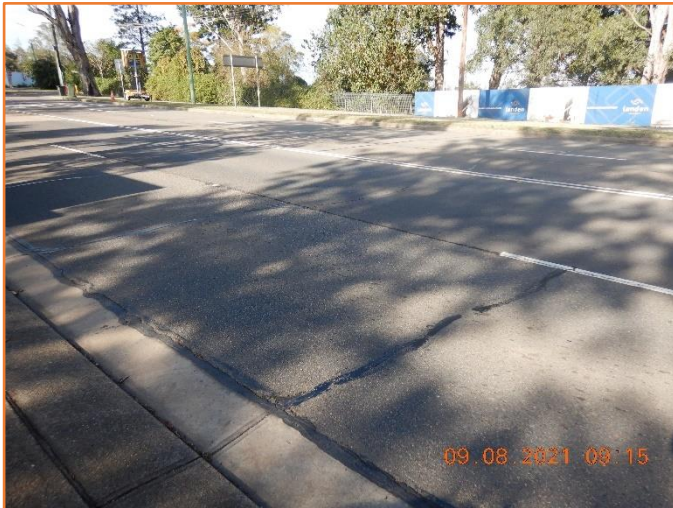
Figure 157: Reasonable - General condition of flexible pavement. Moderate previous repair observed.
