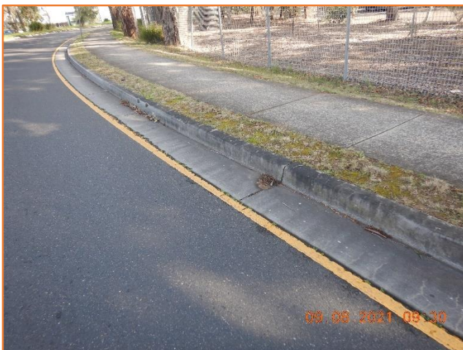
Figure 267: Reasonable - General condition of kerb and gutter.
