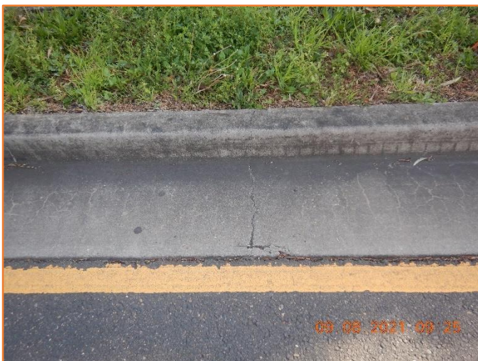
Figure 228: Reasonable - General condition of kerb and gutter. Minor hairline cracking observed.
