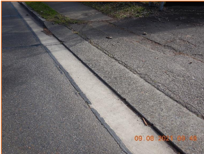
Figure 349: Reasonable - General condition of driveway crossover. Moderate cracking observed.
