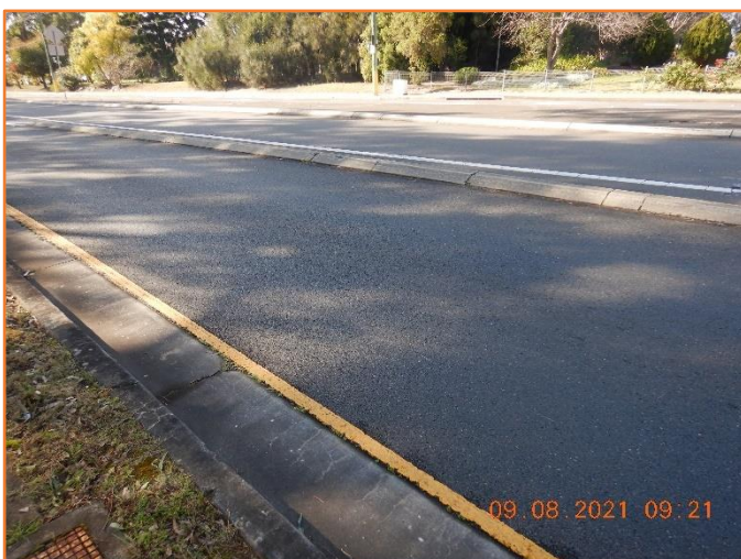
Figure 204: Good - General condition of flexible pavement.
