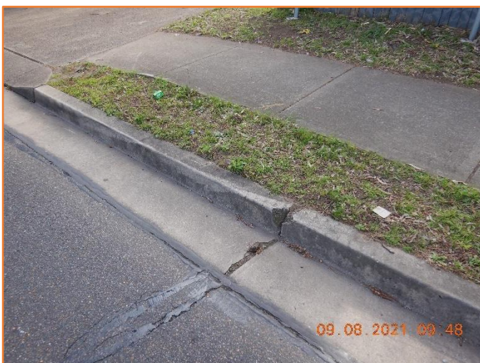
Figure 351: Poor - General condition of kerb and gutter. Major spalling observed.
