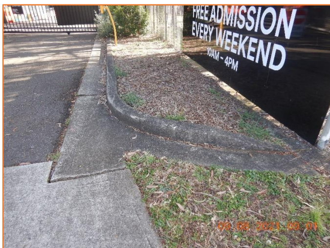
Figure 12: Reasonable - General condition of kerb and gutter.
