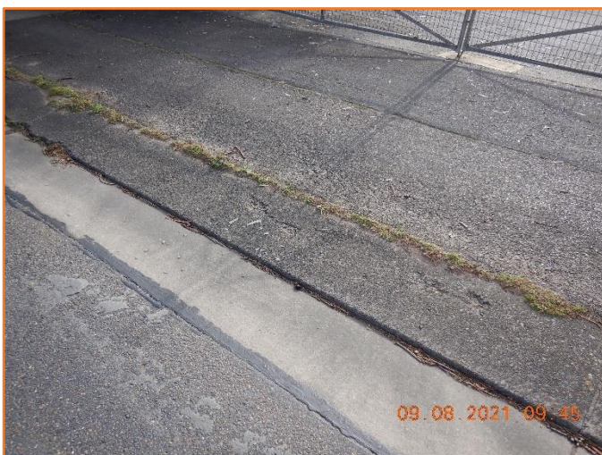
Figure 339: Reasonable - General condition of driveway crossover. Moderate cracking observed.
