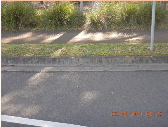
Figure 286: Reasonable - General condition of kerb and gutter. Minor hairline cracking observed.
