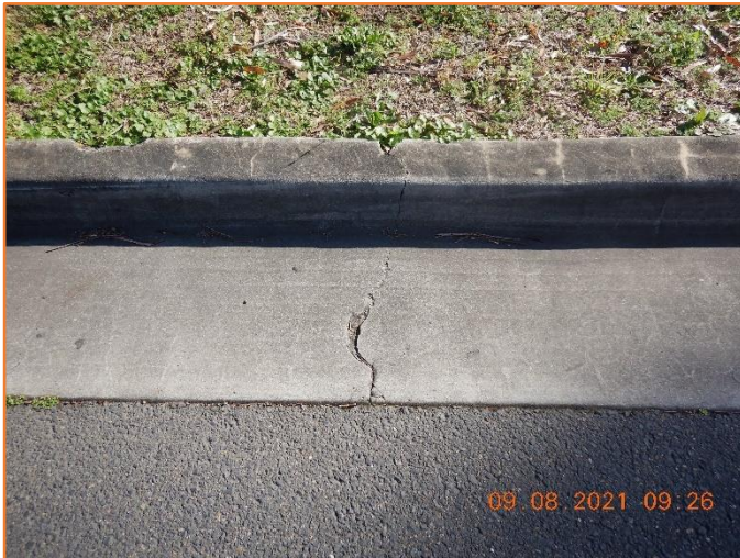
Figure 232: Reasonable - General condition of kerb and gutter. Minor hairline cracking observed.
