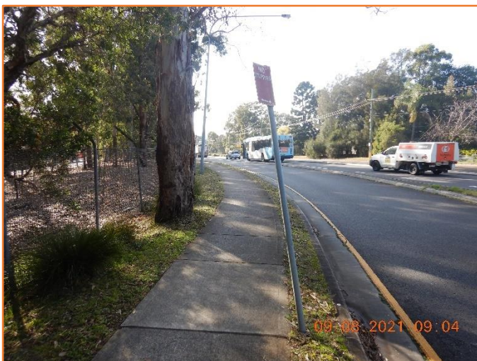
Figure 47: Defective - General condition of traffic signage. Major rotation observed.
