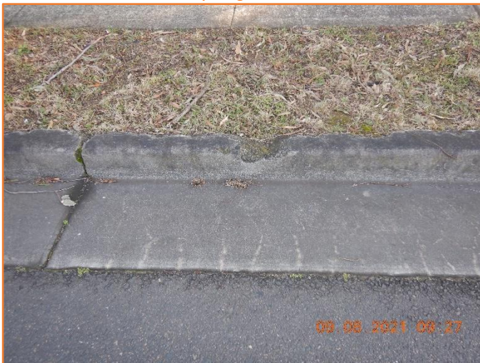
Figure 245: Poor - General condition of kerb and gutter. Moderate cracking and spalling observed.
