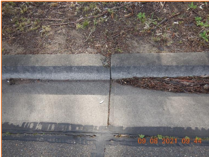
Figure 328: Reasonable - General condition of kerb and gutter. Minor spalling observed.
