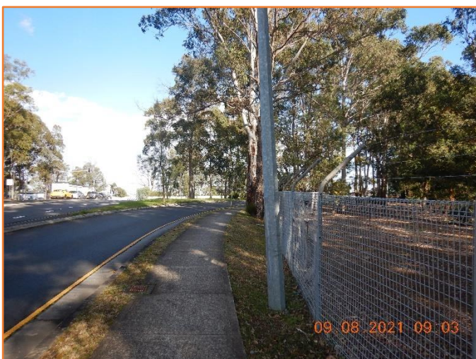
Figure 39: Poor - General condition of monopole assembly. Moderate rotation observed.
