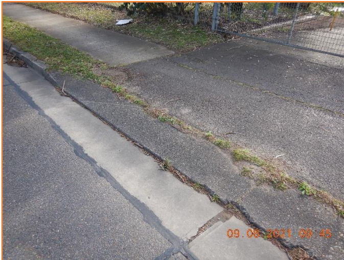
Figure 340: Reasonable - General condition of driveway crossover. Moderate cracking and loss of material observed.
