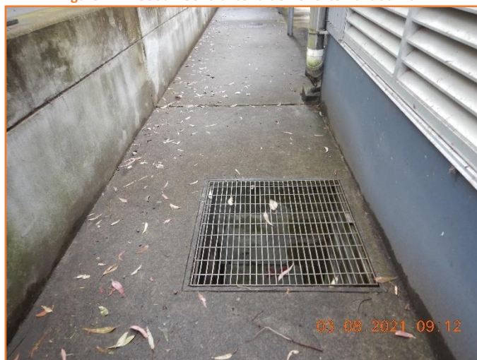
Figure 125: Good - General condition of rigid pavement and grated inlet pit.
