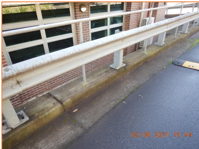
Figure 62: Reasonable - General condition of kerb and gutter.
