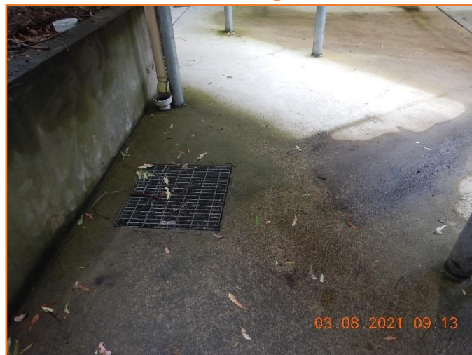
Figure 134: Reasonable - General condition of rigid pavement and grated inlet pit. Minor hairline cracking observed.
