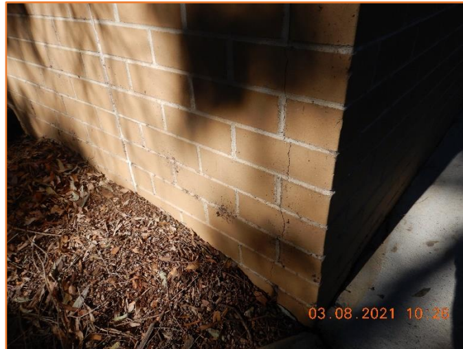
Figure 487: Reasonable - General condition of external masonry wall. Moderate hairline cracking observed.
