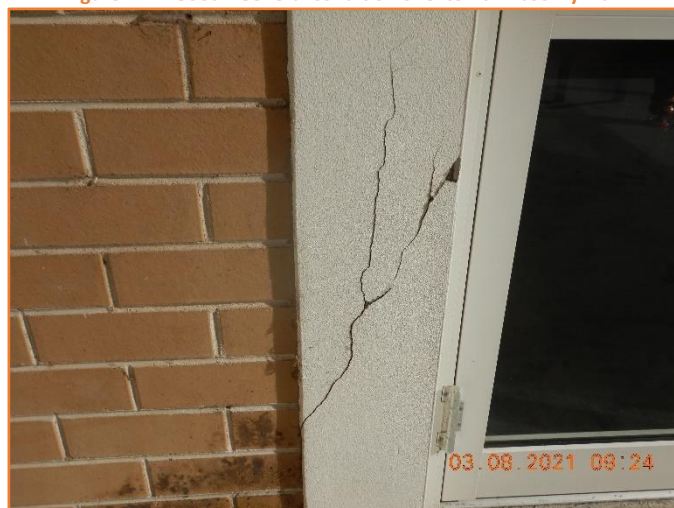
Figure 443: Reasonable - General condition of architrave and door. Moderate cracking observed.
