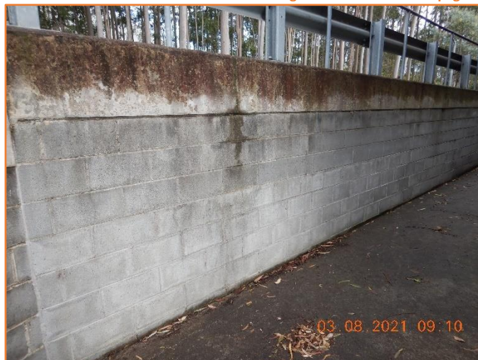
Figure 92: Reasonable - General condition of retaining wall. Minor water seepage observed.
