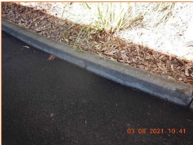
Figure 20: Reasonable - General condition of kerb and gutter.
