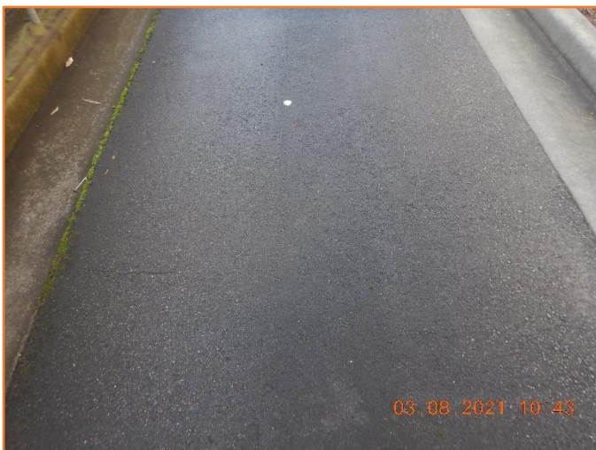
Figure 60: Reasonable - General condition of flexible pavement.
