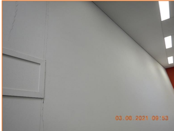
Figure 328: Poor - General condition of internal wall. Extensive cracking observed.
