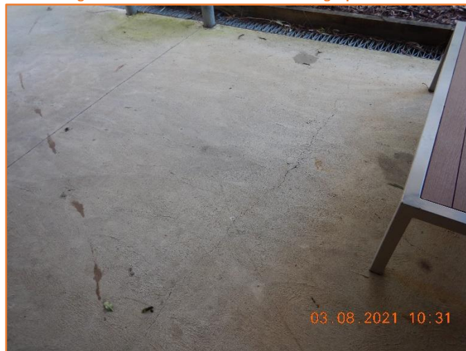
Figure 548: Reasonable - General condition of rigid pavement. Moderate hairline cracking observed.
