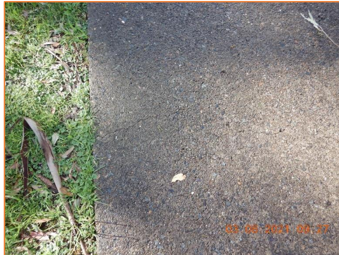
Figure 210: Reasonable - General condition of rigid pavement. Minor hairline cracking observed.
