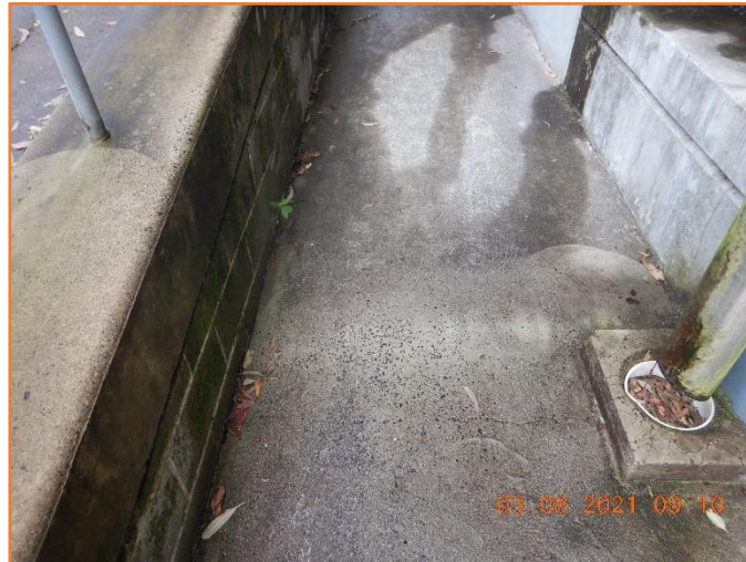
Figure 87: Reasonable - General condition of rigid pavement. Minor hairline cracking observed.
