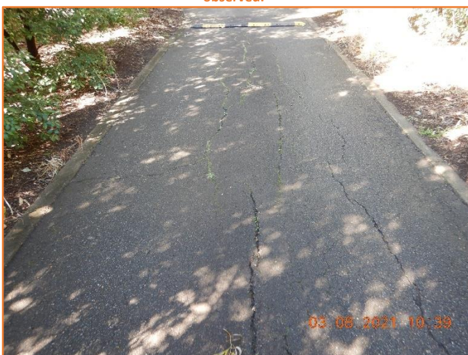
Figure 3: Poor - General condition of flexible pavement. Major cracking observed.
