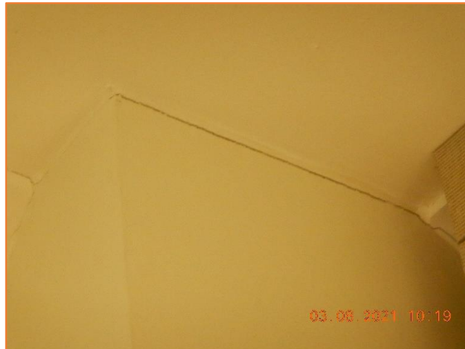
Figure 572: Reasonable - General condition of ceiling and cornice and wall. Minor hairline cracking observed.
