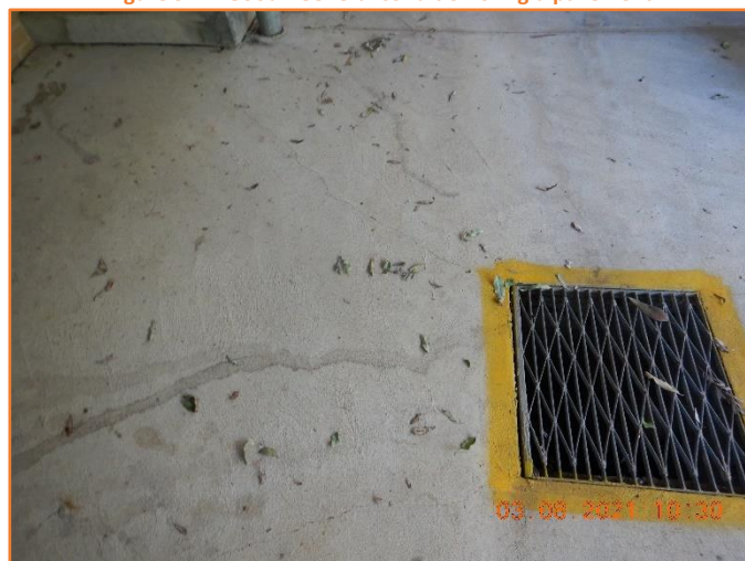
Figure 543: Reasonable - General condition of rigid pavement. Minor hairline cracking observed.
