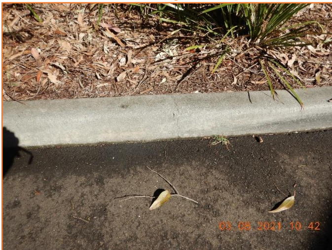
Figure 35: Reasonable - General condition of kerb and gutter. Minor hairline cracking observed.
