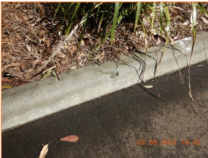
Figure 38: Reasonable - General condition of kerb and gutter. Minor spalling observed.
