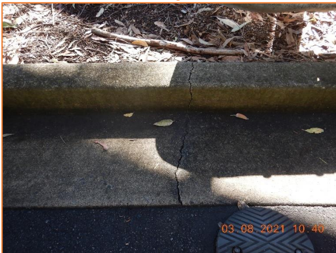
Figure 14: Reasonable - General condition of kerb and gutter. Moderate hairline cracking observed.
