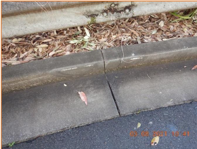
Figure 25: Reasonable - General condition of kerb and gutter. Moderate hairline cracking observed.
