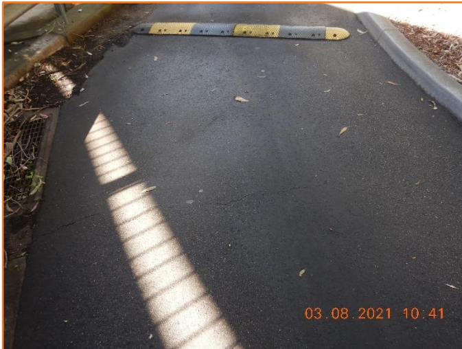
Figure 28: Reasonable - General condition of flexible pavement. Moderate hairline cracking observed.
