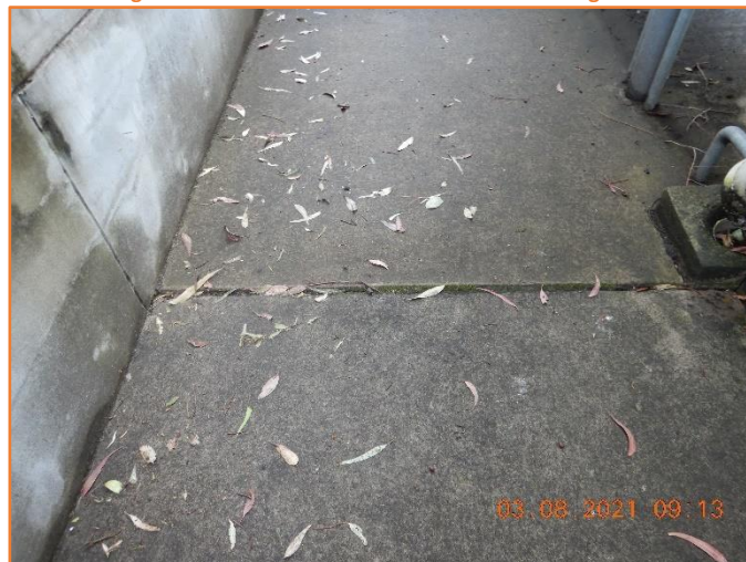
Figure 127: Reasonable - General condition of rigid pavement. Minor differential settlement observed.
