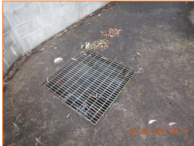
Figure 93: Good - General condition of grated inlet pit.
