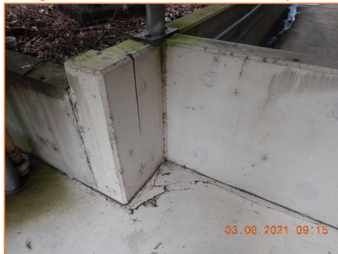
Figure 151: Poor - General condition of rigid pavement. Extensive cracking observed.
