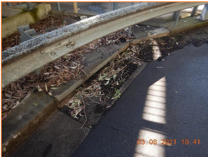
Figure 29: Reasonable - General condition of kerb inlet pit.
