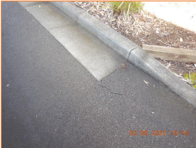
Figure 52: Reasonable - General condition of kerb and gutter and flexible pavement. Minor cracking observed.
