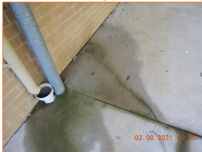
Figure 540: Reasonable - General condition of rigid pavement. Moderate hairline cracking observed.
