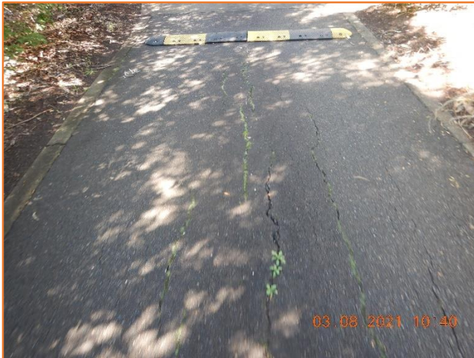
Figure 4: Poor - General condition of flexible pavement. Major cracking observed.
