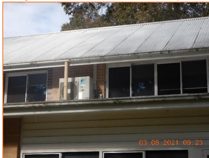
Figure 436: Good - General condition of external masonry wall.
