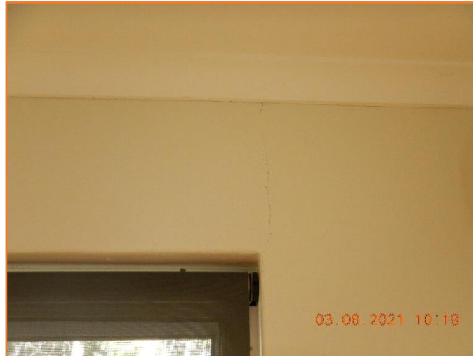
Figure 574: Reasonable - General condition of architrave and window. Minor hairline cracking observed.
