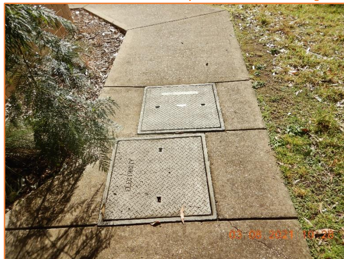
Figure 515: Reasonable - General condition of service pit.
