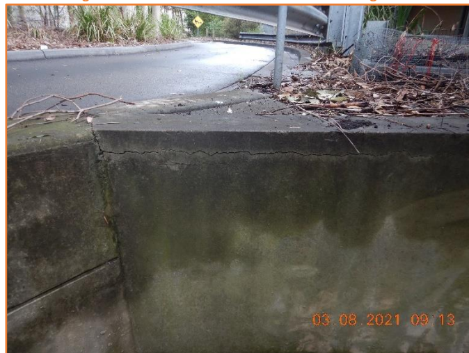
Figure 133: Reasonable - General condition of retaining wall. Moderate hairline cracking observed.
