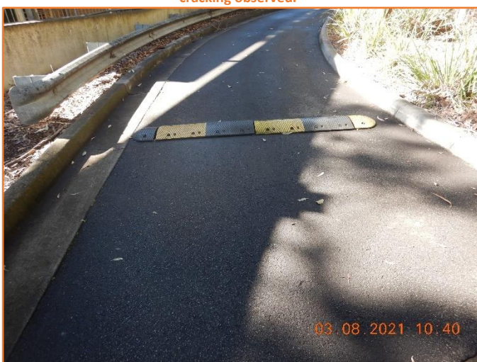
Figure 12: Reasonable - General condition of flexible pavement.
