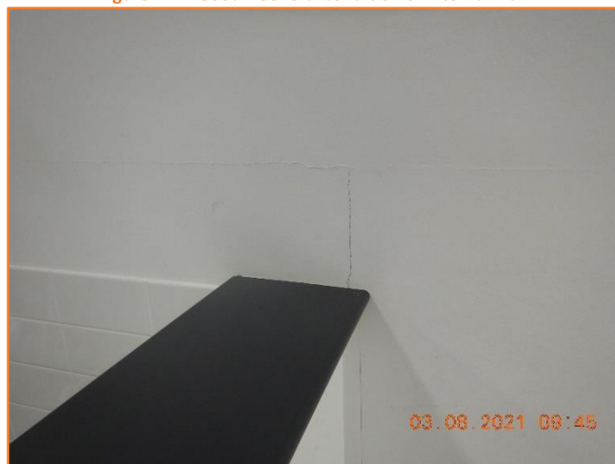
Figure 272: Reasonable - General condition of internal wall. Minor hairline cracking observed.
