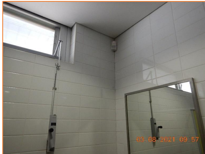
Figure 343: Reasonable - General condition of tiled wall. Moderate hairline cracking observed.
