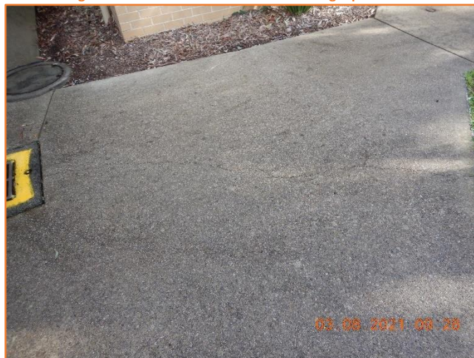
Figure 215: Reasonable - General condition of rigid pavement. Moderate hairline cracking observed.
