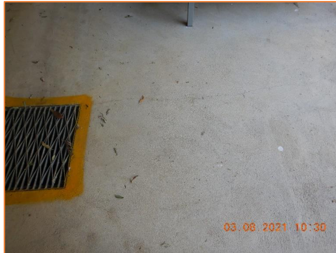
Figure 544: Reasonable - General condition of rigid pavement. Minor hairline cracking observed.
