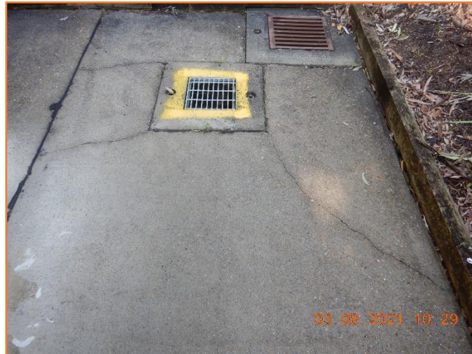
Figure 532: Poor - General condition of rigid pavement and grated inlet pit. Moderate hairline cracking observed.
