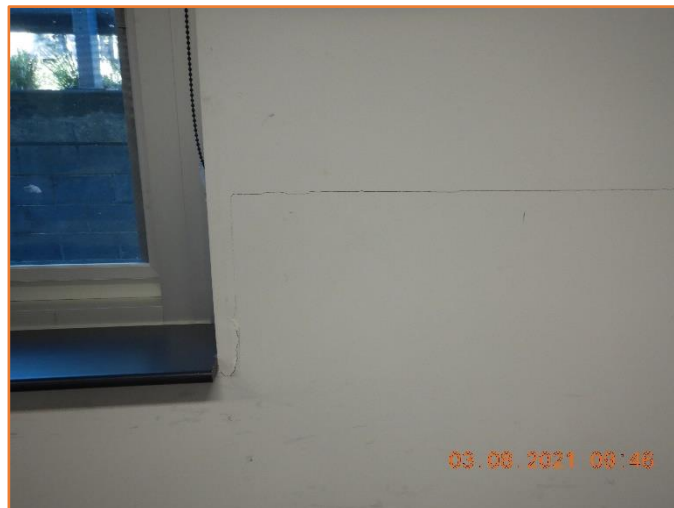
Figure 280: Reasonable - General condition of internal wall. Moderate hairline cracking observed.
