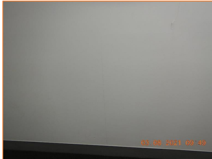
Figure 297: Reasonable - General condition of internal wall. Minor hairline cracking observed.
