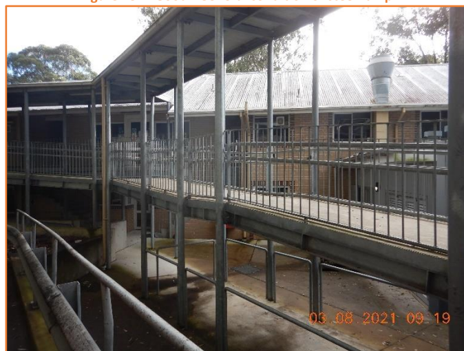
Figure 182: Good - General condition of steel ramp.
