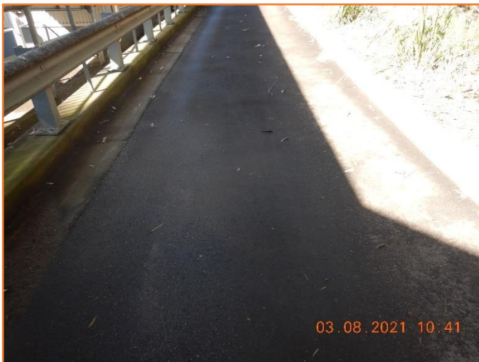
Figure 32: Reasonable - General condition of flexible pavement.
