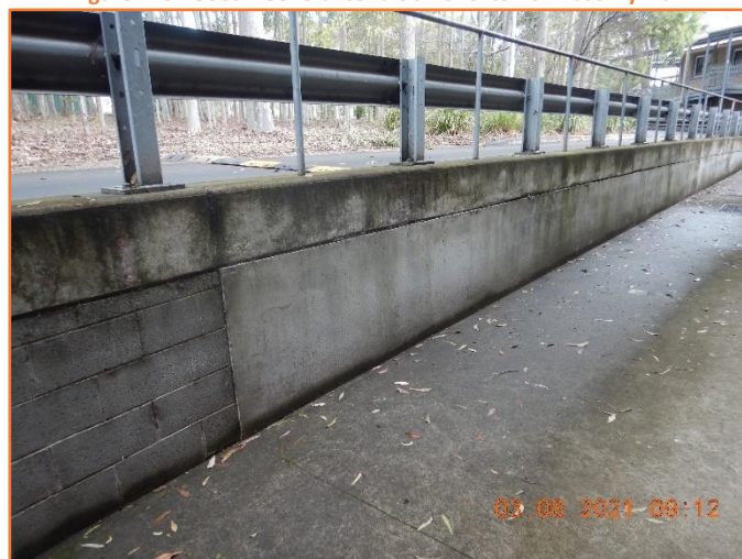
Figure 119: Good - General condition of retaining wall.
