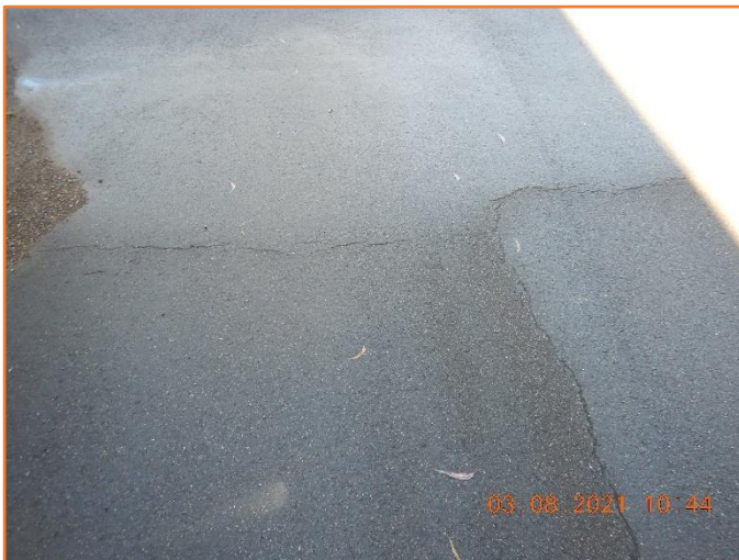
Figure 68: Poor - General condition of flexible pavement. Moderate cracking observed.
