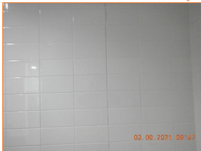
Figure 350: Reasonable - General condition of tiled wall. Moderate cracking observed.
