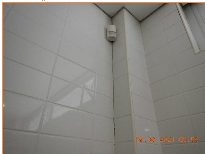
Figure 341: Reasonable - General condition of tiled wall. Moderate hairline cracking observed.
