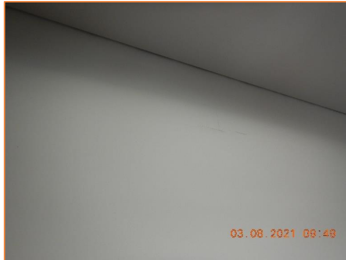
Figure 300: Reasonable - General condition of internal wall. Minor hairline cracking observed.
