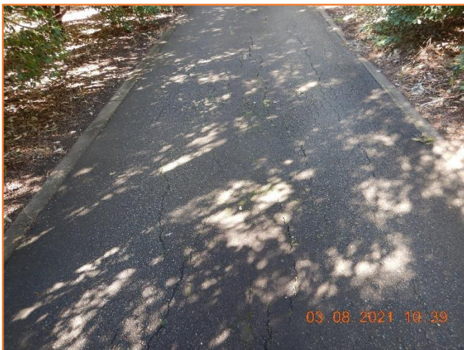
Figure 2: Poor - General condition of flexible pavement. Major cracking observed.
