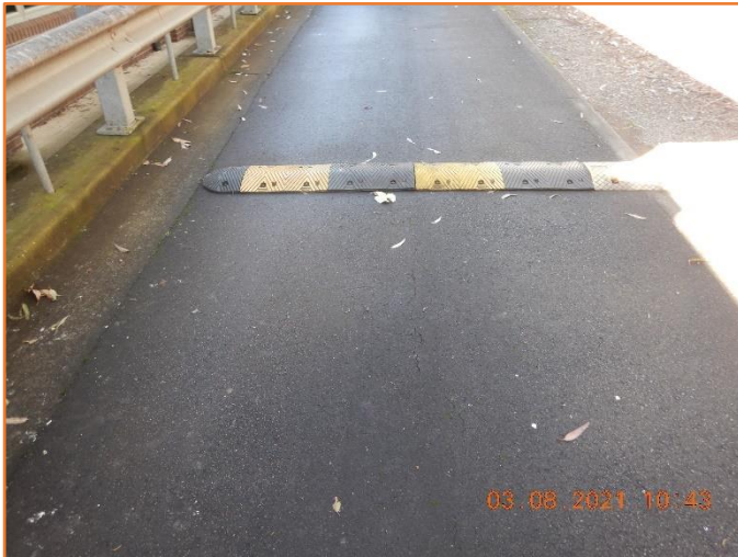
Figure 43: Reasonable - General condition of flexible pavement. Minor cracking observed.
