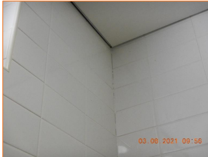
Figure 342: Reasonable - General condition of tiled wall. Moderate hairline cracking observed.
