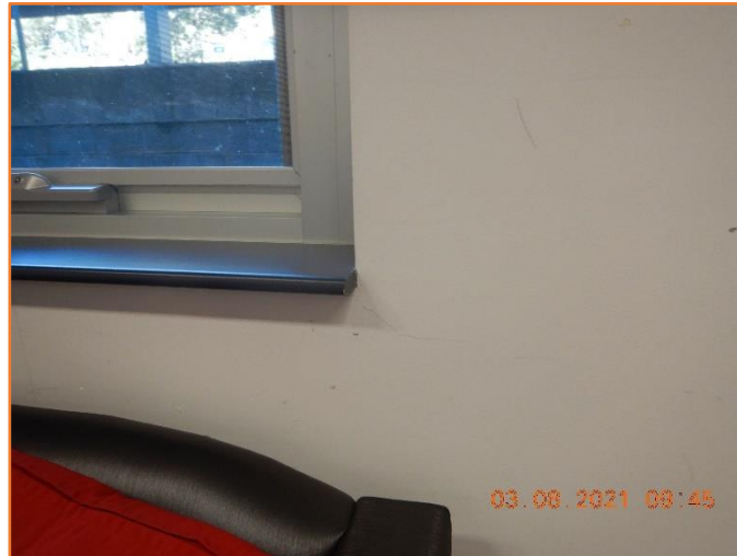
Figure 279: Reasonable - General condition of architrave and window. Minor hairline cracking observed.
