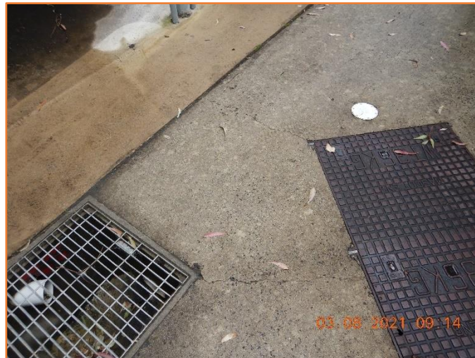
Figure 142: Reasonable - General condition of rigid pavement and grated inlet pit. Minor hairline cracking observed.
