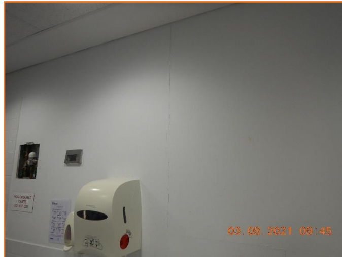
Figure 273: Reasonable - General condition of internal wall. Moderate hairline cracking observed.
