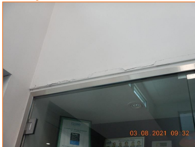
Figure 238: Reasonable - General condition of internal wall. Moderate hairline cracking observed.
