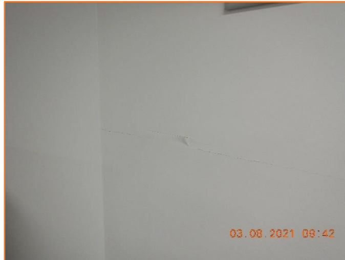
Figure 258: Reasonable - General condition of internal wall. Minor hairline cracking observed.
