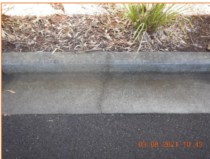
Figure 54: Reasonable - General condition of kerb and gutter. Minor hairline cracking observed.
