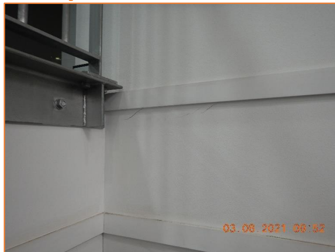
Figure 322: Reasonable - General condition of internal wall. Moderate cracking observed.
