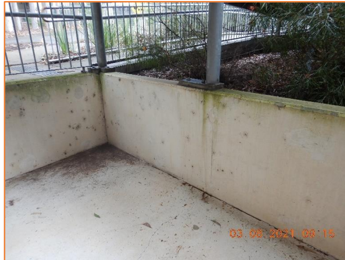
Figure 159: Reasonable - General condition of rigid pavement and retaining wall. Minor hairline cracking observed.
