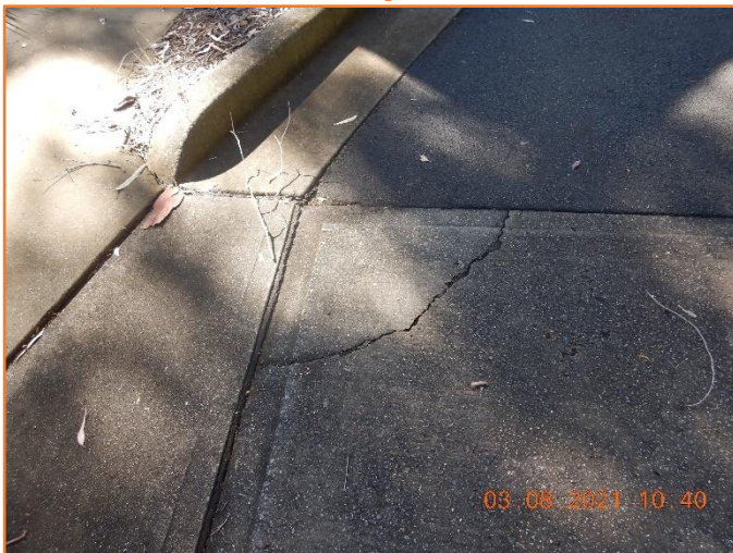
Figure 11: Reasonable - General condition of rigid pavement. Moderate cracking observed.
