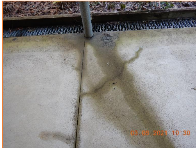
Figure 541: Reasonable - General condition of rigid pavement. Moderate hairline cracking observed.
