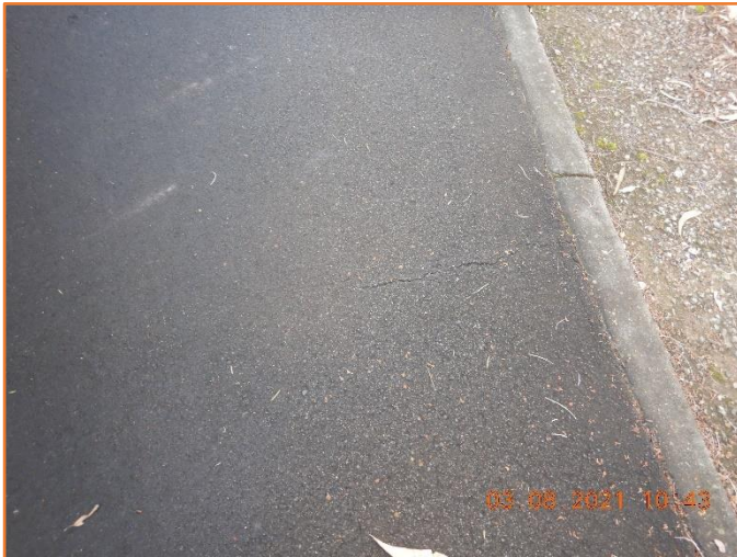
Figure 49: Reasonable - General condition of flexible pavement. Minor cracking observed.
