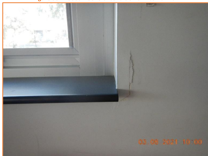
Figure 368: Poor - General condition of architrave and window. Moderate cracking observed.
