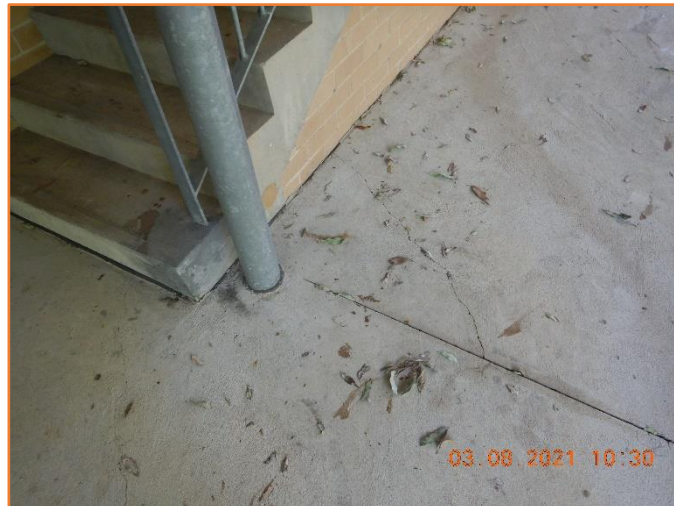
Figure 545: Reasonable - General condition of rigid pavement. Moderate hairline cracking observed.
