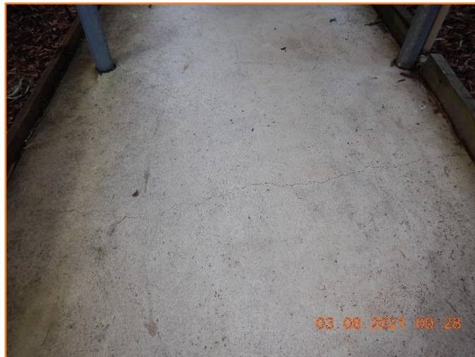
Figure 218: Reasonable - General condition of rigid pavement. Moderate hairline cracking observed.
