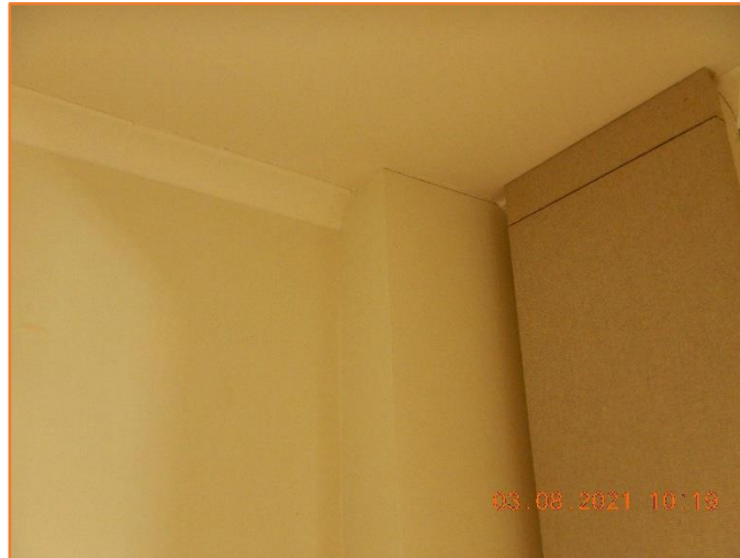
Figure 571: Reasonable - General condition of ceiling and cornice and wall. Minor hairline cracking observed.
