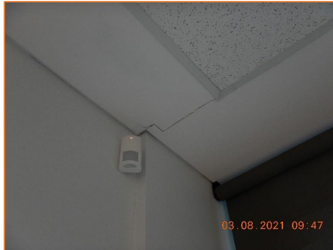
Figure 285: Reasonable - General condition of ceiling. Moderate hairline cracking observed.
