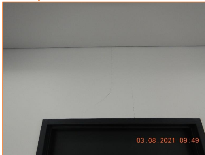
Figure 304: Reasonable - General condition of internal wall. Moderate hairline cracking observed.
