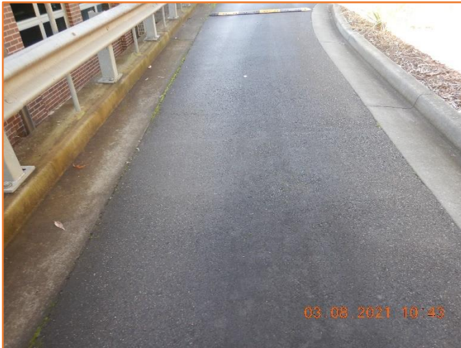
Figure 58: Reasonable - General condition of flexible pavement.
