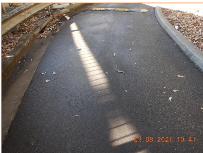
Figure 24: Reasonable - General condition of flexible pavement.
