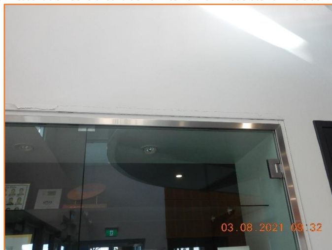
Figure 239: Reasonable - General condition of internal wall. Moderate hairline cracking observed.
