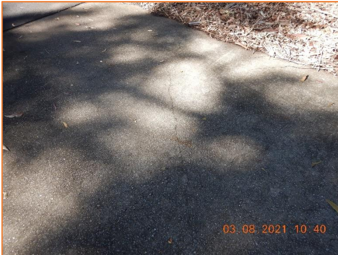
Figure 10: Reasonable - General condition of rigid pavement. Moderate hairline cracking observed.
