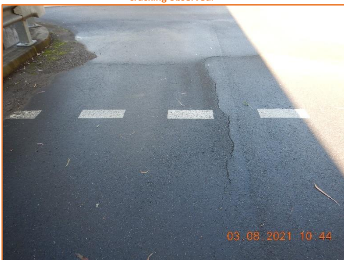
Figure 66: Poor - General condition of flexible pavement. Moderate cracking observed.
