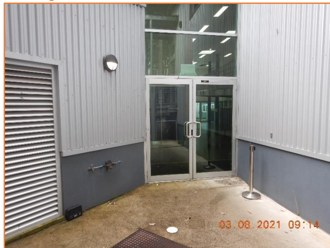
Figure 139: Good - General condition of external clad wall.
