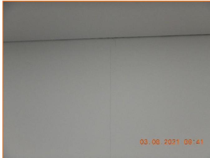
Figure 255: Reasonable - General condition of internal wall. Moderate hairline cracking observed.
