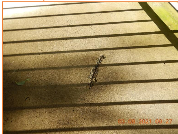
Figure 202: Poor - General condition of slab. Spalling and exposed reinforcement observed.
