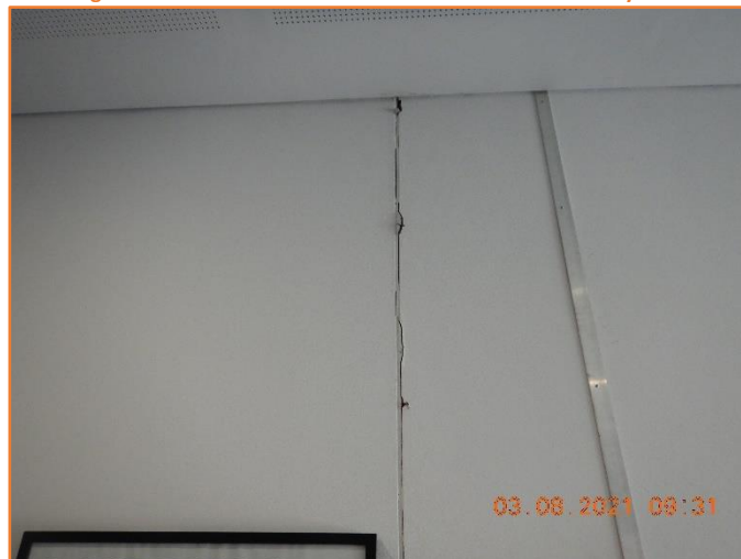
Figure 232: Reasonable - General condition of internal wall. Moderate hairline cracking observed.
