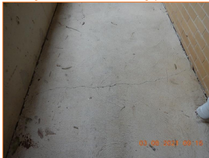
Figure 169: Reasonable - General condition of rigid pavement. Moderate hairline cracking observed.
