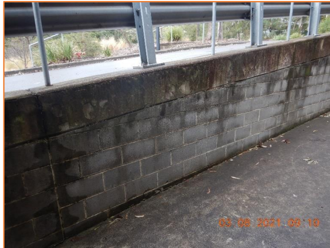
Figure 90: Reasonable - General condition of retaining wall. Minor water seepage observed.
