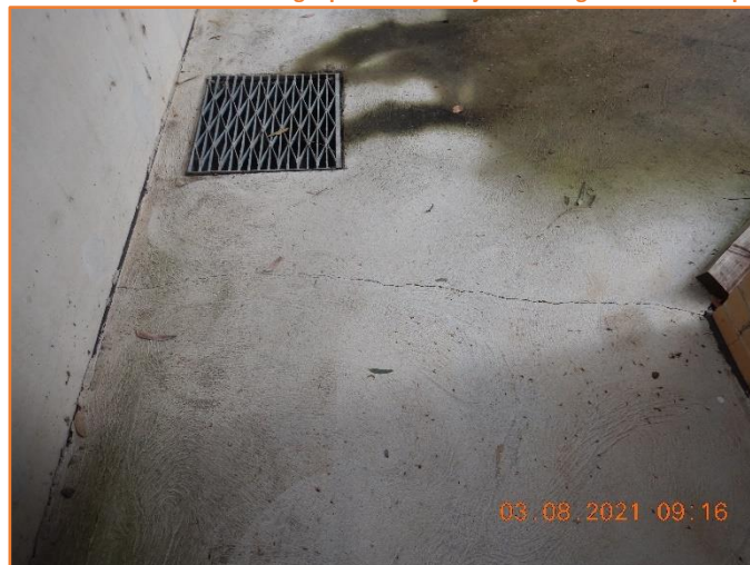
Figure 172: Reasonable - General condition of rigid pavement. Moderate cracking observed.
