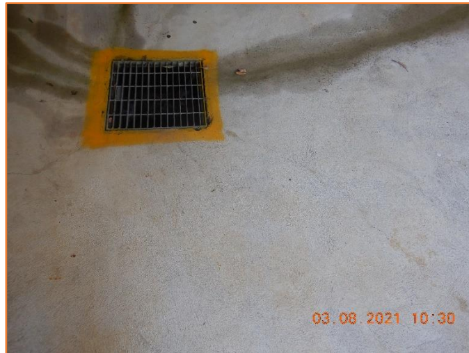
Figure 539: Reasonable - General condition of rigid pavement. Minor hairline cracking observed.
