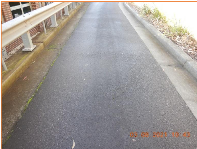
Figure 53: Reasonable - General condition of flexible pavement.
