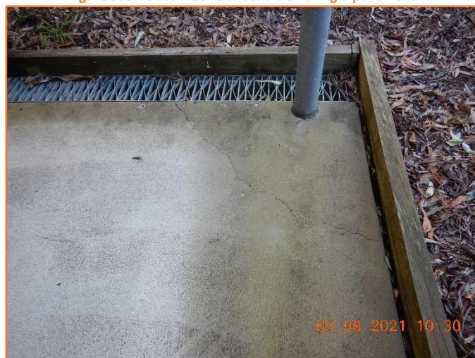
Figure 537: Reasonable - General condition of rigid pavement. Moderate hairline cracking observed.
