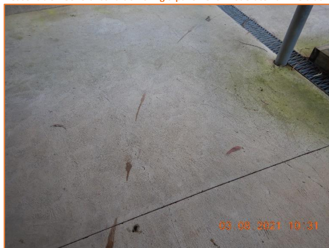
Figure 549: Reasonable - General condition of rigid pavement. Minor hairline cracking observed.
