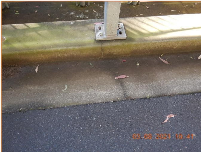
Figure 34: Reasonable - General condition of kerb and gutter. Minor hairline cracking observed.
