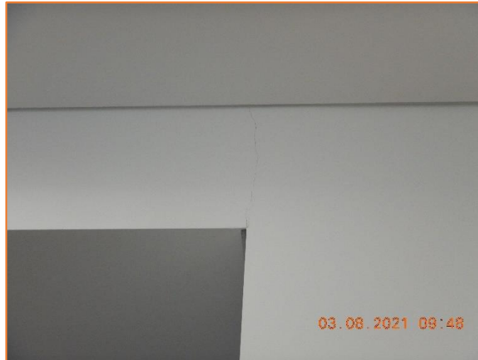
Figure 294: Reasonable - General condition of internal wall. Minor hairline cracking observed.
