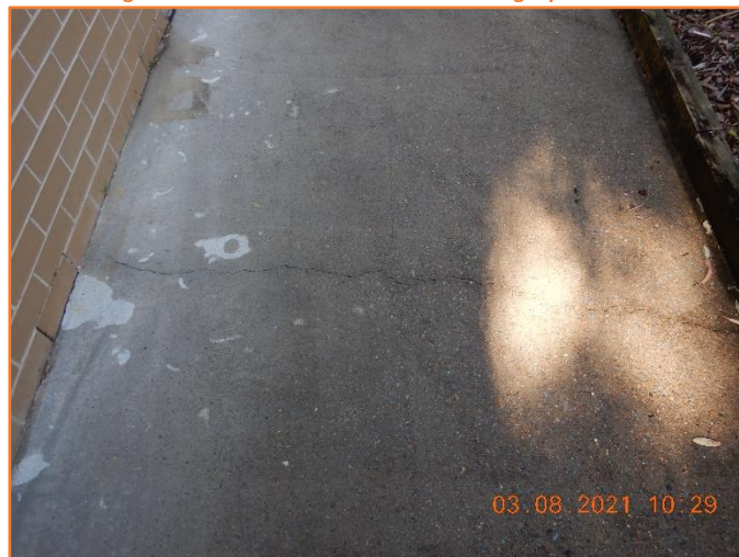
Figure 531: Reasonable - General condition of rigid pavement. Moderate hairline cracking observed.
