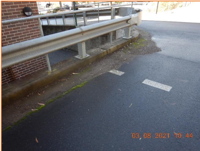
Figure 67: Reasonable - General condition of kerb and gutter.
