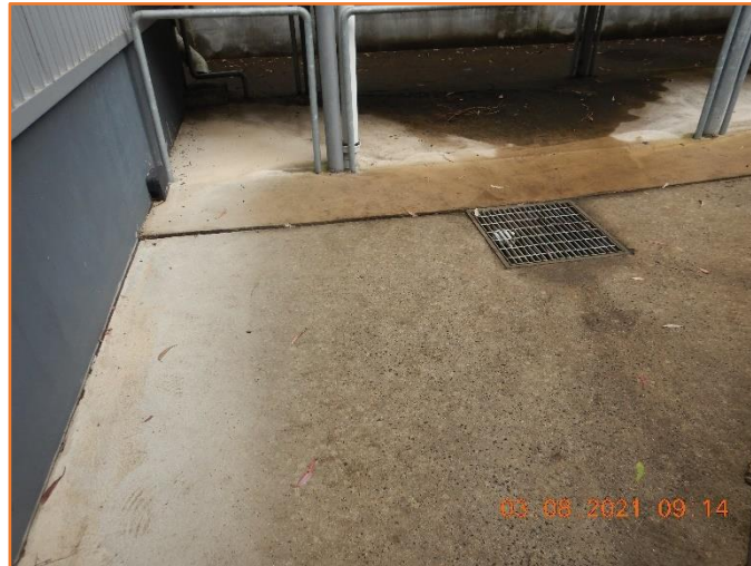
Figure 141: Good - General condition of rigid pavement and grated inlet pit.
