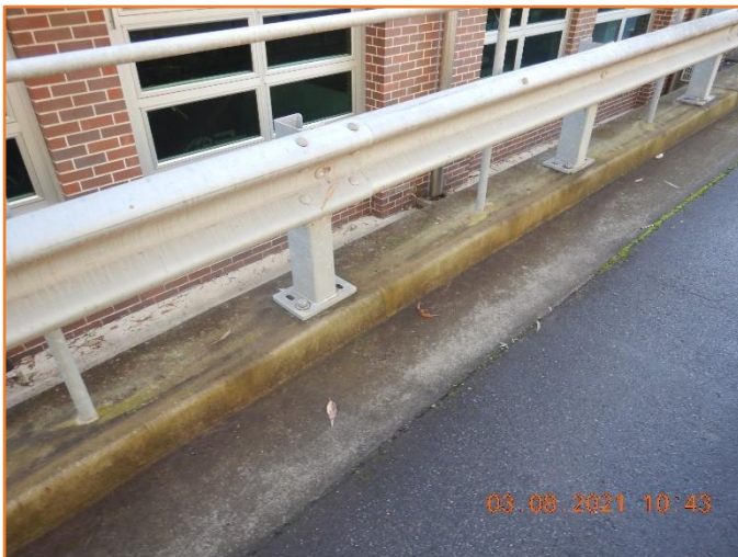
Figure 59: Reasonable - General condition of kerb and gutter.
