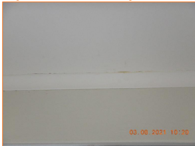
Figure 578: Reasonable - General condition of ceiling and cornice. Minor water damage observed.
