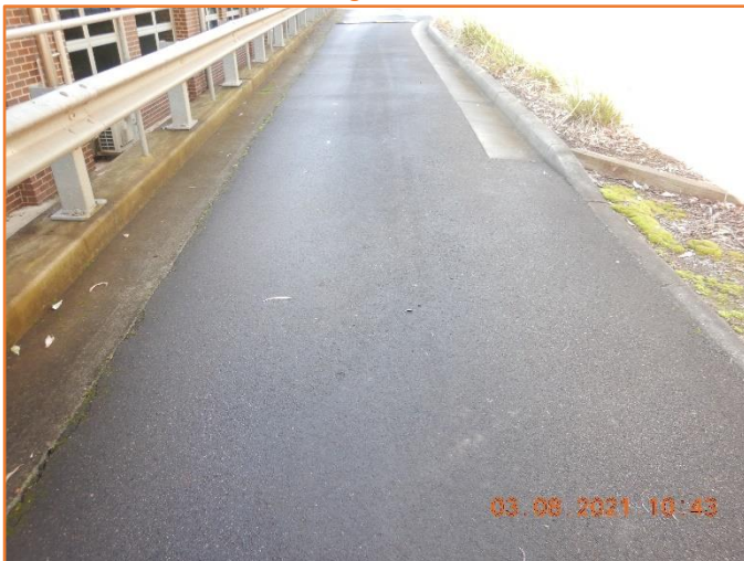
Figure 50: Reasonable - General condition of flexible pavement.
