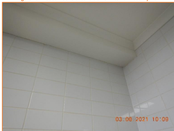
Figure 455: Reasonable - General condition of tiled wall. Minor hairline cracking observed.
