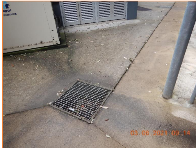
Figure 144: Reasonable - General condition of rigid pavement and grated inlet pit. Moderate hairline cracking observed.
