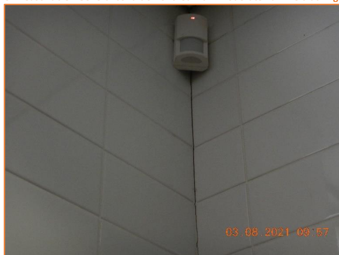
Figure 344: Reasonable - General condition of tiled wall. Moderate hairline cracking observed.
