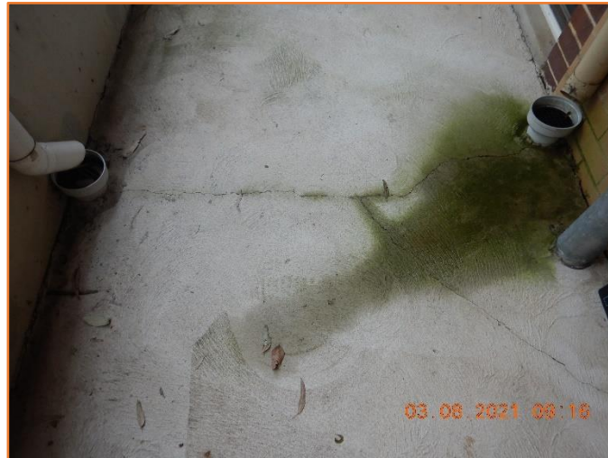
Figure 171: Poor - General condition of rigid pavement. Major cracking and water seepage observed.
