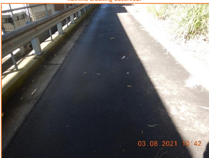
Figure 36: Reasonable - General condition of flexible pavement.
