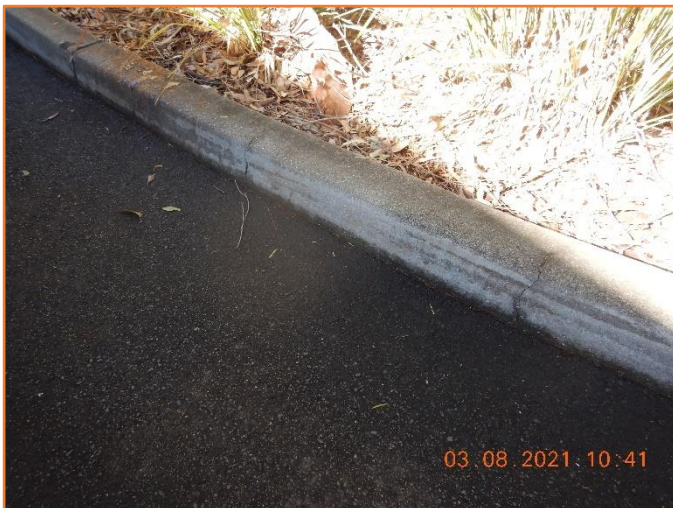
Figure 17: Reasonable - General condition of kerb and gutter. Minor hairline cracking observed.
