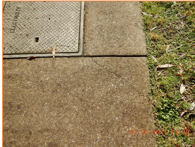
Figure 514: Good - General condition of footpath. Minor hairline cracking observed.
