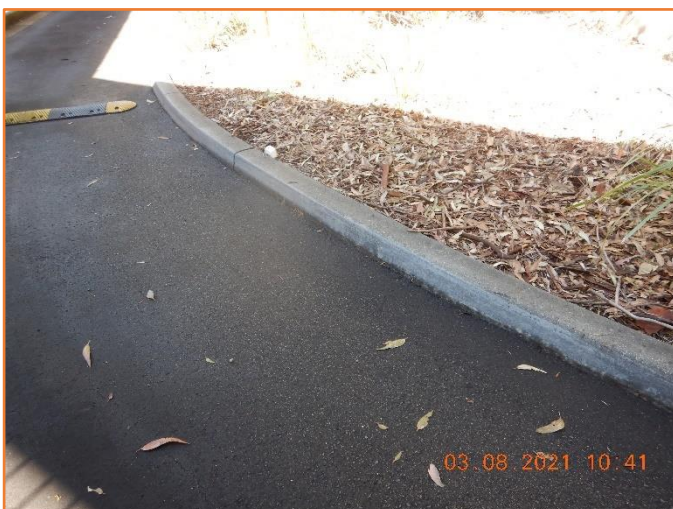
Figure 27: Reasonable - General condition of kerb and gutter.
