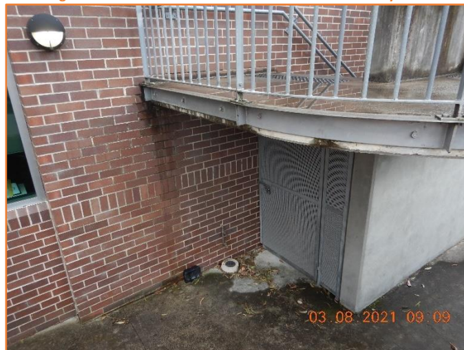
Figure 73: Reasonable - General condition of external masonry wall. Moderate water seepage observed.
