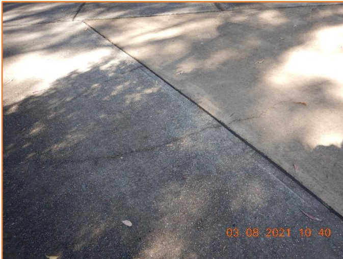
Figure 7: Reasonable - General condition of rigid pavement. Moderate hairline cracking observed.
