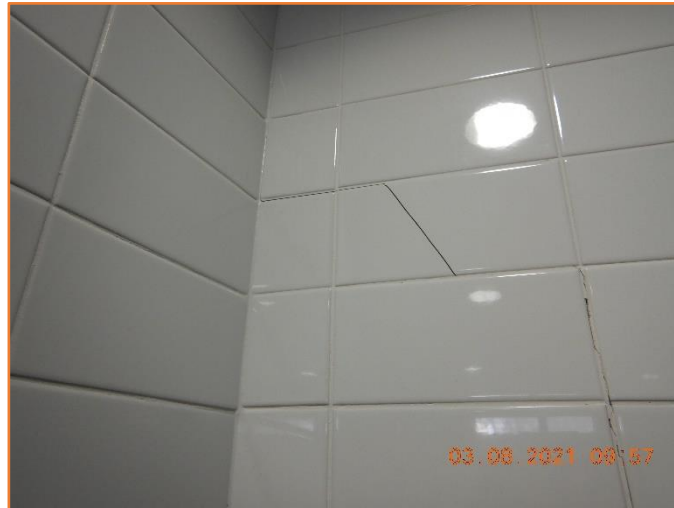
Figure 348: Reasonable - General condition of tiled wall. Moderate cracking observed.
