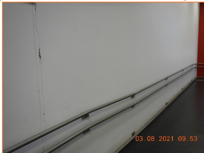
Figure 329: Poor - General condition of internal wall. Extensive cracking observed.
