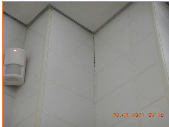
Figure 313: Reasonable - General condition of tiled wall. Minor hairline cracking observed.
