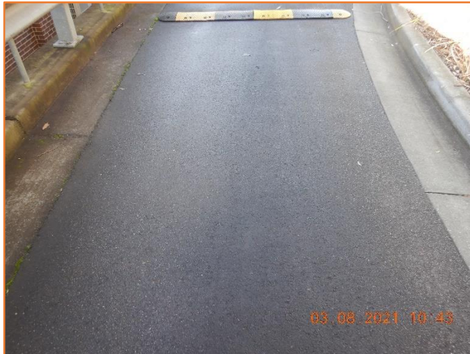
Figure 61: Reasonable - General condition of flexible pavement.
