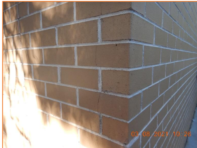
Figure 488: Reasonable - General condition of external masonry wall. Moderate hairline cracking observed.
