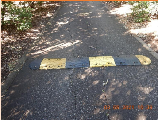
Figure 1: Poor - General condition of flexible pavement. Major cracking observed.
