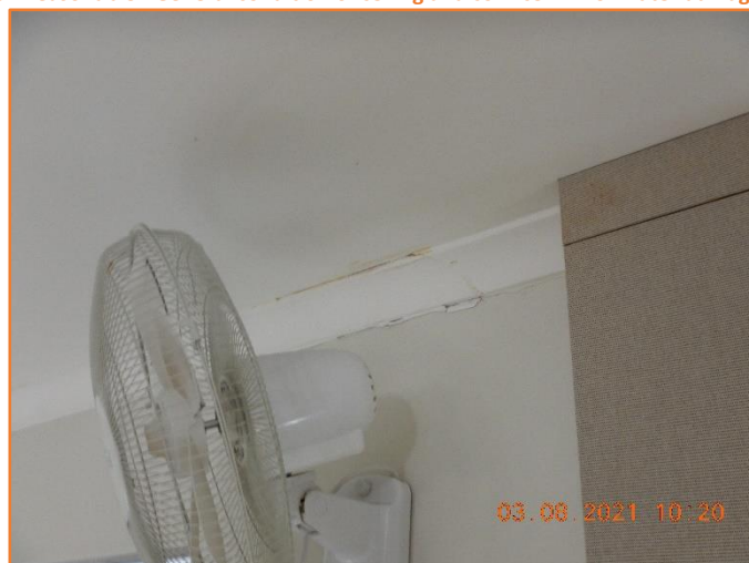
Figure 579: Poor - General condition of ceiling and cornice. Moderate cracking and water damage observed.
