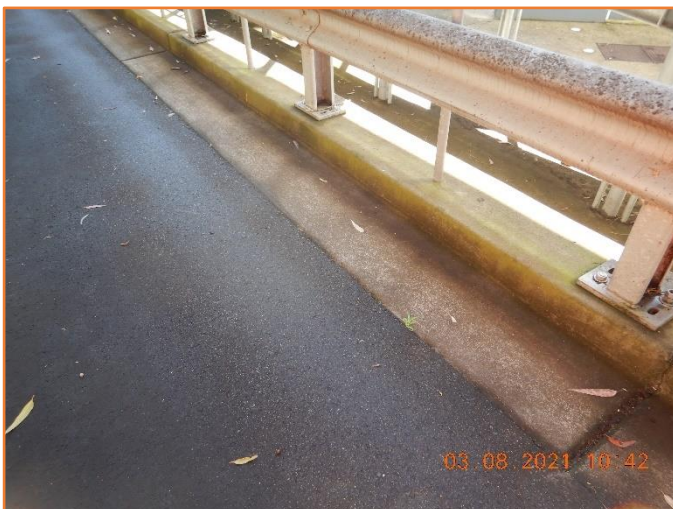
Figure 42: Reasonable - General condition of kerb and gutter.
