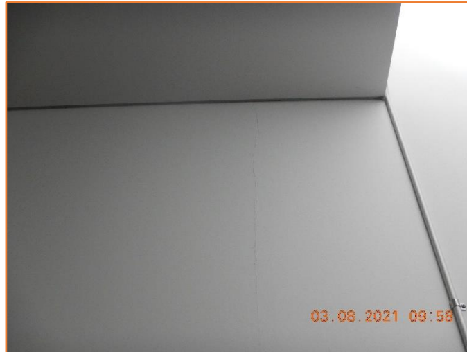
Figure 360: Reasonable - General condition of internal wall. Minor hairline cracking observed.
