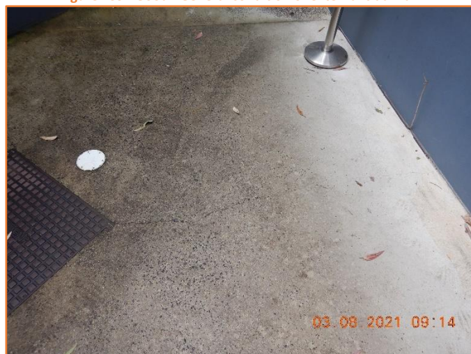
Figure 140: Reasonable - General condition of rigid pavement. Minor hairline cracking observed.
