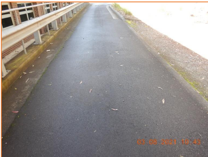
Figure 47: Reasonable - General condition of flexible pavement.
