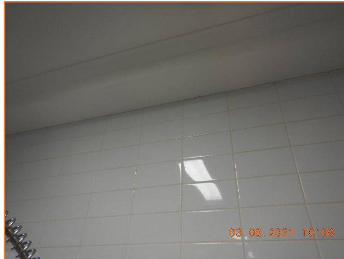
Figure 456: Reasonable - General condition of tiled wall. Minor hairline cracking observed.
