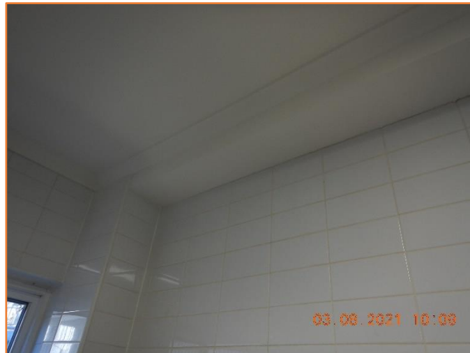
Figure 457: Reasonable - General condition of tiled wall. Minor hairline cracking observed.
