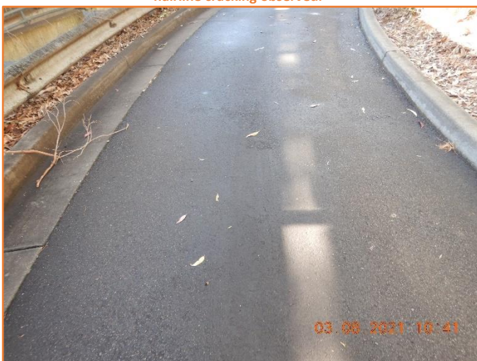
Figure 18: Reasonable - General condition of flexible pavement.
