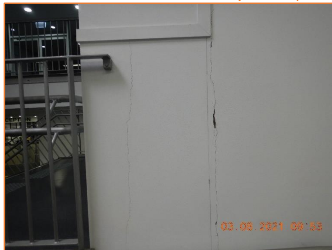
Figure 325: Poor - General condition of internal wall. Extensive cracking observed.
