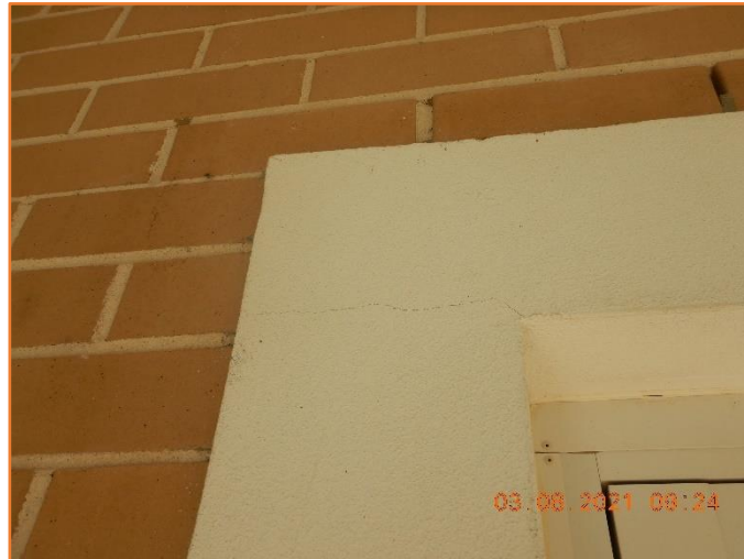
Figure 444: Reasonable - General condition of architrave and door. Minor hairline cracking observed.
