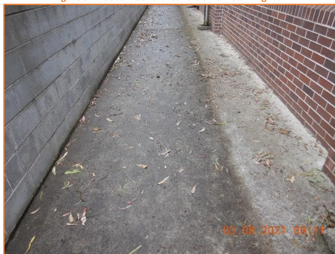
Figure 98: Good - General condition of rigid pavement.
