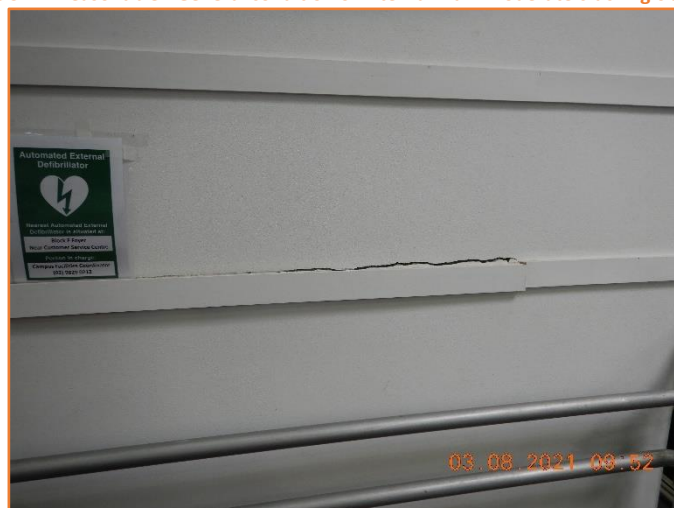
Figure 323: Reasonable - General condition of internal wall. Moderate cracking observed.
