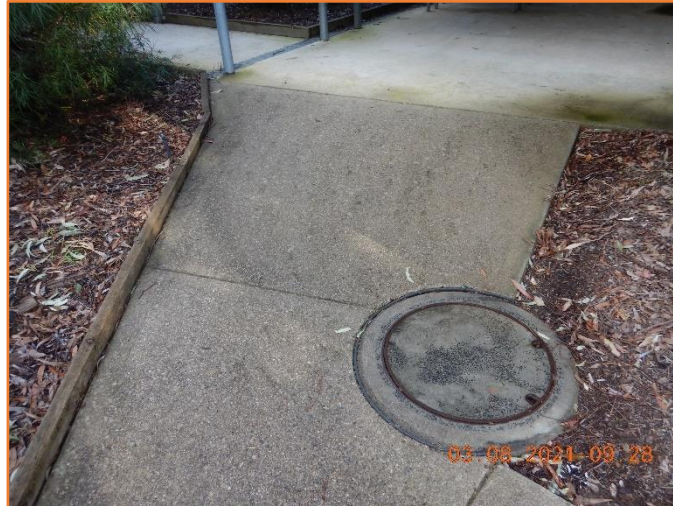
Figure 216: Reasonable - General condition of rigid pavement and sewer manhole.
