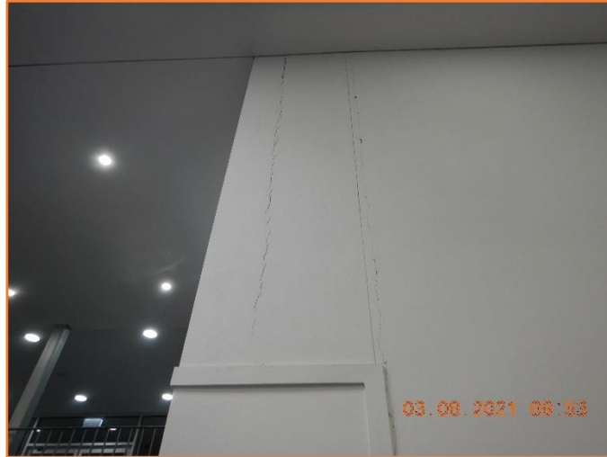
Figure 327: Poor - General condition of internal wall. Extensive cracking observed.
