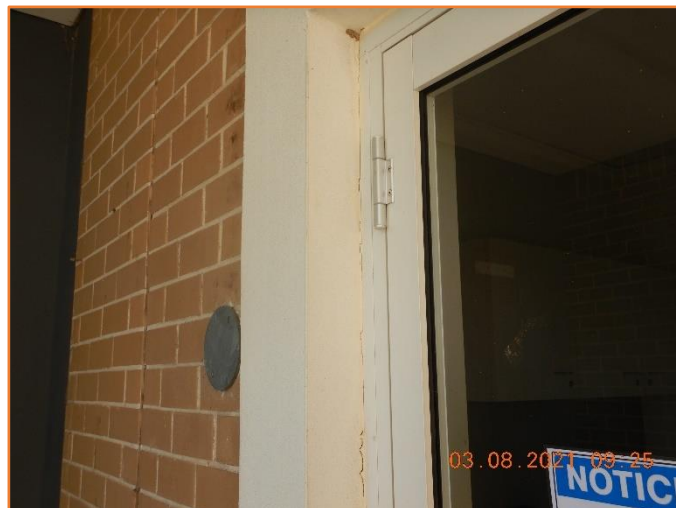
Figure 446: Reasonable - General condition of architrave and door. Minor hairline cracking observed.
