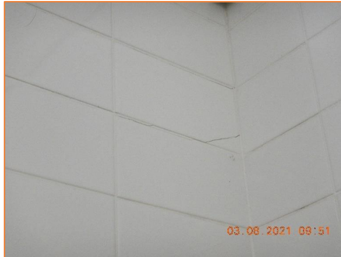
Figure 318: Reasonable - General condition of tiled wall. Minor hairline cracking observed.
