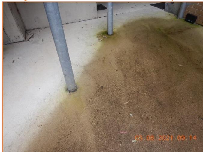
Figure 148: Reasonable - General condition of rigid pavement. Minor hairline cracking observed.
