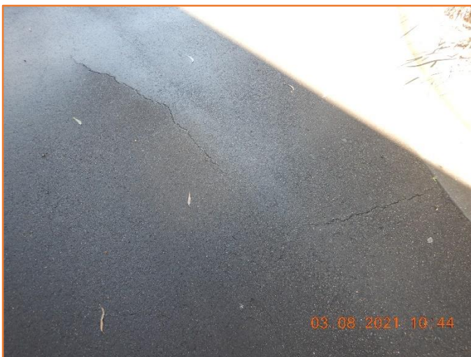
Figure 65: Reasonable - General condition of flexible pavement. Minor cracking observed.
