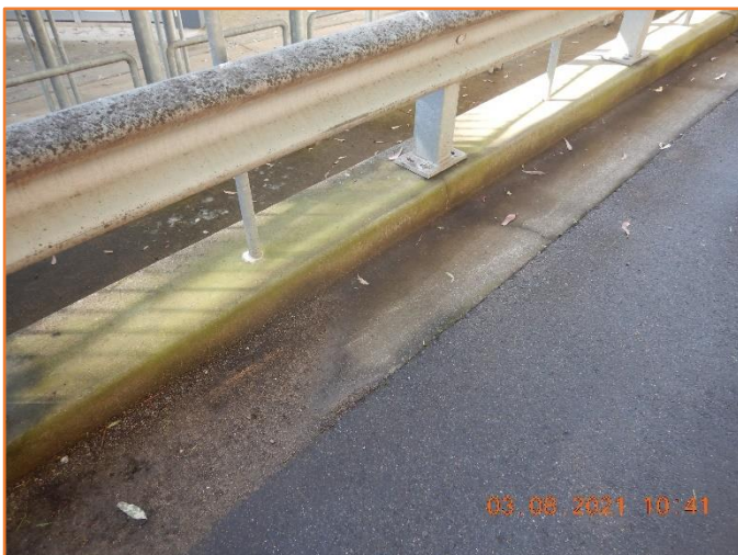
Figure 33: Reasonable - General condition of kerb and gutter. Minor hairline cracking observed.
