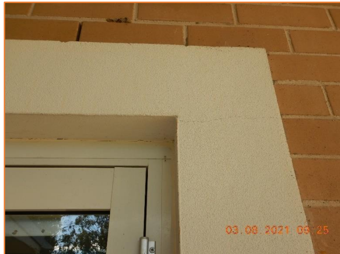
Figure 445: Reasonable - General condition of architrave and door. Minor hairline cracking observed.
