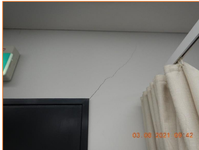
Figure 259: Poor - General condition of internal wall. Moderate cracking observed.
