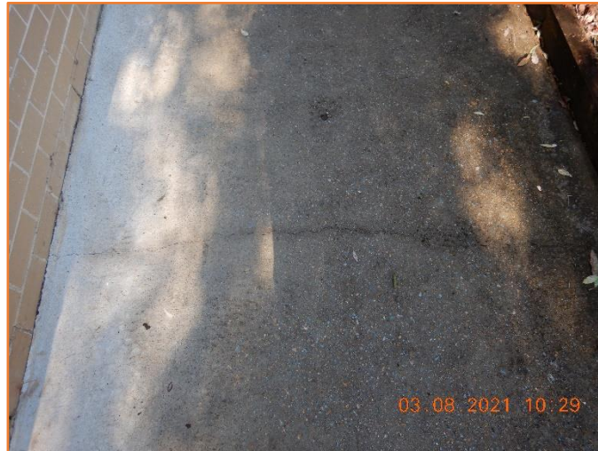
Figure 529: Reasonable - General condition of rigid pavement. Minor hairline cracking observed.
