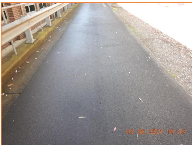
Figure 45: Reasonable - General condition of flexible pavement.
