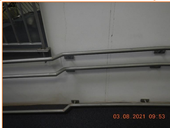
Figure 326: Poor - General condition of internal wall. Extensive cracking observed.
