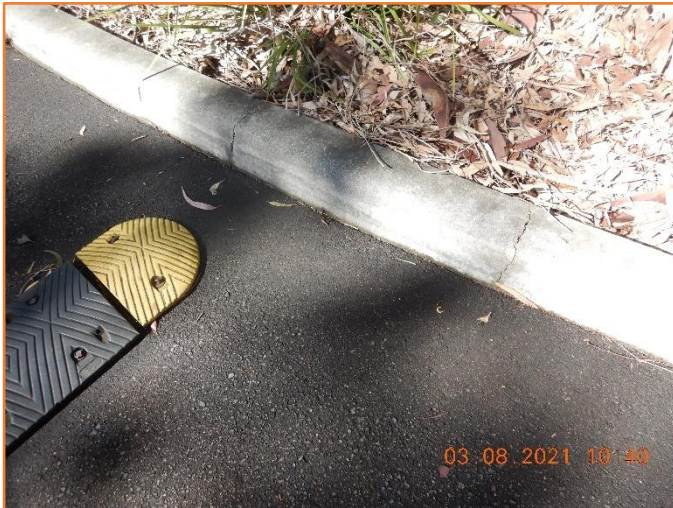
Figure 13: Reasonable - General condition of kerb and gutter. Minor hairline cracking observed.
