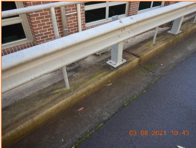
Figure 55: Reasonable - General condition of kerb and gutter.
