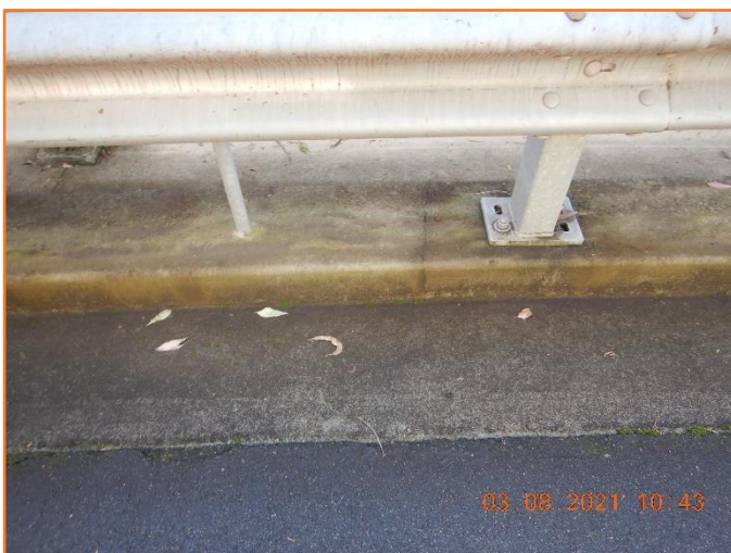
Figure 51: Reasonable - General condition of kerb and gutter. Minor hairline cracking observed.
