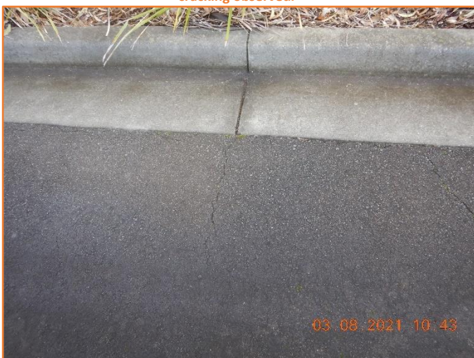
Figure 57: Reasonable - General condition of flexible pavement. Minor cracking observed.
