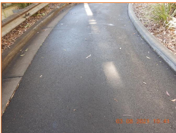
Figure 21: Reasonable - General condition of flexible pavement. Minor hairline cracking observed.
