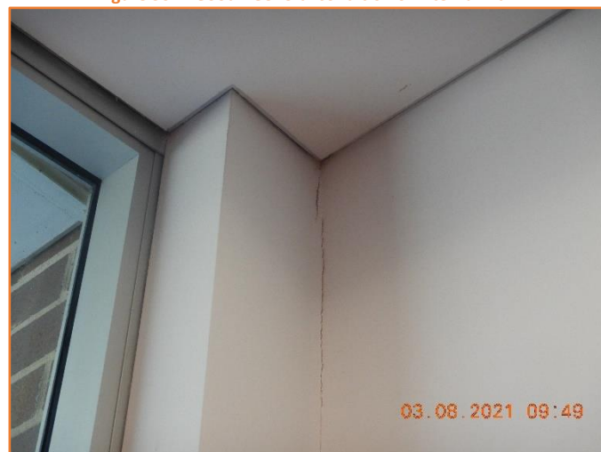
Figure 308: Reasonable - General condition of internal wall. Moderate cracking observed.
