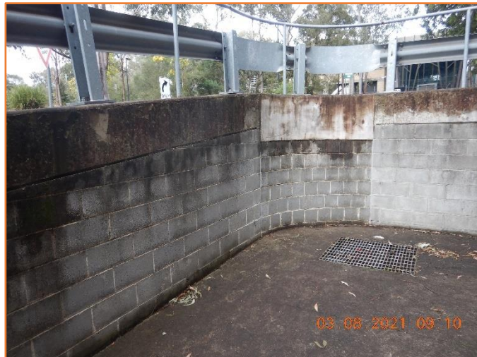
Figure 91: Reasonable - General condition of retaining wall. Minor water seepage observed.
