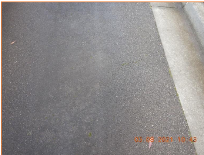
Figure 56: Reasonable - General condition of flexible pavement. Minor cracking observed.
