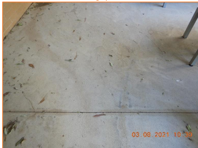
Figure 546: Reasonable - General condition of rigid pavement. Moderate hairline cracking observed.
