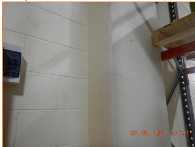
Figure 523: Reasonable - General condition of column. Minor hairline cracking observed.
