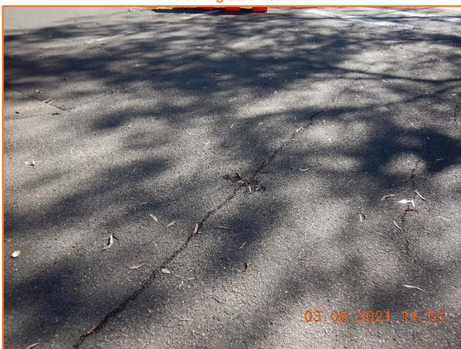
Figure 2: Reasonable - General condition of flexible pavement. Moderate cracking observed.
