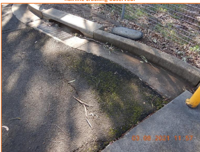
Figure 45: Reasonable - General condition of kerb and gutter and kerb inlet pit.
