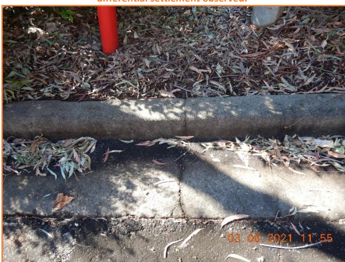
Figure 18: Reasonable - General condition of kerb and gutter. Moderate hairline cracking observed.
