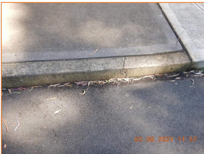
Figure 50: Reasonable - General condition of kerb and gutter. Moderate cracking observed.
