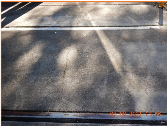
Figure 44: Reasonable - General condition of rigid pavement. Moderate hairline cracking observed.
