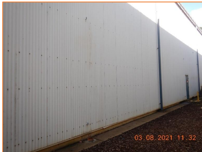
Figure 545: Reasonable - General condition of external clad wall. Minor corrosion observed.
