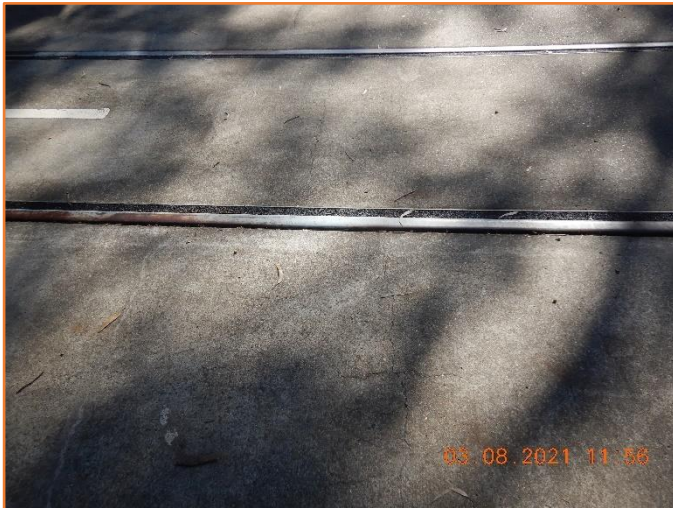
Figure 43: Reasonable - General condition of rigid pavement. Minor hairline cracking observed.
