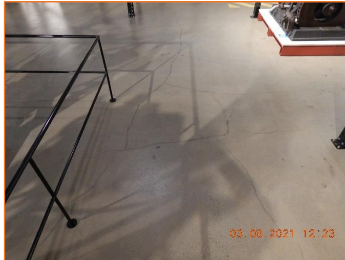
Figure 389: Reasonable - General condition of floor. Moderate hairline cracking observed.
