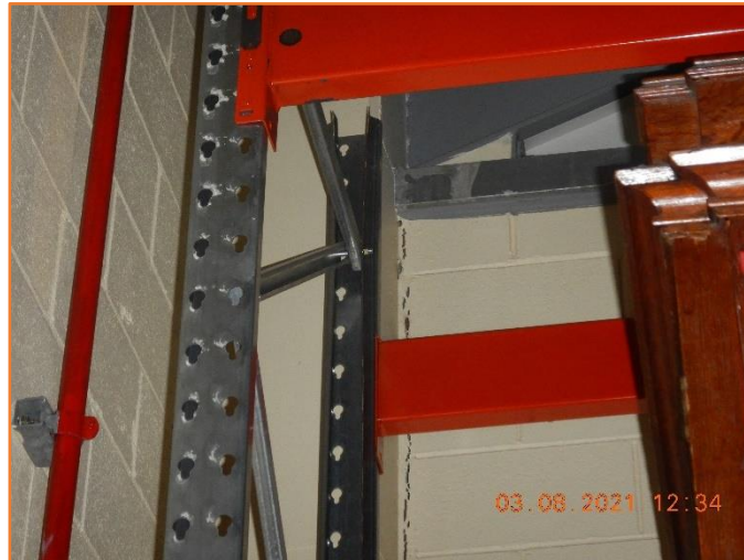
Figure 489: Reasonable - General condition of internal masonry wall. Moderate hairline cracking observed.
