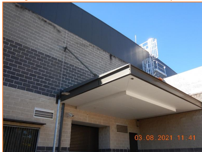
Figure 629: Reasonable - General condition of external masonry wall. Minor water seepage observed.
