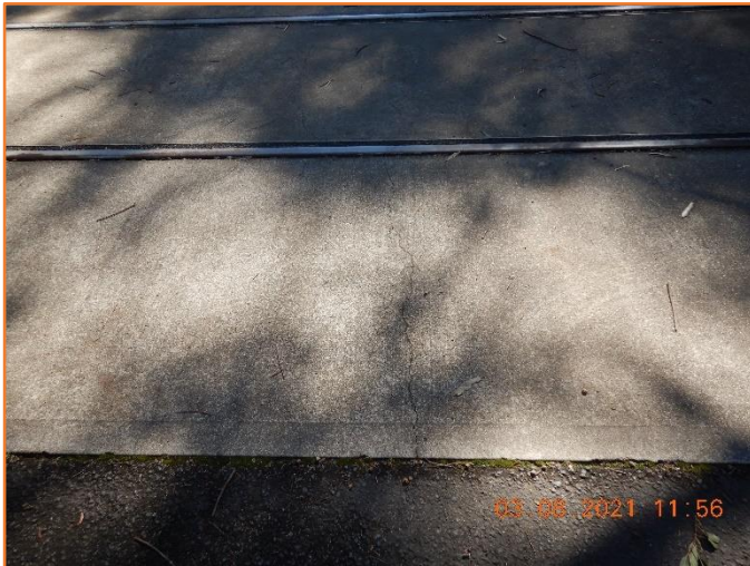
Figure 37: Reasonable - General condition of rigid pavement. Moderate hairline cracking observed.
