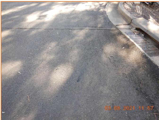
Figure 47: Reasonable - General condition of flexible pavement. Minor cracking observed.
