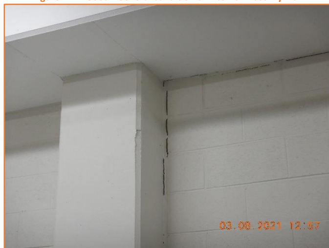
Figure 723: Reasonable - General condition of internal masonry wall. Moderate hairline cracking observed.
