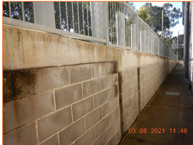
Figure 674: Reasonable - General condition of retaining wall. Moderate water seepage observed.
