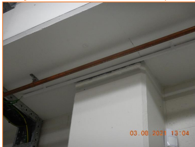
Figure 764: Reasonable - General condition of slab soffit and column. Moderate cracking observed.
