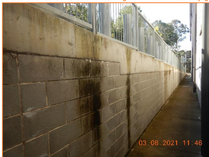
Figure 672: Reasonable - General condition of retaining wall. Moderate water seepage observed.
