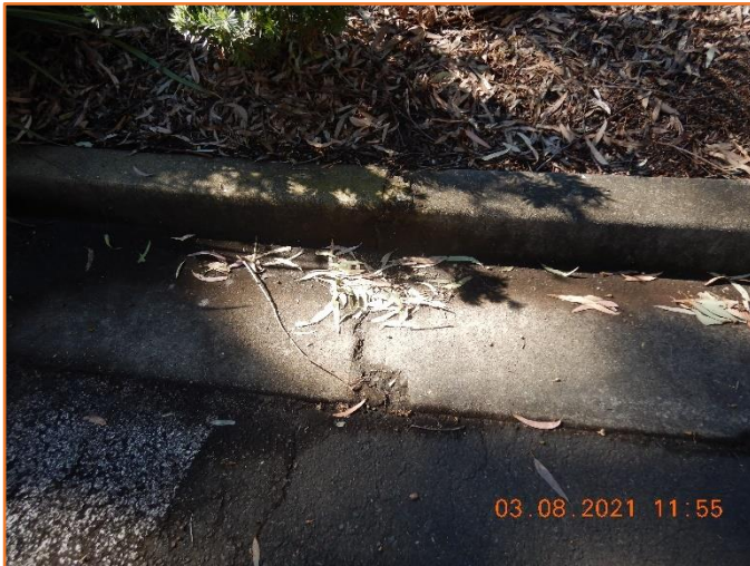
Figure 28: Reasonable - General condition of kerb and gutter. Moderate cracking observed.
