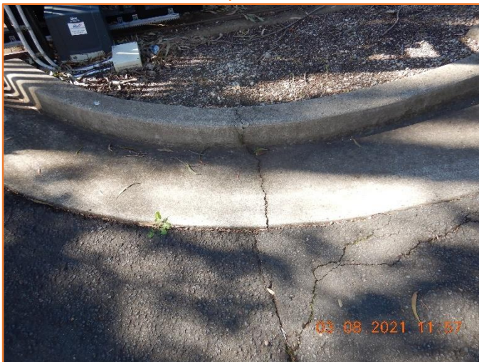
Figure 53: Poor - General condition of kerb and gutter and flexible pavement. Major cracking observed.
