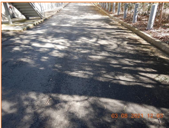
Figure 134: Reasonable - General condition of flexible pavement.
