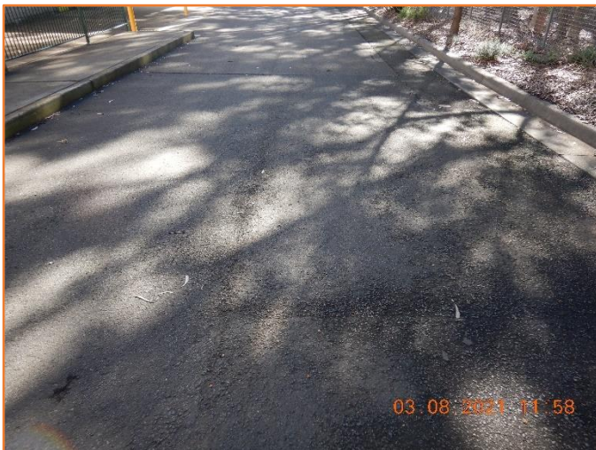
Figure 65: Reasonable - General condition of flexible pavement.
