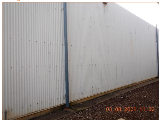
Figure 543: Reasonable - General condition of external clad wall. Minor corrosion observed.
