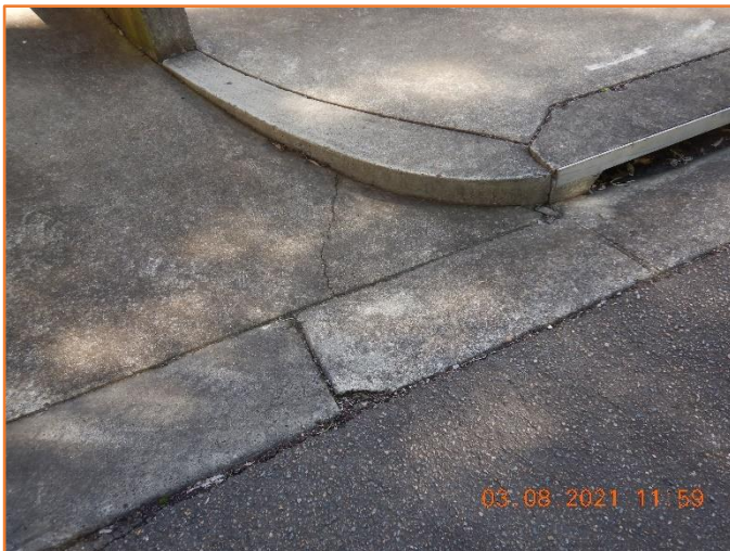
Figure 83: Reasonable - General condition of rigid pavement and gutter. Minor cracking observed.
