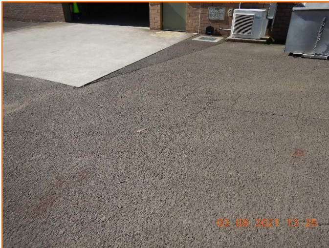
Figure 211: Reasonable - General condition of flexible pavement. Moderate cracking observed.
