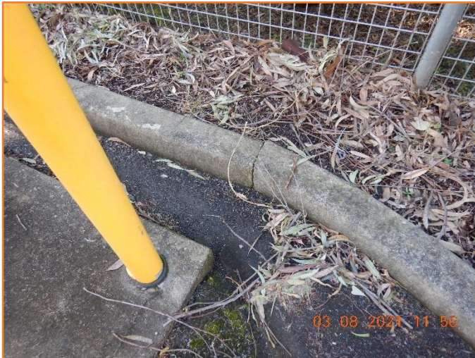
Figure 40: Reasonable - General condition of kerb and gutter. Moderate lateral displacement observed.
