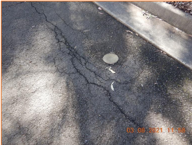
Figure 67: Poor - General condition of flexible pavement and service pit. Major cracking observed.
