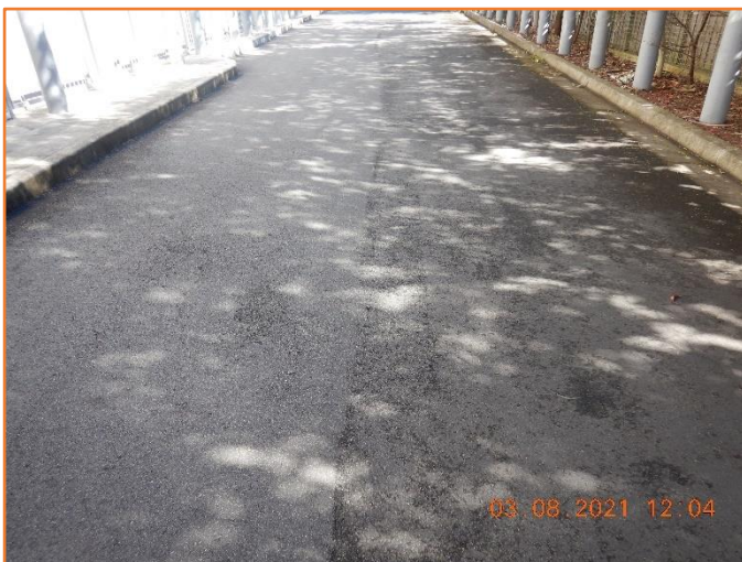
Figure 152: Reasonable - General condition of flexible pavement.
