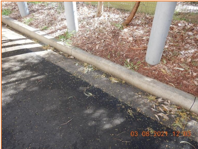
Figure 145: Reasonable - General condition of kerb and gutter.
