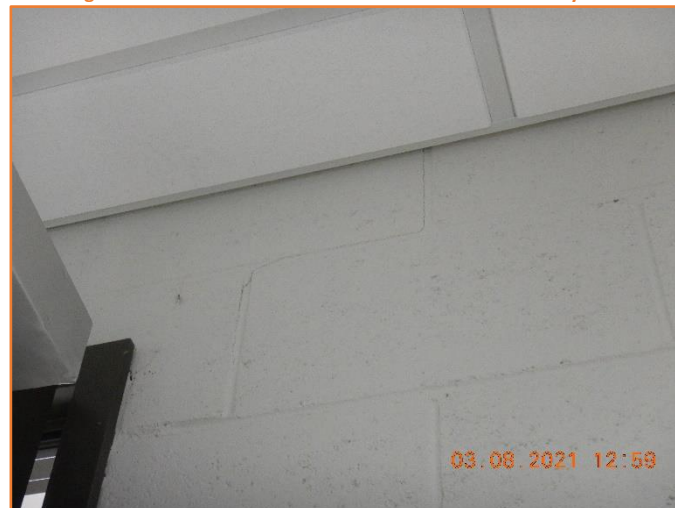
Figure 746: Reasonable - General condition of internal masonry wall. Minor step cracking observed.
