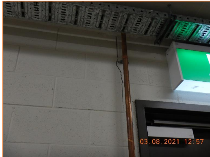
Figure 730: Poor - General condition of internal masonry wall. Moderate cracking observed.
