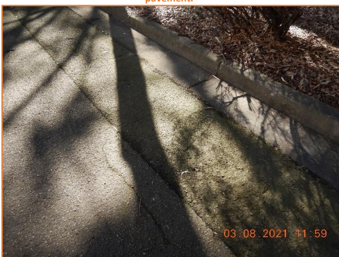
Figure 75: Reasonable - General condition of kerb and gutter and flexible pavement. Minor cracking observed.
