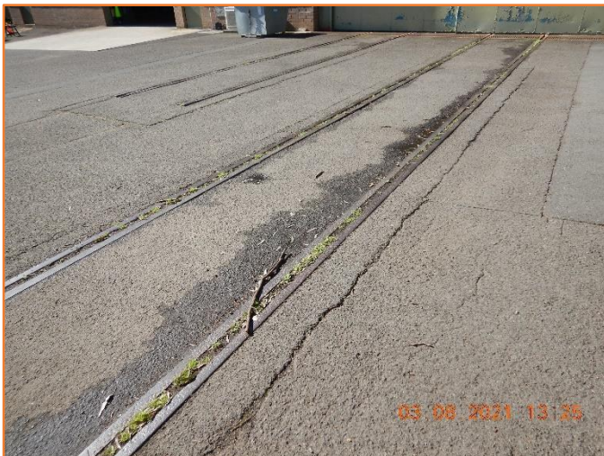
Figure 206: Poor - General condition of flexible pavement. Major cracking observed.
