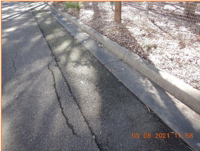
Figure 70: Reasonable - General condition of kerb and gutter and flexible pavement. Moderate cracking observed.
