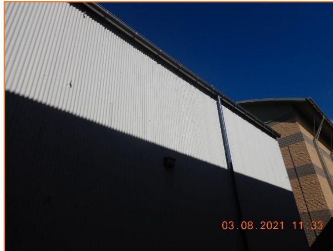
Figure 553: Reasonable - General condition of external clad wall.
