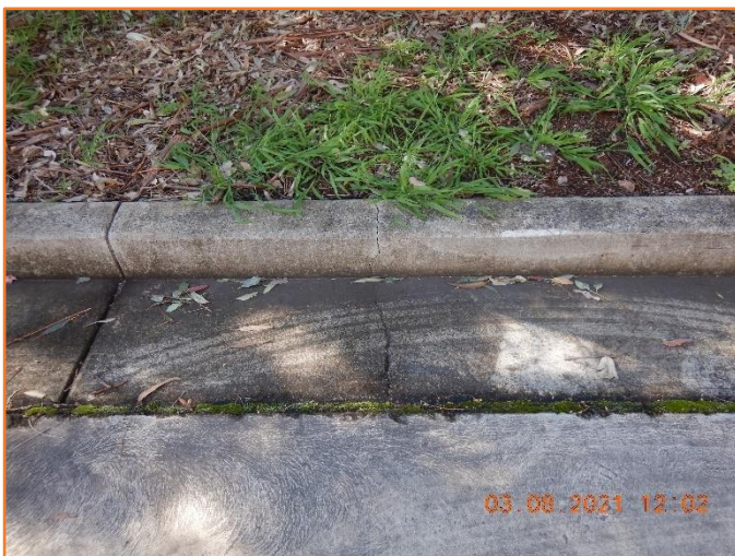
Figure 123: Reasonable - General condition of kerb and gutter. Moderate hairline cracking observed.
