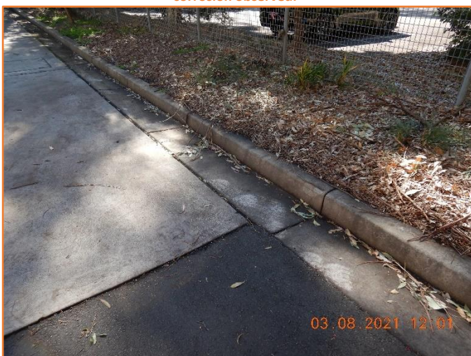
Figure 117: Reasonable - General condition of kerb and gutter.
