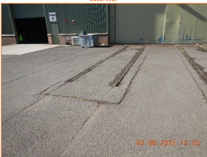
Figure 207: Poor - General condition of flexible pavement. Major cracking observed.
