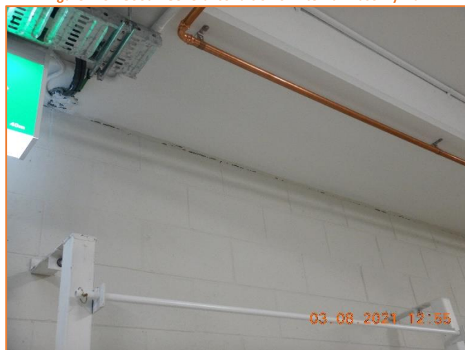
Figure 714: Reasonable - General condition of internal masonry wall. Minor hairline cracking observed.
