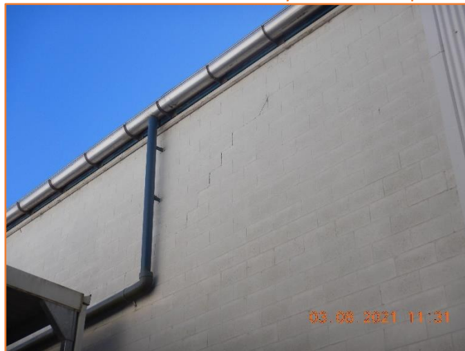
Figure 533: Poor - General condition of external masonry wall. Moderate step cracking observed.
