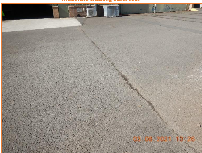
Figure 213: Reasonable - General condition of flexible pavement. Moderate cracking observed.
