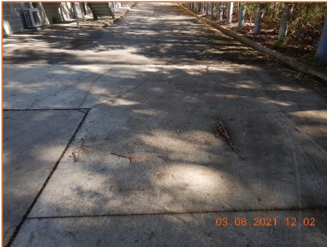
Figure 130: Reasonable - General condition of rigid pavement.
