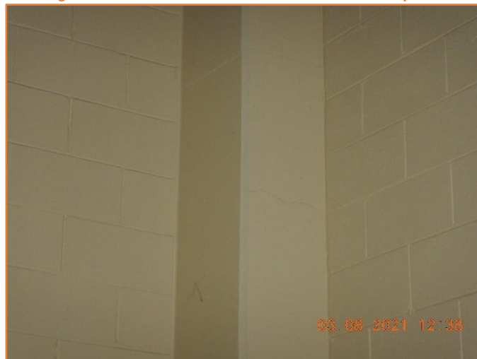
Figure 511: Reasonable - General condition of column. Minor hairline cracking observed.
