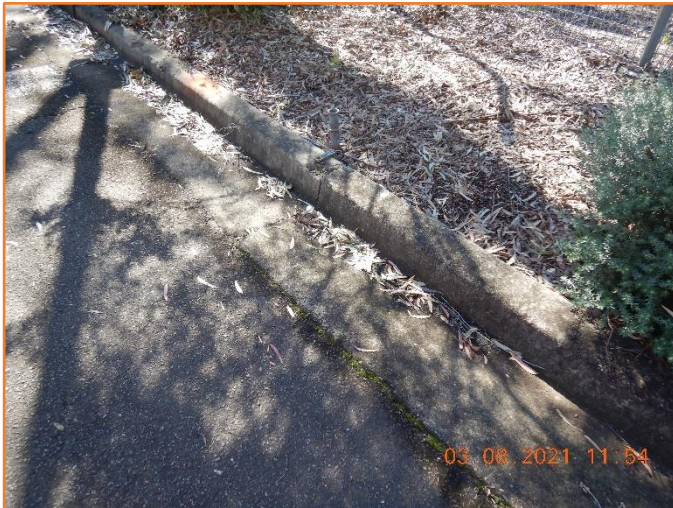
Figure 13: Reasonable - General condition of kerb and gutter.
