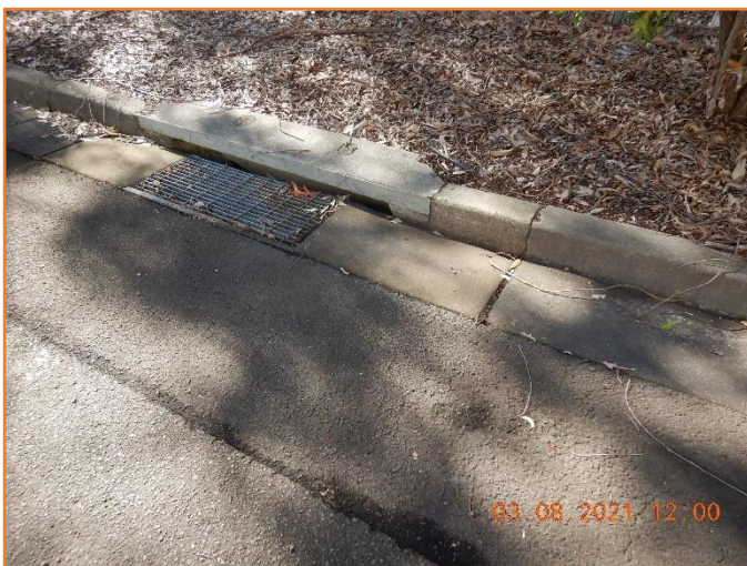
Figure 98: Reasonable - General condition of kerb and gutter and kerb inlet pit. Minor spalling observed.
