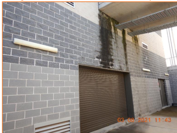
Figure 635: Reasonable - General condition of external masonry wall. Moderate water seepage observed.
