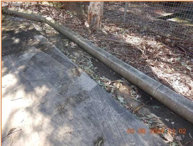
Figure 127: Reasonable - General condition of kerb and gutter.
