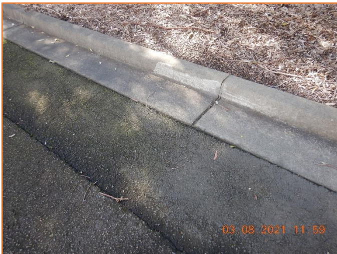
Figure 86: Reasonable - General condition of kerb and gutter.
