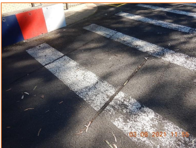
Figure 30: Reasonable - General condition of flexible pavement. Moderate physical damage observed.
