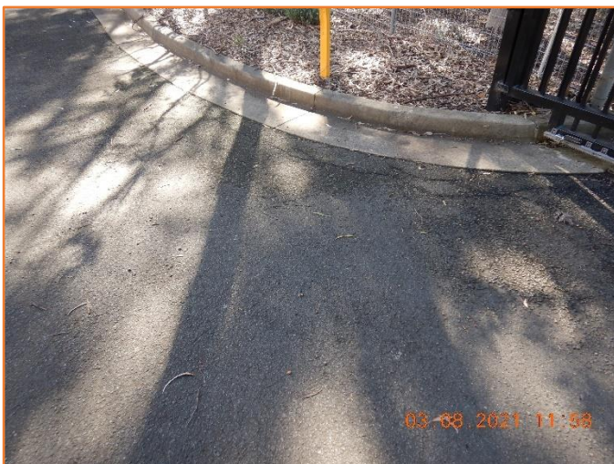
Figure 57: Reasonable - General condition of kerb and gutter and flexible pavement. Minor cracking observed.
