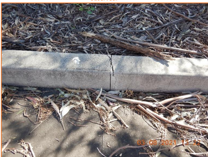
Figure 174: Reasonable - General condition of kerb. Minor hairline cracking observed.
