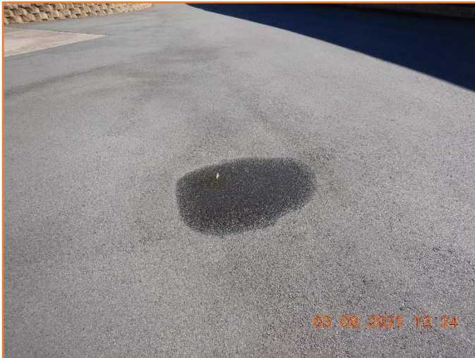
Figure 193: Reasonable - General condition of flexible pavement. Minor differential settlement observed.
