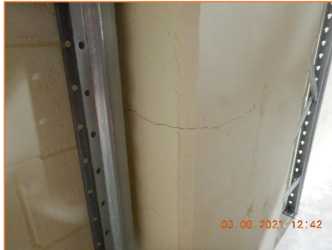
Figure 528: Reasonable - General condition of column. Moderate hairline cracking observed.
