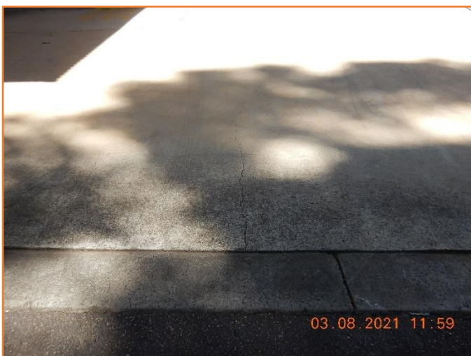
Figure 81: Reasonable - General condition of rigid pavement. Moderate hairline cracking observed.
