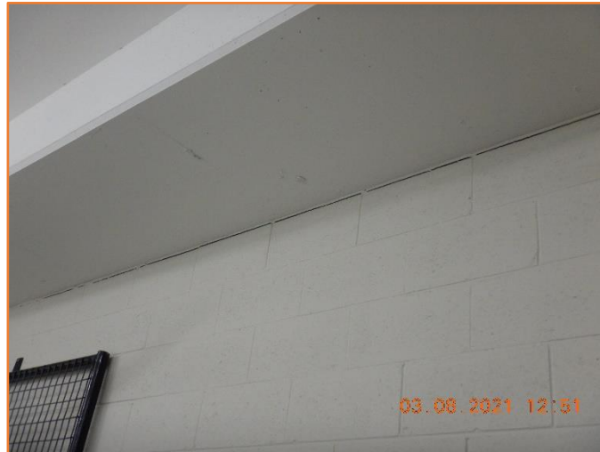
Figure 685: Reasonable - General condition of internal masonry wall. Minor hairline cracking observed.
