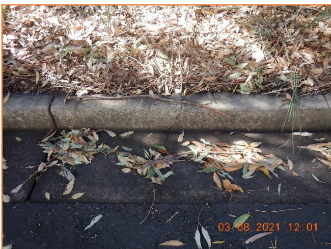
Figure 114: Reasonable - General condition of kerb and gutter. Moderate hairline cracking observed.
