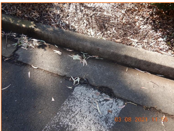
Figure 27: Reasonable - General condition of kerb and gutter. Minor spalling observed.
