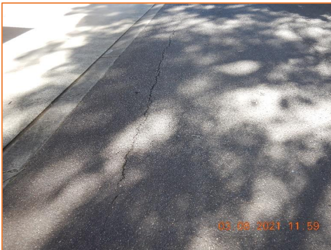
Figure 77: Reasonable - General condition of flexible pavement. Moderate cracking observed.
