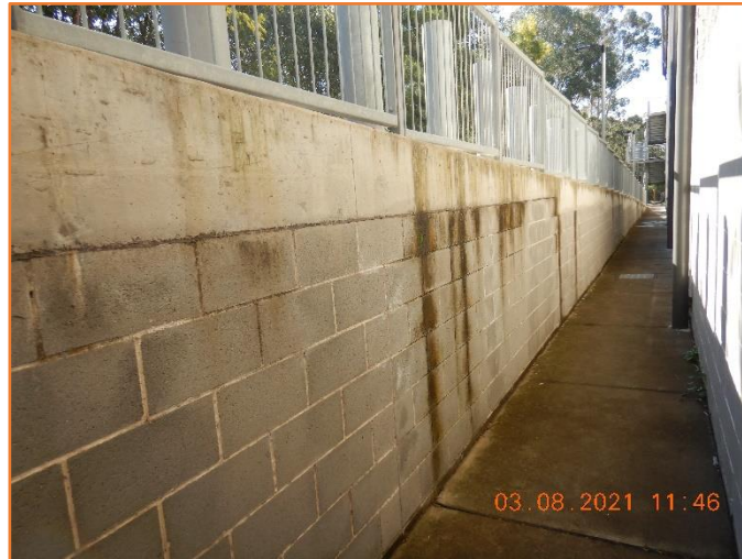
Figure 673: Reasonable - General condition of retaining wall. Moderate water seepage observed.
