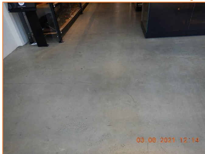
Figure 316: Reasonable - General condition of floor. Minor hairline cracking observed.
