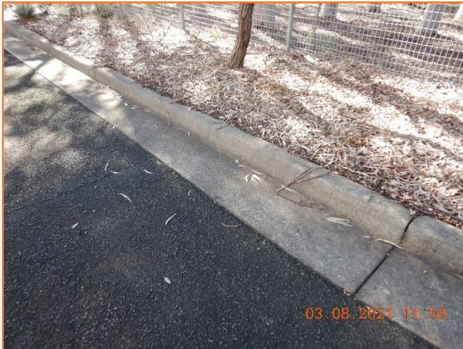
Figure 64: Reasonable - General condition of kerb and gutter.
