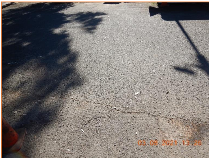
Figure 218: Reasonable - General condition of flexible pavement. Moderate cracking observed.
