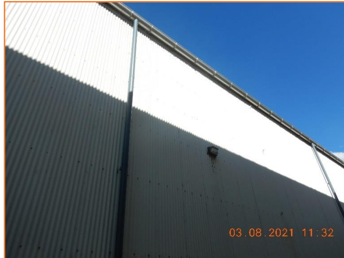
Figure 544: Reasonable - General condition of external clad wall. Minor corrosion observed.
