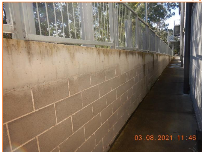
Figure 675: Reasonable - General condition of retaining wall. Moderate water seepage observed.
