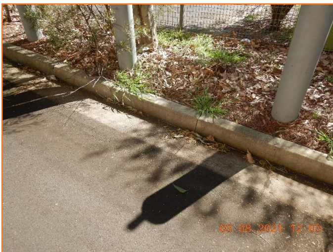
Figure 147: Reasonable - General condition of kerb and gutter.
