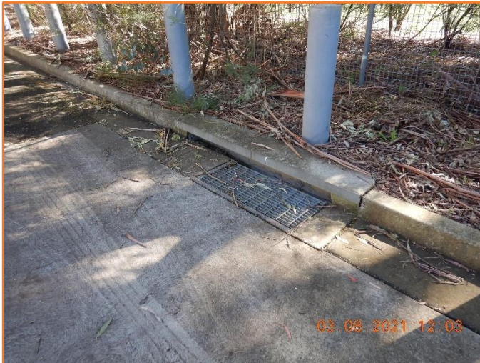
Figure 133: Reasonable - General condition of kerb inlet pit.
