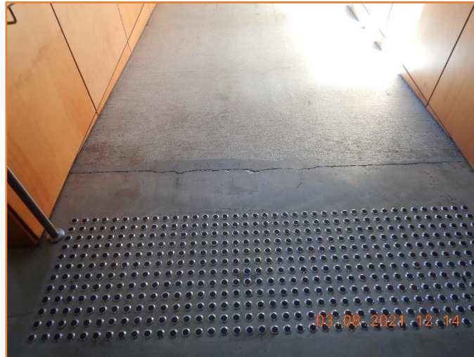
Figure 314: Reasonable - General condition of floor. Moderate hairline cracking observed.
