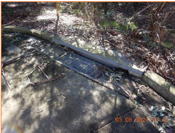
Figure 128: Reasonable - General condition of kerb inlet pit.
