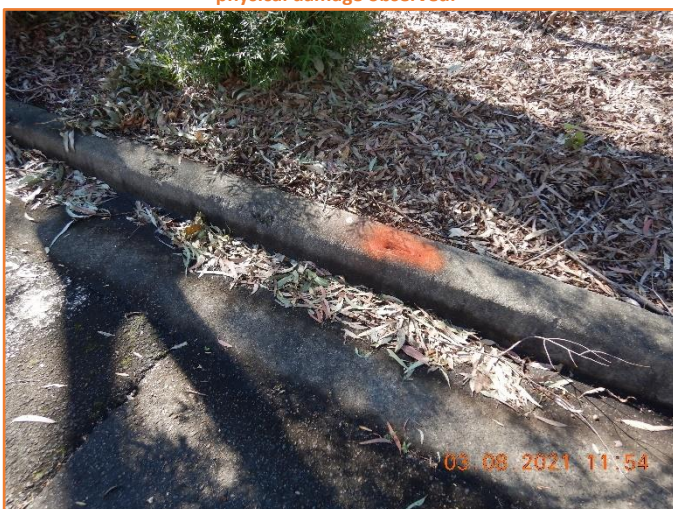
Figure 15: Reasonable - General condition of kerb and gutter.
