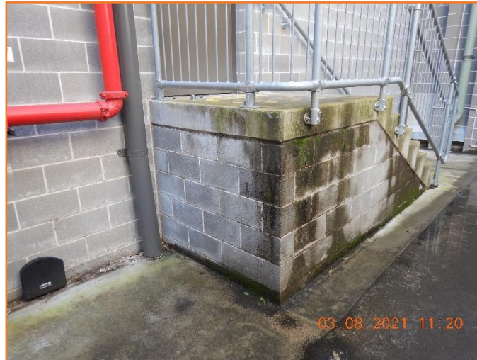
Figure 308: Reasonable - General condition of steps. Moderate water seepage and efflorescence observed.
