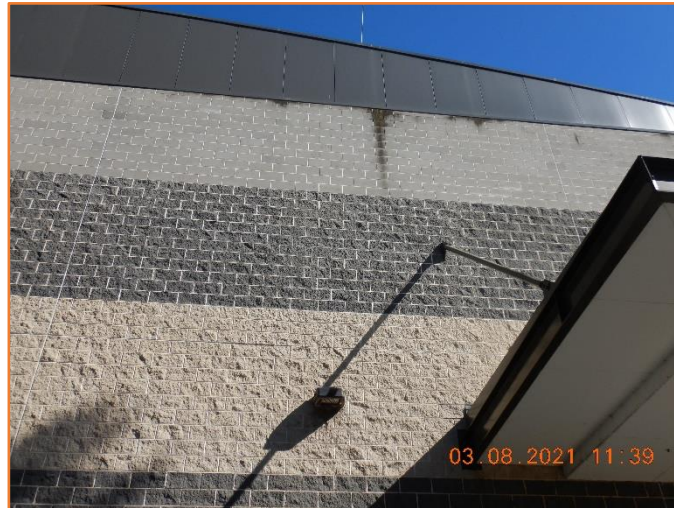
Figure 607: Reasonable - General condition of external masonry wall. Minor water seepage observed.
