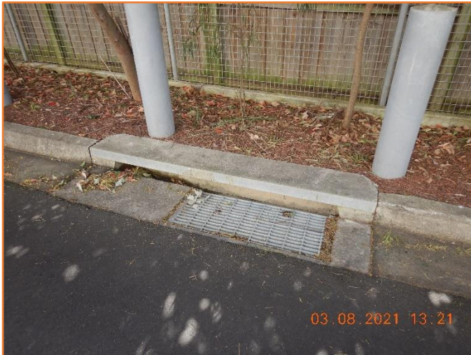
Figure 154: Good - General condition of kerb inlet pit.
