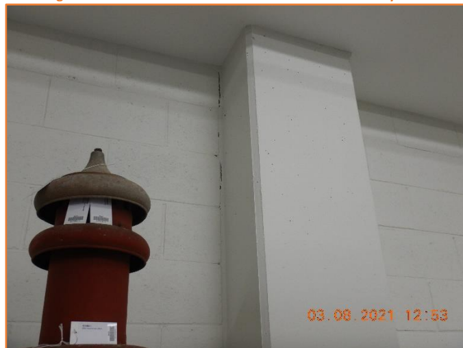
Figure 701: Reasonable - General condition of internal masonry wall. Moderate hairline cracking observed.
