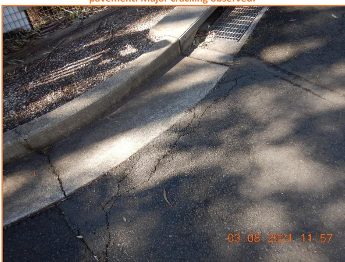
Figure 54: Poor - General condition of kerb and gutter and flexible pavement. Major cracking observed.
