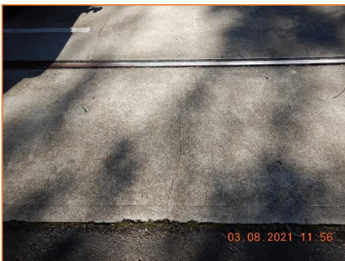
Figure 39: Reasonable - General condition of rigid pavement. Moderate hairline cracking observed.
