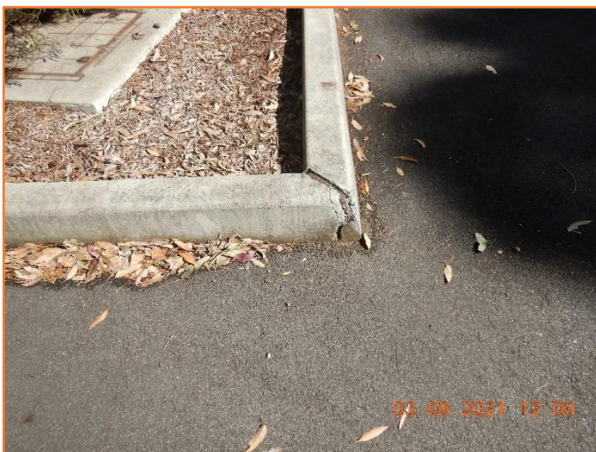
Figure 104: Reasonable - General condition of kerb. Minor cracking observed.
