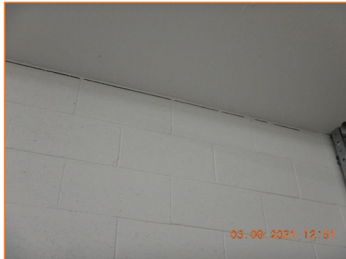
Figure 686: Reasonable - General condition of internal masonry wall. Minor hairline cracking observed.
