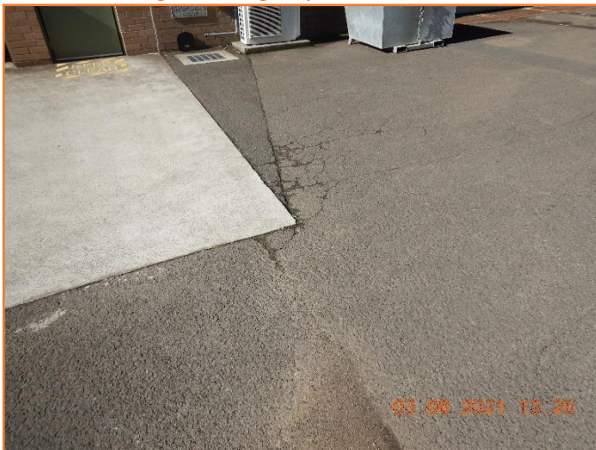
Figure 215: Reasonable - General condition of flexible pavement. Moderate alligator cracking observed.
