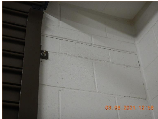
Figure 737: Poor - General condition of external rendered wall. Moderate cracking observed.
