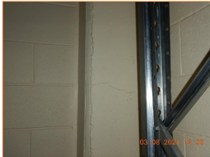
Figure 499: Reasonable - General condition of column. Minor hairline cracking observed.
