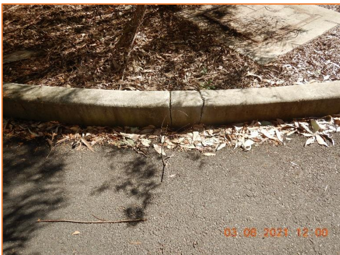
Figure 102: Reasonable - General condition of kerb. Moderate cracking observed.
