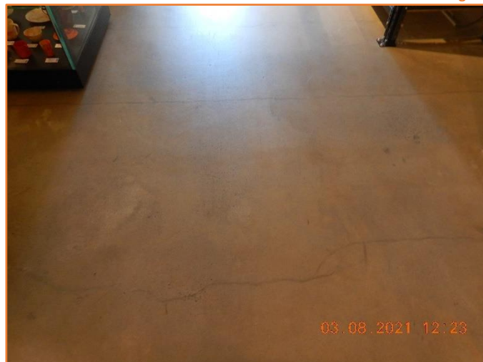
Figure 396: Reasonable - General condition of floor. Moderate hairline cracking observed.
