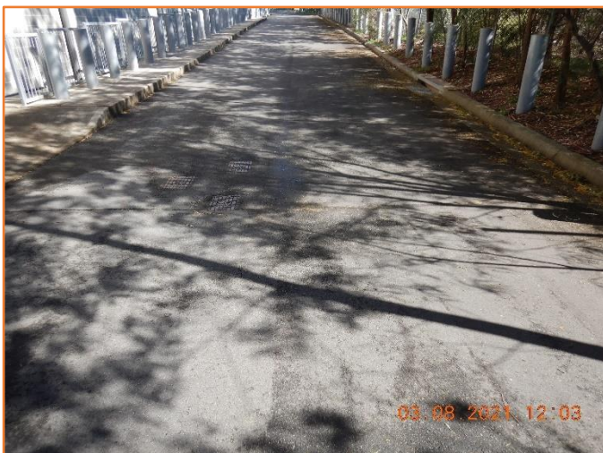
Figure 138: Reasonable - General condition of flexible pavement.
