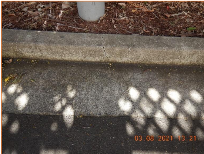
Figure 160: Reasonable - General condition of kerb and gutter. Moderate hairline cracking observed.
