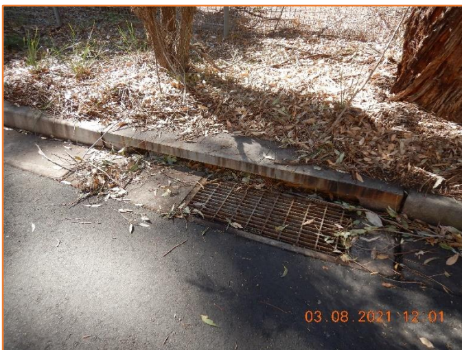
Figure 116: Reasonable - General condition of kerb inlet pit. Minor corrosion observed.
