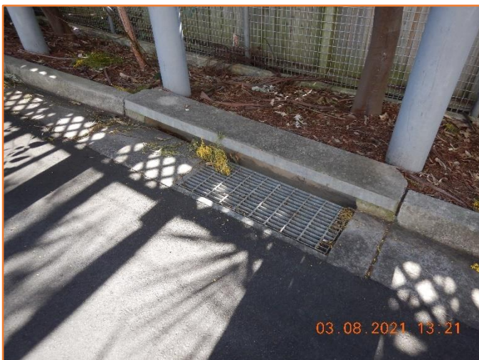
Figure 165: Good - General condition of kerb inlet pit.
