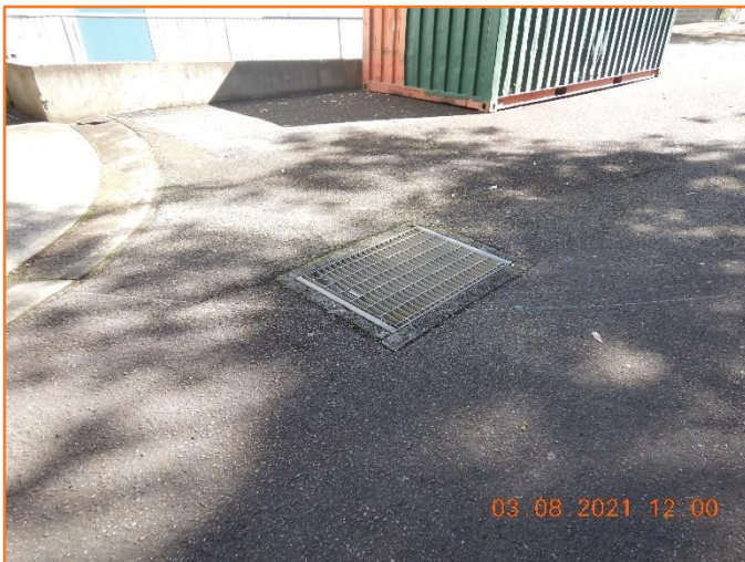
Figure 89: Reasonable - General condition of grated inlet pit.
