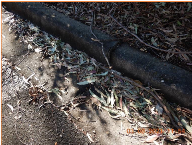
Figure 17: Reasonable - General condition of kerb and gutter. Moderate differential settlement observed.
