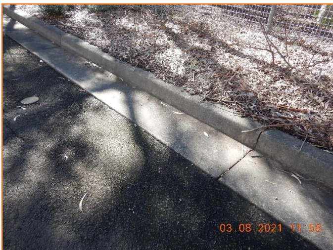
Figure 66: Reasonable - General condition of kerb and gutter.
