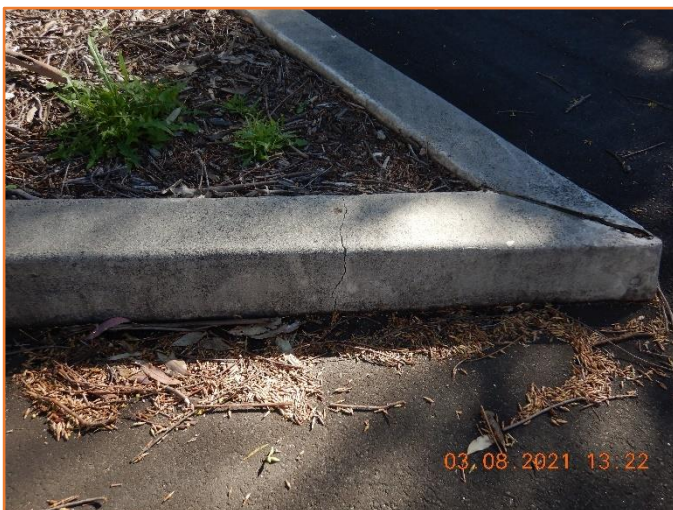
Figure 173: Reasonable - General condition of kerb. Minor hairline cracking observed.
