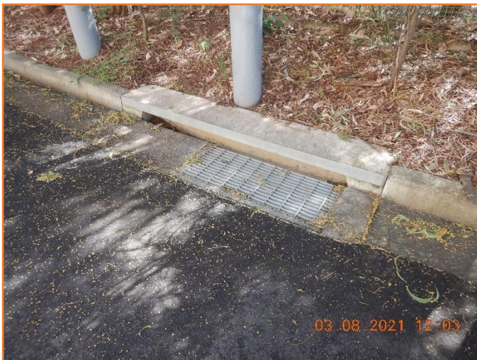
Figure 143: Good - General condition of kerb inlet pit.
