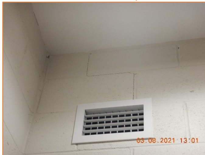
Figure 750: Reasonable - General condition of internal masonry wall. Minor step cracking observed.
