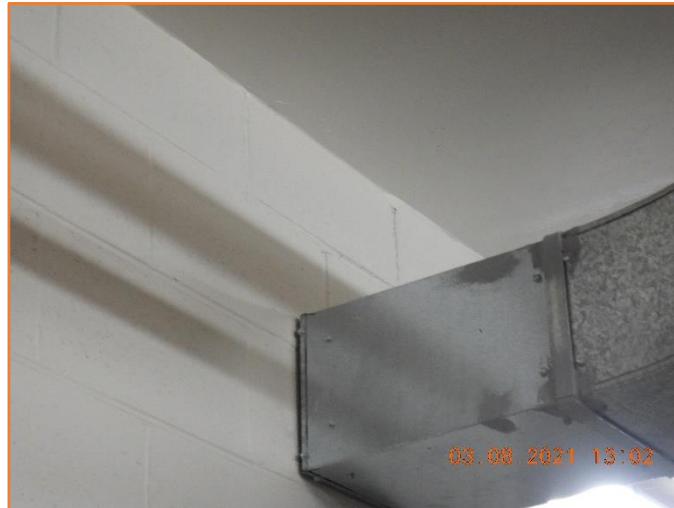
Figure 754: Reasonable - General condition of internal masonry wall. Minor step cracking observed.
