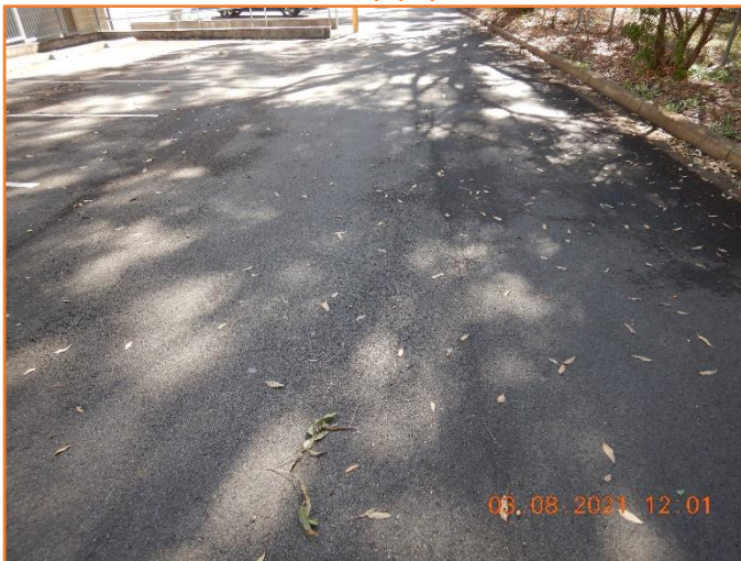
Figure 107: Reasonable - General condition of flexible pavement. Reasonable - General condition of kerb and gutter. Minor hairline cracking observed.
