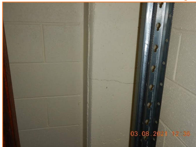
Figure 500: Reasonable - General condition of column. Minor hairline cracking observed.
