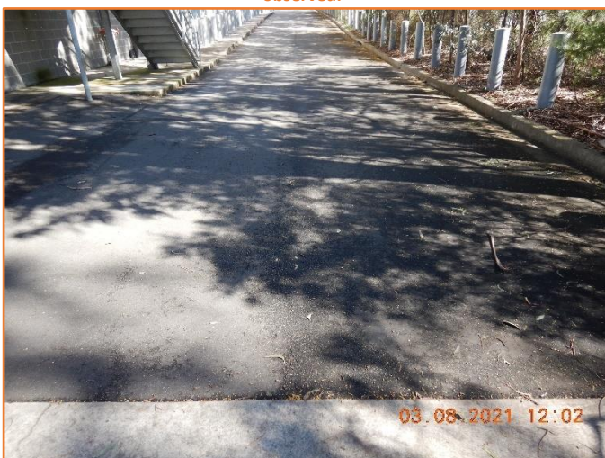
Figure 132: Reasonable - General condition of flexible pavement.
