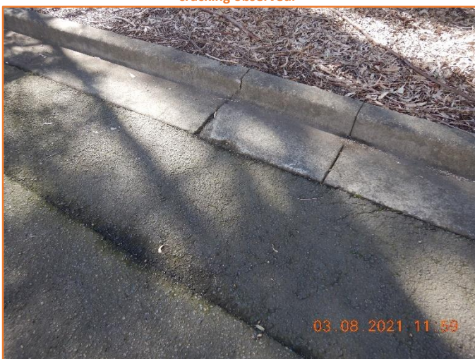
Figure 78: Reasonable - General condition of kerb and gutter. Moderate spalling and loss of material observed.
