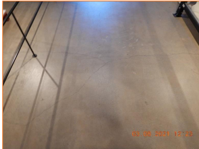
Figure 395: Reasonable - General condition of floor. Moderate hairline cracking observed.
