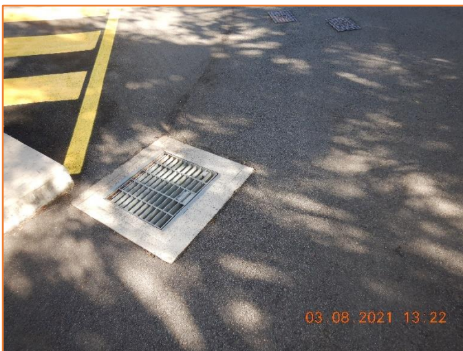
Figure 167: Reasonable - General condition of flexible pavement and grated inlet pit. Moderate cracking observed.
