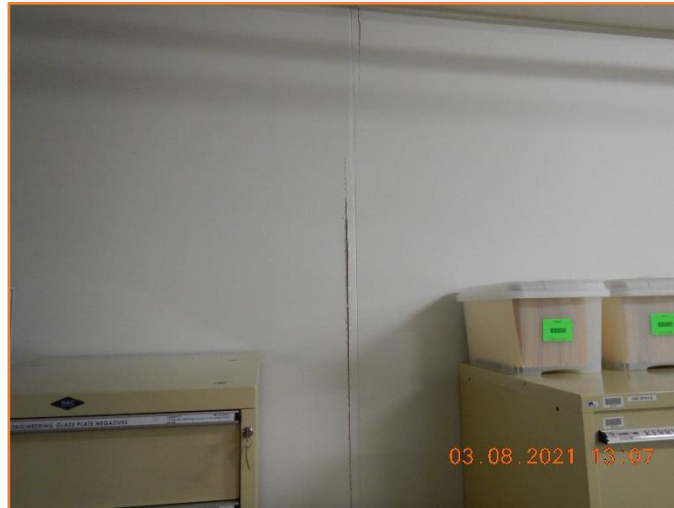
Figure 784: Reasonable - General condition of internal wall. Moderate hairline cracking observed.
