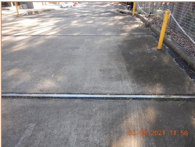
Figure 41: Reasonable - General condition of rigid pavement.
