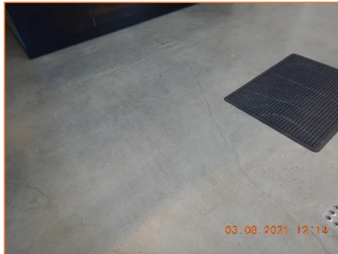
Figure 315: Reasonable - General condition of floor. Minor hairline cracking observed.
