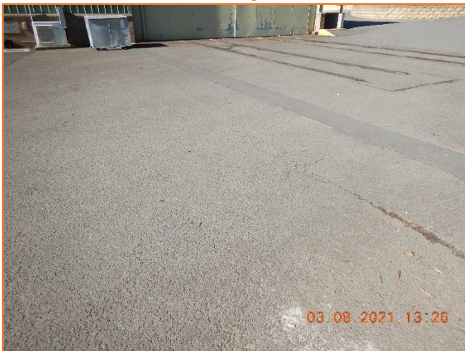
Figure 212: Reasonable - General condition of flexible pavement. Moderate cracking observed.
