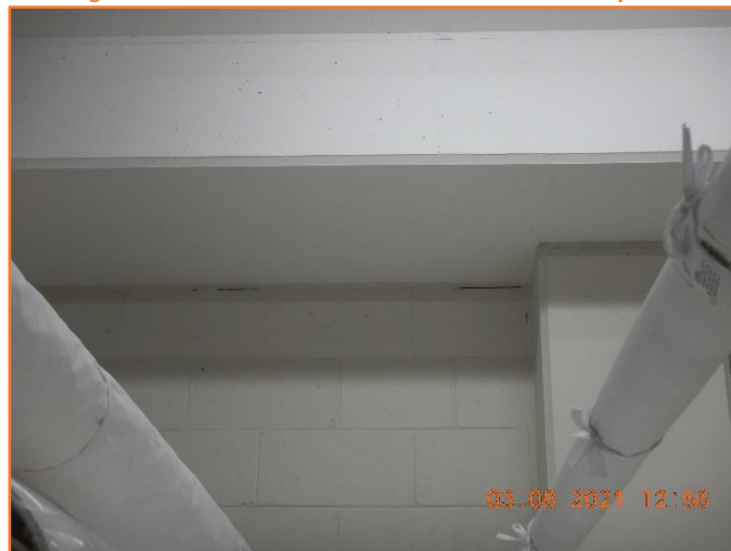
Figure 719: Reasonable - General condition of internal masonry wall. Minor hairline cracking observed.
