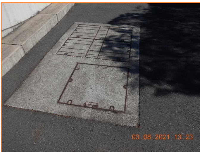
Figure 183: Reasonable - General condition of service pits.
