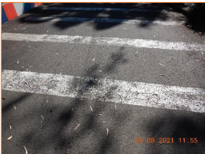
Figure 21: Reasonable - General condition of flexible pavement. Moderate cracking observed.
