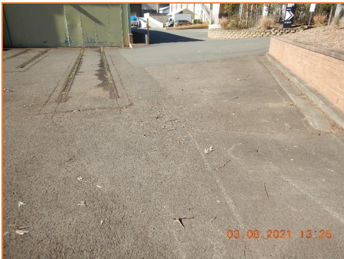
Figure 209: Reasonable - General condition of flexible pavement. Moderate cracking observed.
