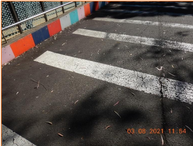
Figure 10: Reasonable - General condition of flexible pavement. Moderate cracking observed.
