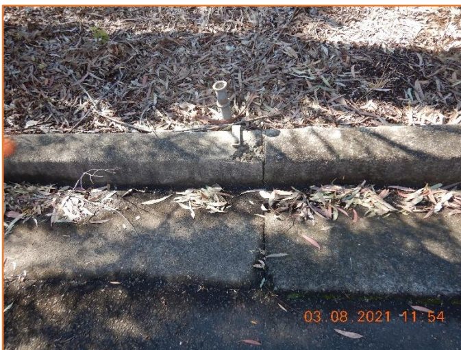
Figure 14: Reasonable - General condition of kerb and gutter. Minor physical damage observed.
