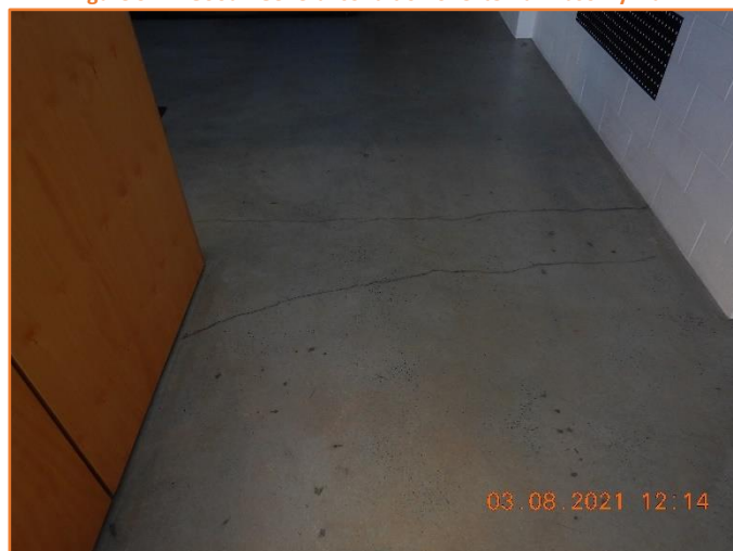
Figure 313: Reasonable - General condition of floor. Moderate hairline cracking observed.
