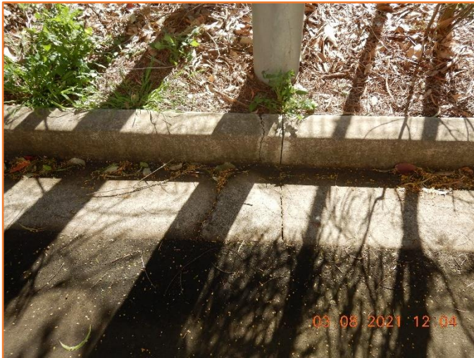
Figure 148: Reasonable - General condition of kerb and gutter. Moderate cracking observed.
