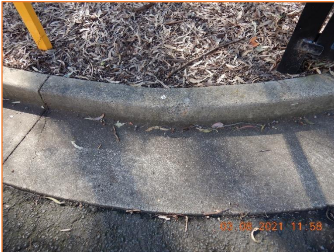
Figure 58: Reasonable - General condition of kerb and gutter. Minor spalling observed.
