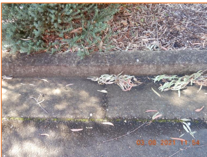
Figure 12: Reasonable - General condition of kerb and gutter. Minor hairline cracking observed.
