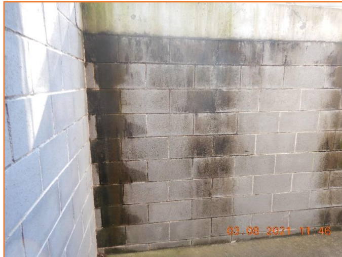
Figure 670: Reasonable - General condition of retaining wall. Moderate water seepage observed.
