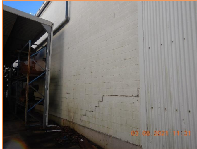
Figure 532: Poor - General condition of external masonry wall. Moderate step cracking observed.
