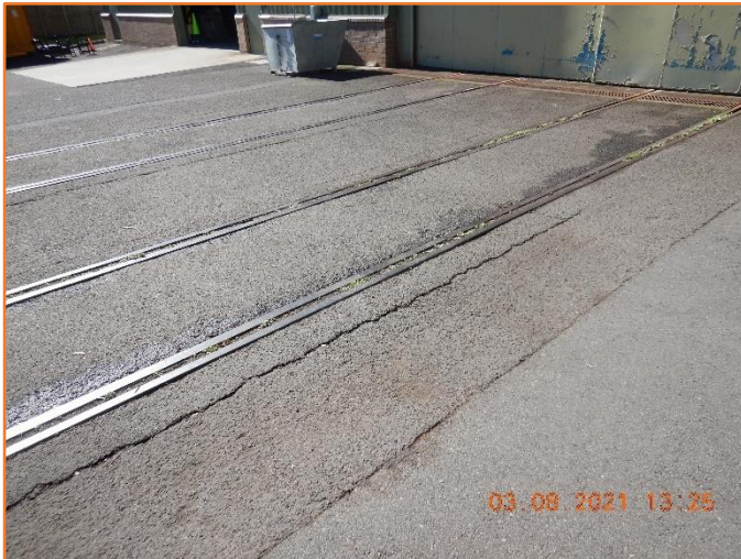
Figure 205: Poor - General condition of flexible pavement. Major cracking observed.
