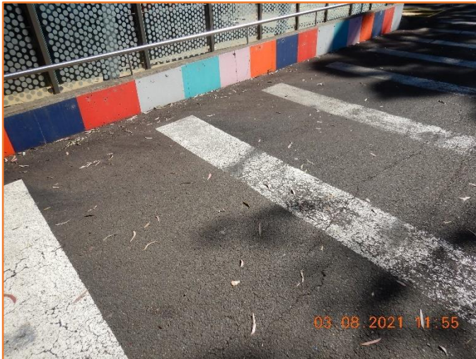
Figure 22: Reasonable - General condition of flexible pavement. Moderate cracking observed.
