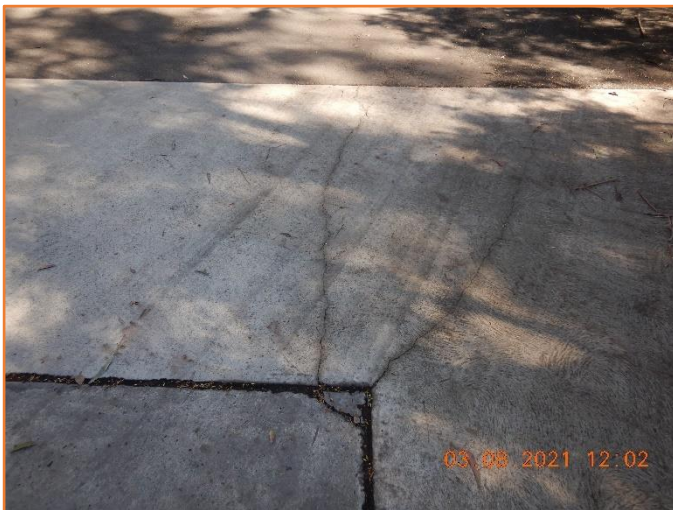
Figure 131: Poor - General condition of rigid pavement. Moderate cracking observed.
