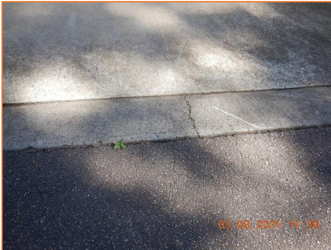
Figure 82: Reasonable - General condition of gutter. Minor cracking observed.
