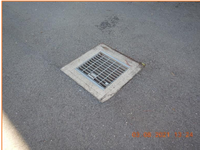
Figure 199: grated inlet pit.
