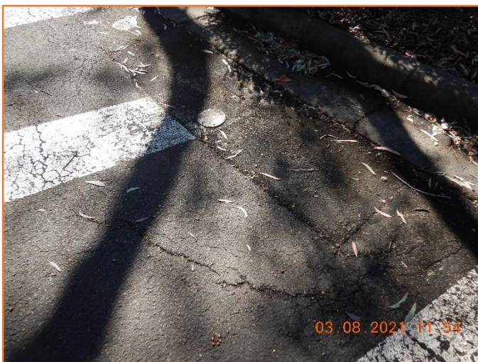
Figure 8: Poor - General condition of flexible pavement. Moderate cracking and vertical displacement observed.
