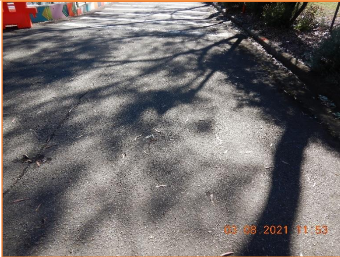
Figure 1: Reasonable - General condition of flexible pavement. Moderate cracking observed.
