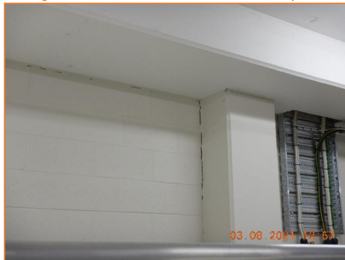
Figure 728: Reasonable - General condition of internal masonry wall. Moderate hairline cracking observed.
