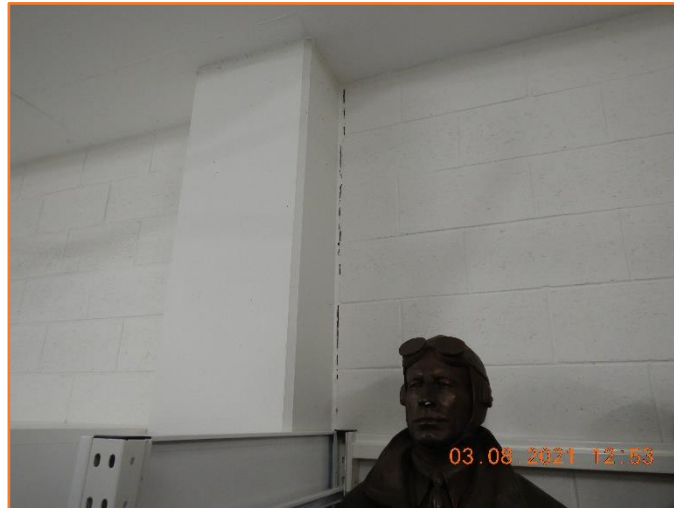
Figure 697: Reasonable - General condition of internal masonry wall. Moderate hairline cracking observed.
