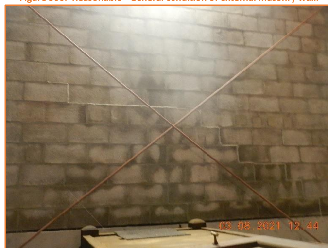
Figure 567: Poor - General condition of internal masonry wall. Moderate step cracking observed.
