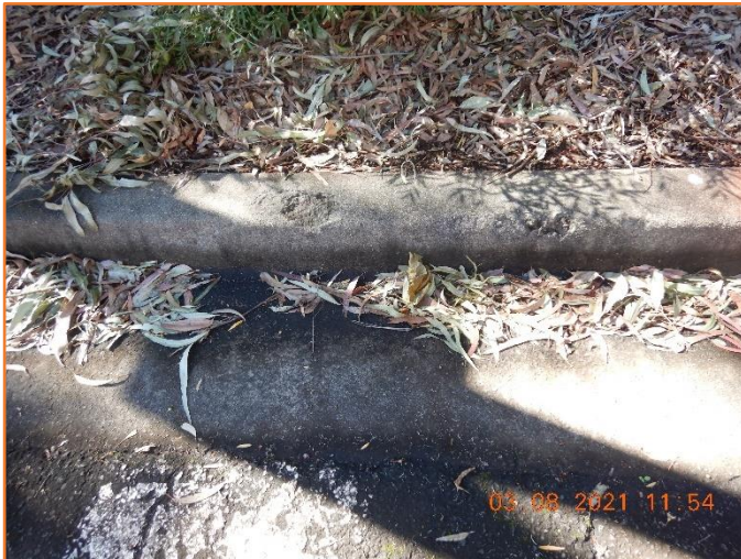
Figure 16: Reasonable - General condition of kerb and gutter. Minor spalling observed.
