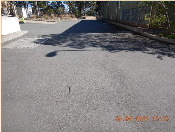
Figure 181: Reasonable - General condition of flexible pavement. Minor physical damage observed.
