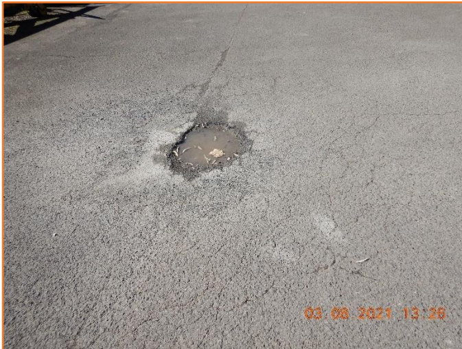
Figure 214: Defective - General condition of flexible pavement. Major alligator cracking and pot holes observed.
