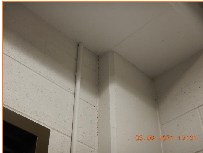
Figure 749: Reasonable - General condition of internal masonry wall. Minor hairline cracking observed.
