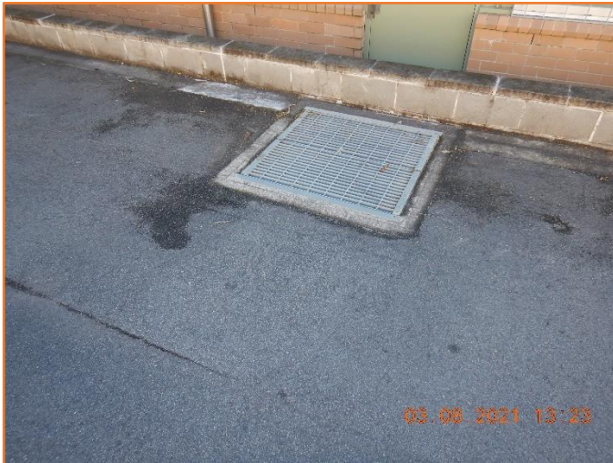
Figure 190: Good - General condition of grated inlet pit.
