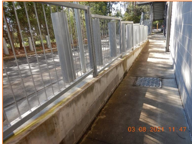
Figure 679: Good - General condition of retaining wall.
