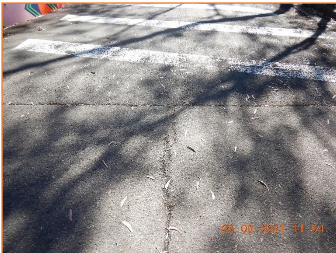
Figure 5: Reasonable - General condition of flexible pavement. Moderate cracking observed.
