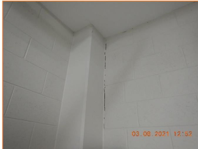
Figure 694: Reasonable - General condition of internal masonry wall. Moderate hairline cracking observed.
