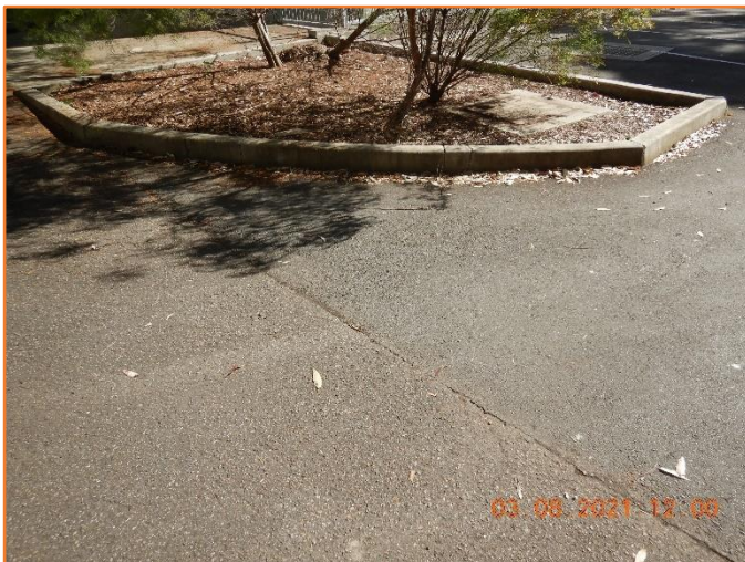
Figure 101: Reasonable - General condition of kerb and flexible pavement.
