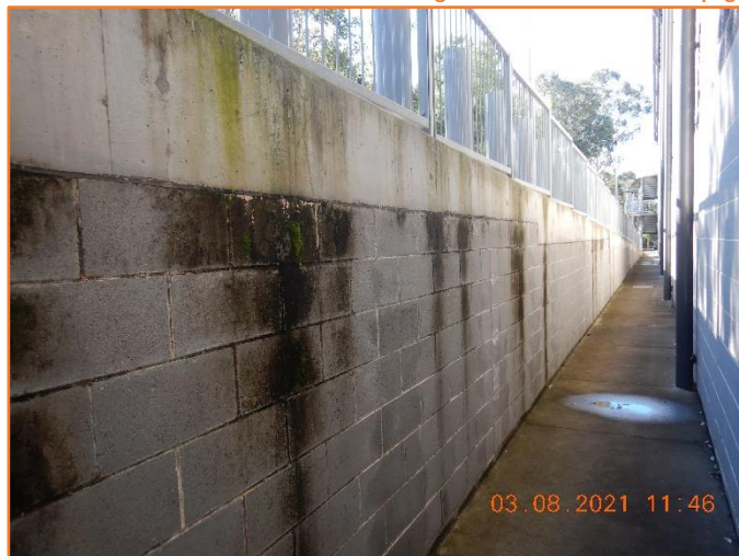
Figure 671: Reasonable - General condition of retaining wall. Moderate water seepage observed.
