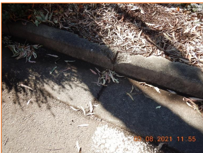
Figure 24: Reasonable - General condition of kerb and gutter. Moderate spalling observed.
