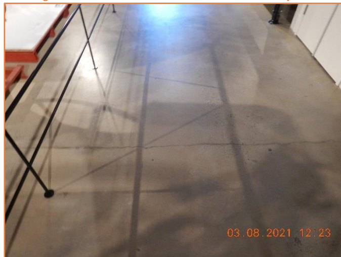
Figure 393: Reasonable - General condition of floor. Moderate hairline cracking observed.
