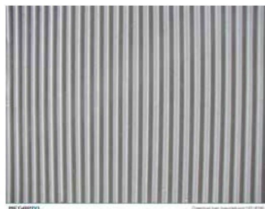
CORRUGATED PRECAST CONCRETE WITH COLOUR OXIDE COATING TO THE BUILDING BASE
